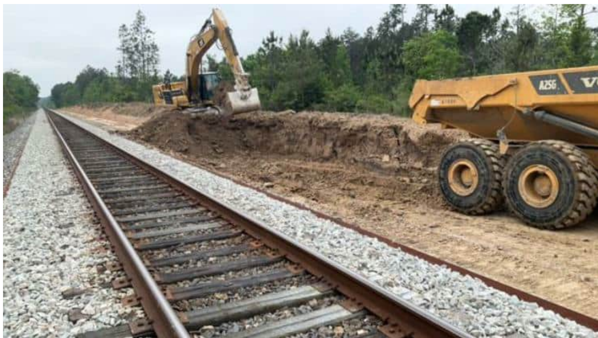
Figure 11. Cut and move overburden for fill, south of private road crossing; Facing Southwest. (N. Bartosch 04/20/24)
