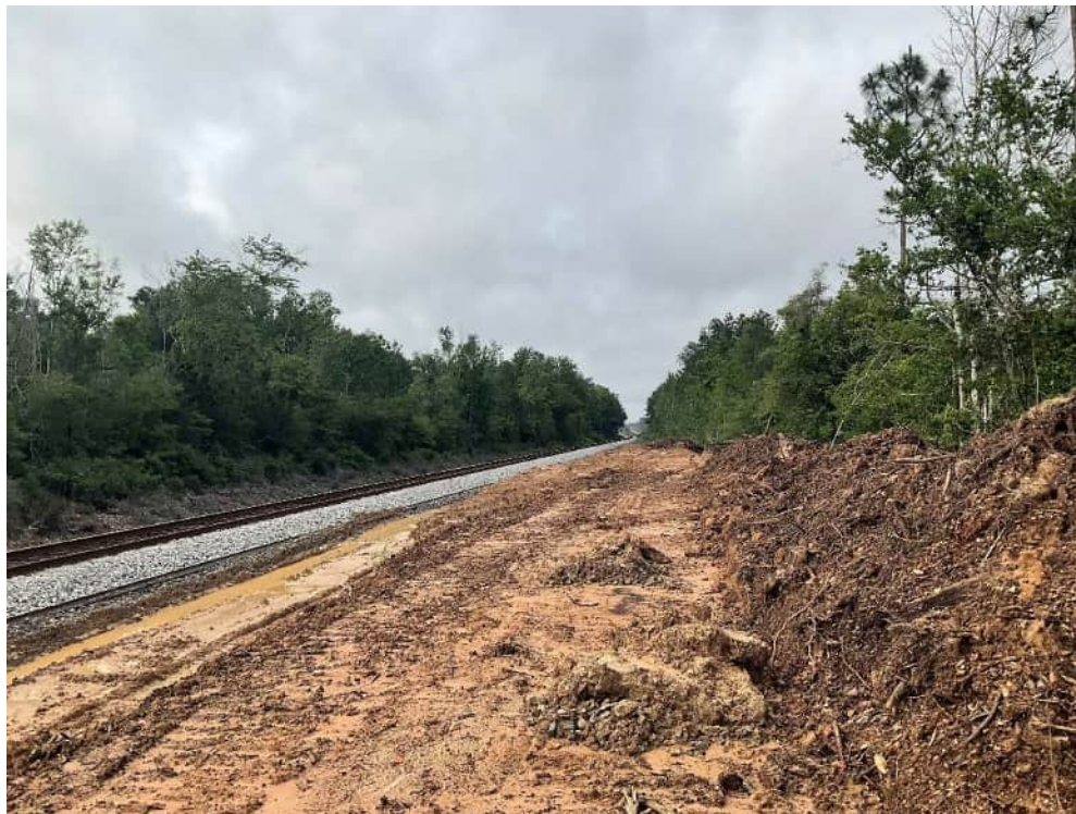
Figure 18. Southern extreme of project area, new disturbance complete; facing South. (N. Bartosch 05/06/24)
