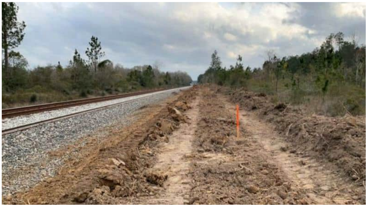
Figure 5. Initial cut of overburden south of the private road crossing, nearing southern extreme of project; facing south. (N. Bartosch 02/27/24)
