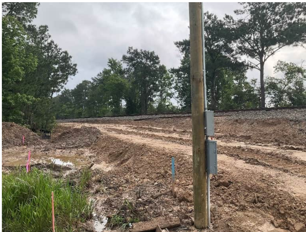
Figure 14. South Singer Switch Cabin project location, new disturbance complete; facing Northeast. (N. Bartosch 05/06/24)
