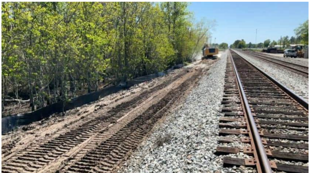
Figure 8. An example of lime mixing for soil stabilization, North section of project; facing South. (N. Bartosch 03/26/24)
