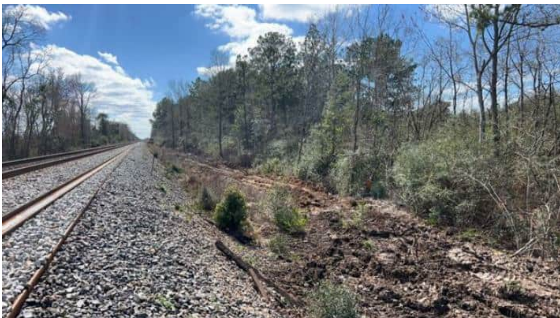
Figure 2. Initial topsoil clearing near South Singer Switch Cabin; facing south. (N. Bartosch 02/21/24)
