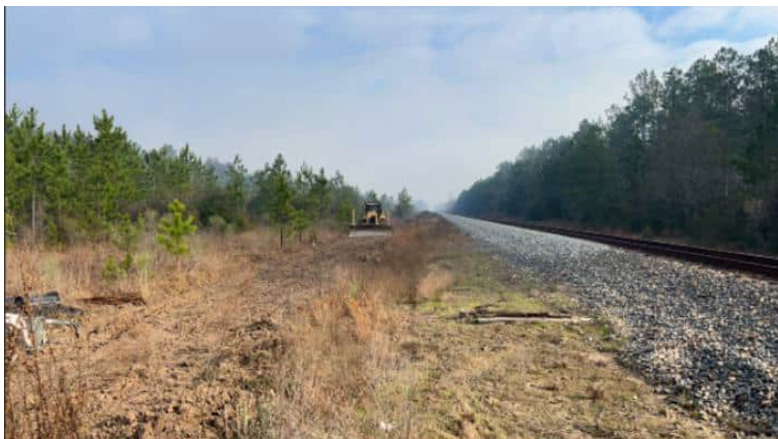
Figure 4. Initial topsoil clearing near private road crossing, south portion of project; facing North. (N. Bartosch 02/21/24)
