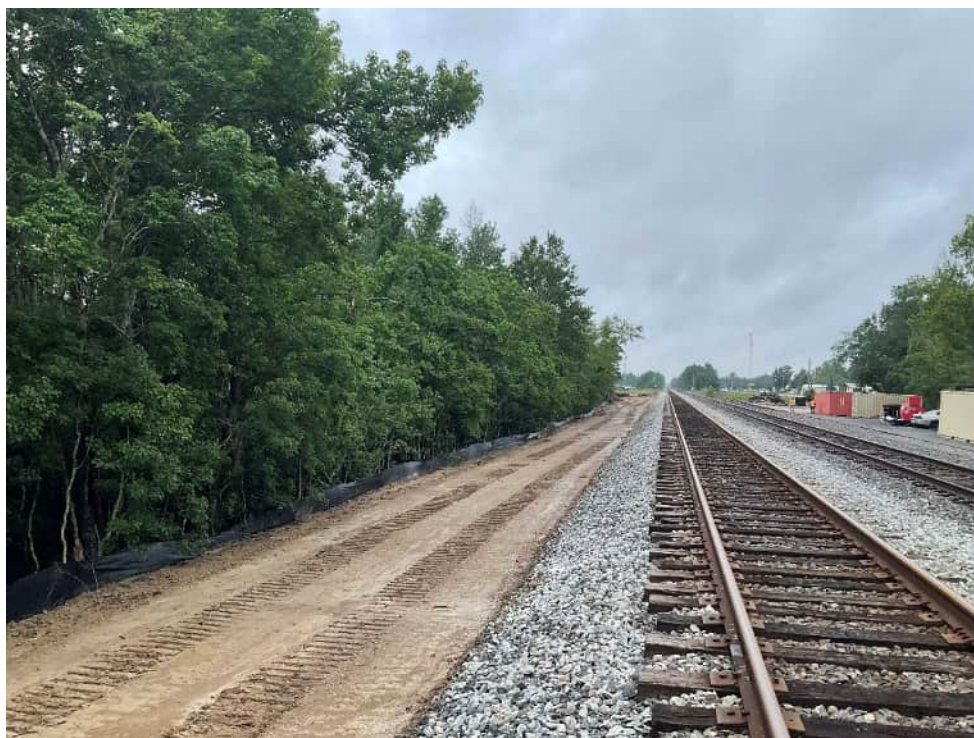
Figure 12. North Singer project section, new disturbance complete; facing South. (N. Bartosch 05/06/24)
