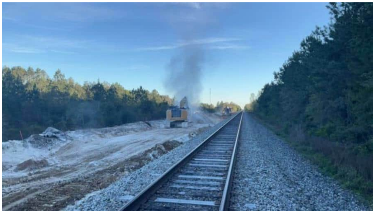
Figure 7. An example of lime mixing for soil stabilization, near private road crossing; facing North. (N. Bartosch 03/19/24)
