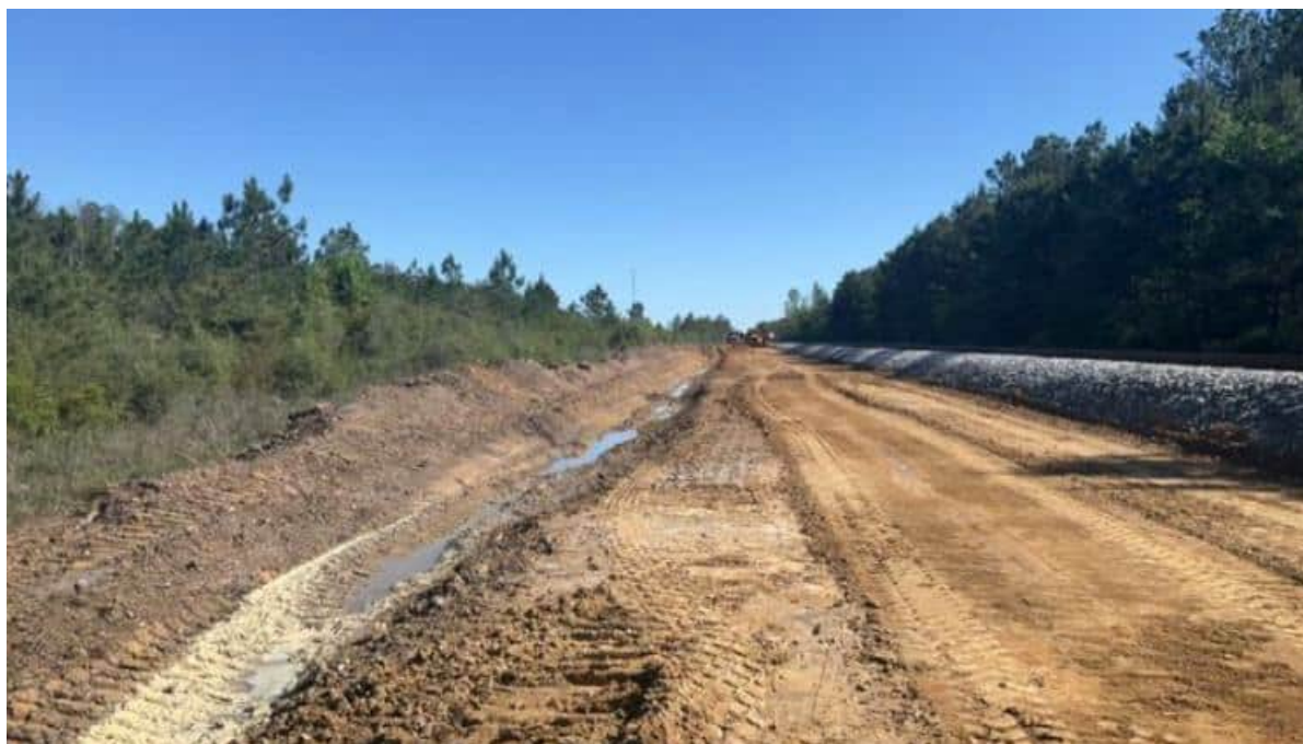
Figure 9. Drainage ditch construction progress example between South Singer Switch Cabin and private road crossing; facing North. (N. Bartosch 04/03/24)
