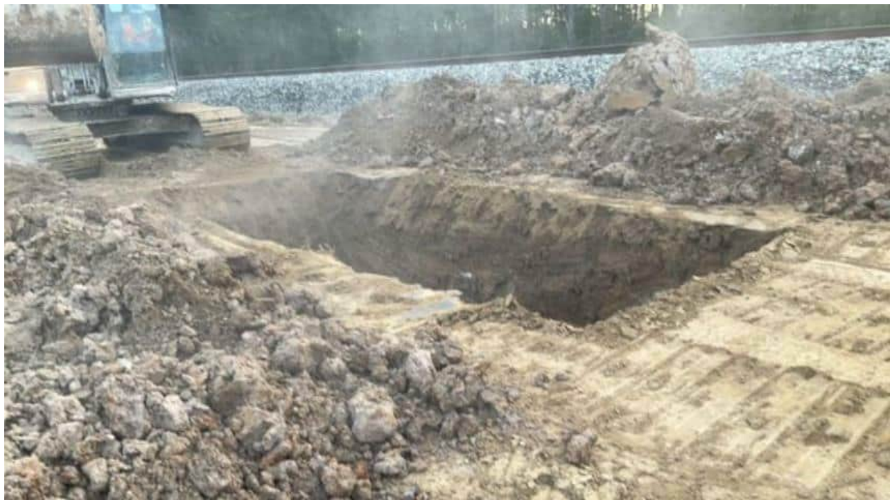
Figure 6. An example of lime mixing pit for soil stabilization; facing Northeast. (N. Bartosch 03/13/24)
