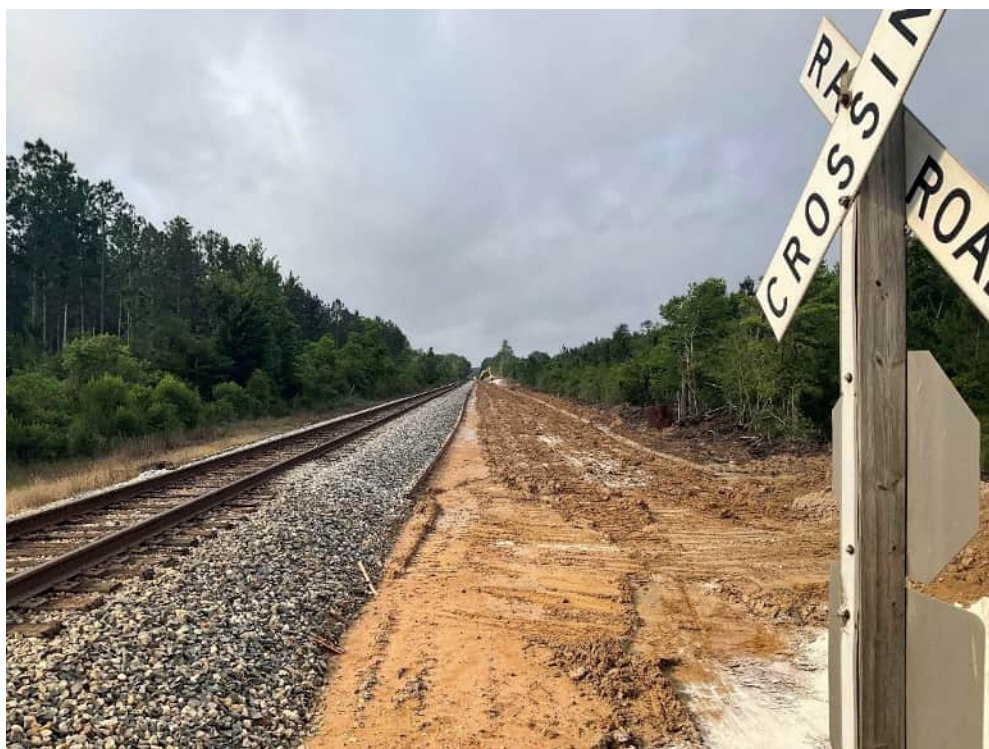
Figure 17. Private Road Crossing project area, new disturbance complete; facing South. (N. Bartosch 05/06/24)
