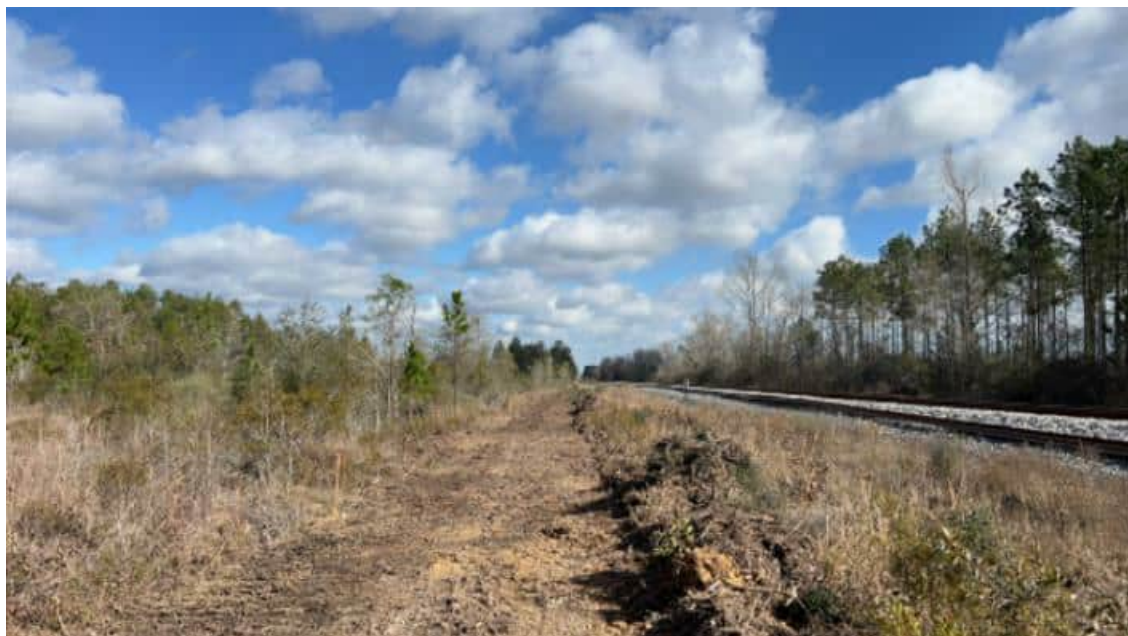
Figure 3. Initial topsoil clearing between South Singer Switch Cabin and private road crossing; facing North. (N. Bartosch 02/21/24)
