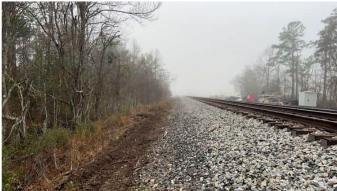
Figure 1. Initial topsoil clearing for access road to North Singer Switch Cabin; facing south. (N. Bartosch 02/21/24)
