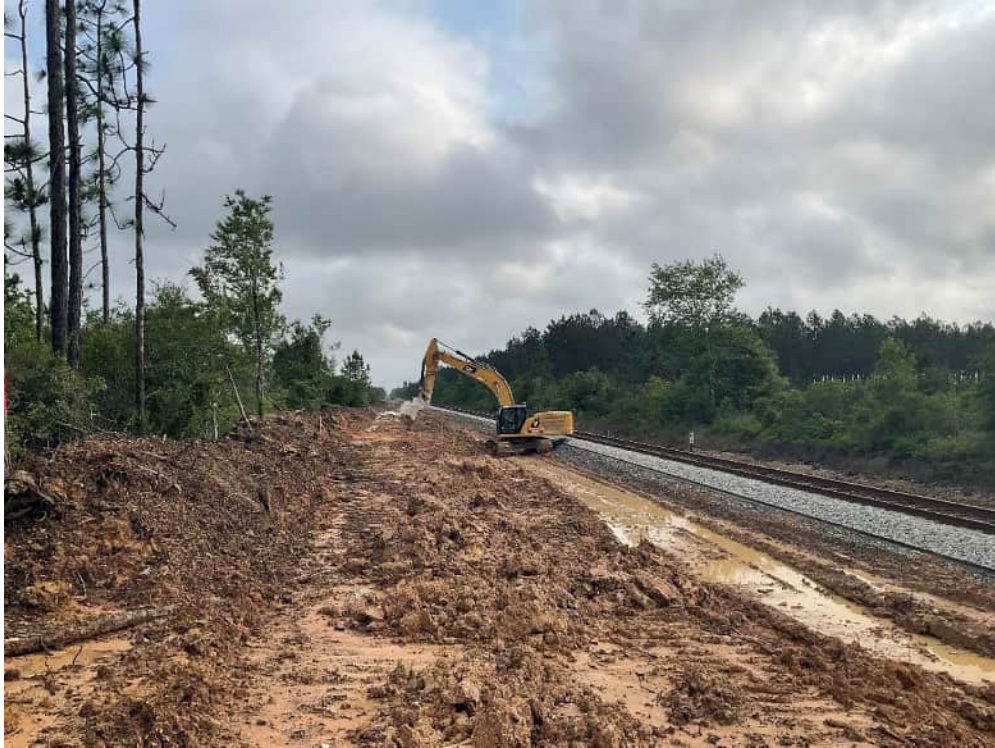
Figure 19. Southern extreme of project area, new disturbance complete; facing North. (N. Bartosch 05/06/24)
