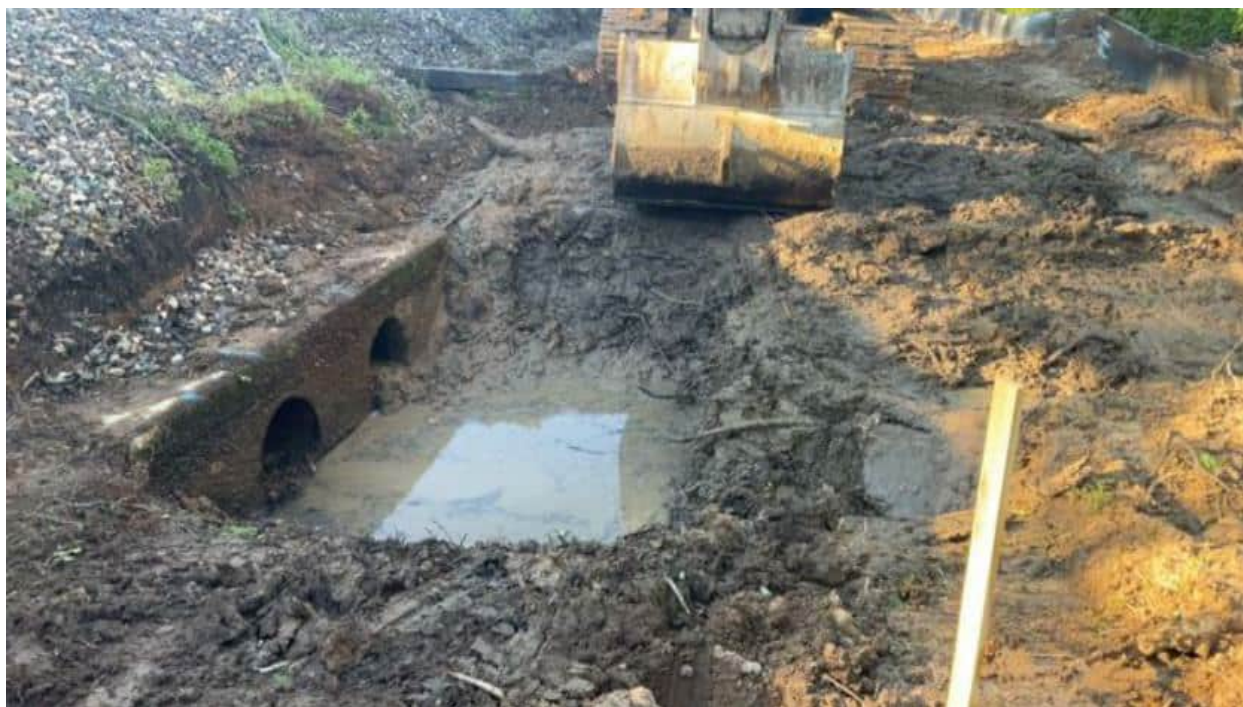
Figure 10. Jack and Bore pipe installation excavation preparation example, near South Singer Switch Cabin; facing South. (N. Bartosch 04/04/24)
