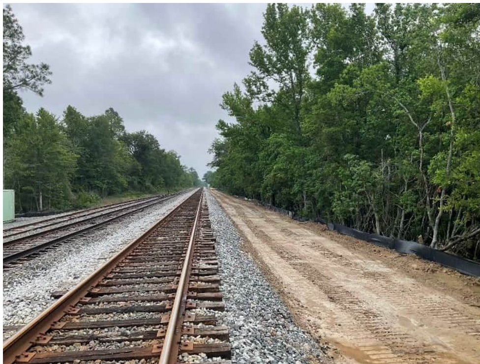
Figure 13. North Singer project section, new disturbance complete; facing North. (N. Bartosch 05/06/24)
