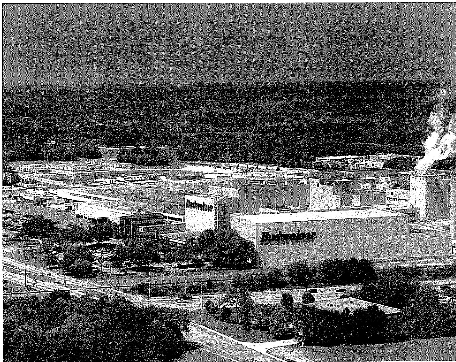
The Anheuser-Busch brewery at 111 Busch Drive in North Jacksonville.
