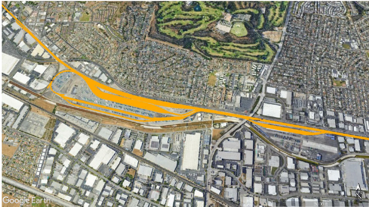
Figure No. 5 Google Earth Image of UP City of Industry Intermodal Terminal
