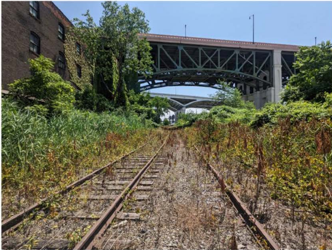
BJB 74.00-0 , Carnegie Avenue Overhead Bridge. Reverse Track View, from high milepost facing low milepost
