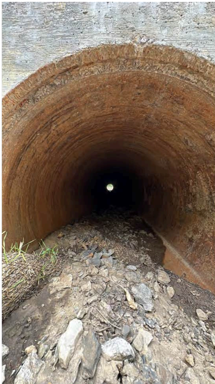
Picture 1: View of 36'x 67'' culvert south of Bailey Road at WQS point number 2.
