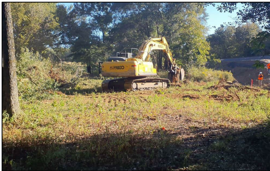
Figure 12. Tree felling to assist with inserting culvert pipe extension; view facing northeast. (Photograph by T. Himebaugh 10/9/23.)
