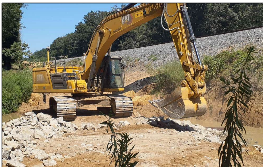
Figure 6. Excavator spreading gravel near bridge; view facing east. (Photograph by T. Himebaugh 9/1/23.)
