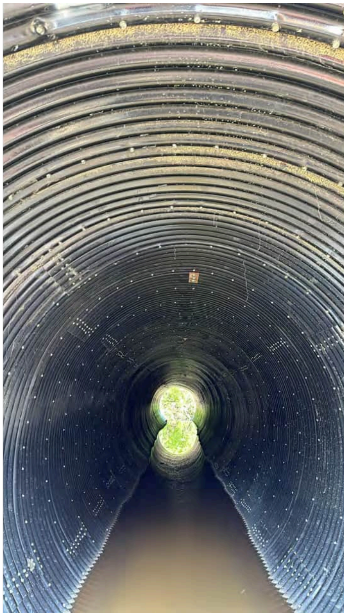
Picture 1: View of 96'x 86'' culvert north of Bailey Road at WQS point number 1.
