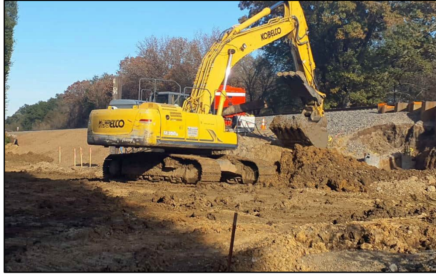
Figure 15. Excavator cleaning out mud near drill locations; view facing northeast. (Photograph by T. Himebaugh 11/13/23.)
