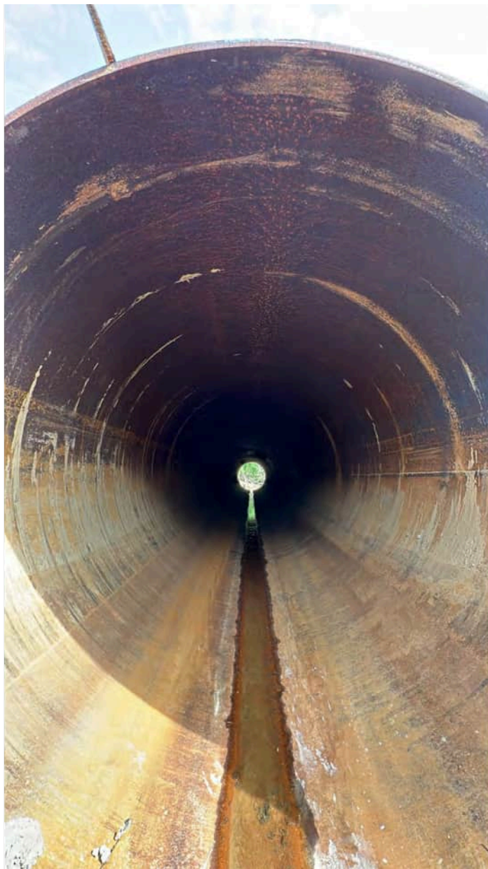
Picture 3: View of 84' by 86'' culvert north of Bailey Road at WQS point number 1.
