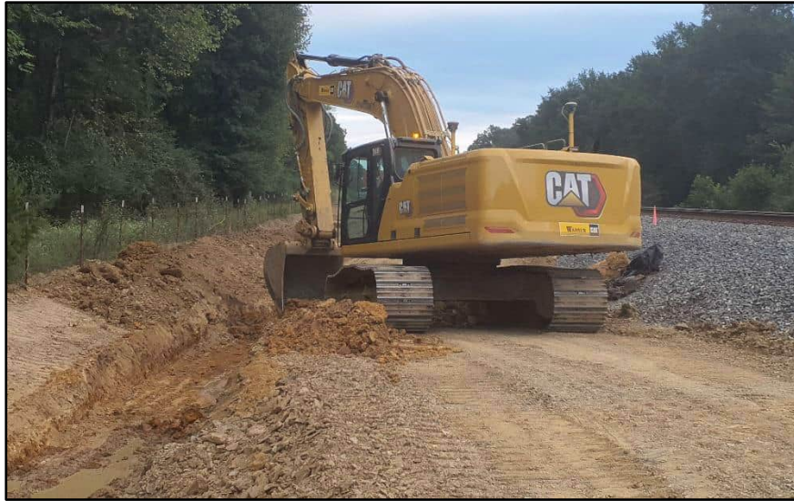
Figure 11. Excavator clearing area for culvert installation; view facing northeast. (Photograph by T. Himebaugh 10/4/23.)
