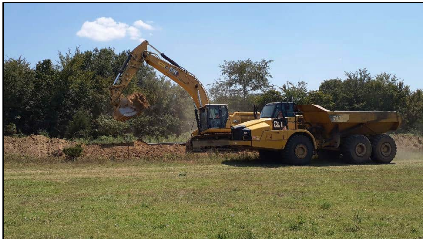
Figure 4. Removal of backfill via excavator and dump truck; view facing south. (Photograph by T. Himebaugh 8/29/23.)
