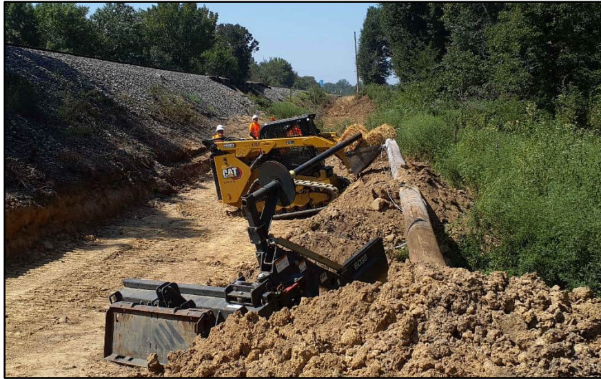
Figure 3. Preparing area for silt fence installation, hay bales used as ballast; view facing southwest. (Photograph by T. Himebaugh 8/25/23.)
