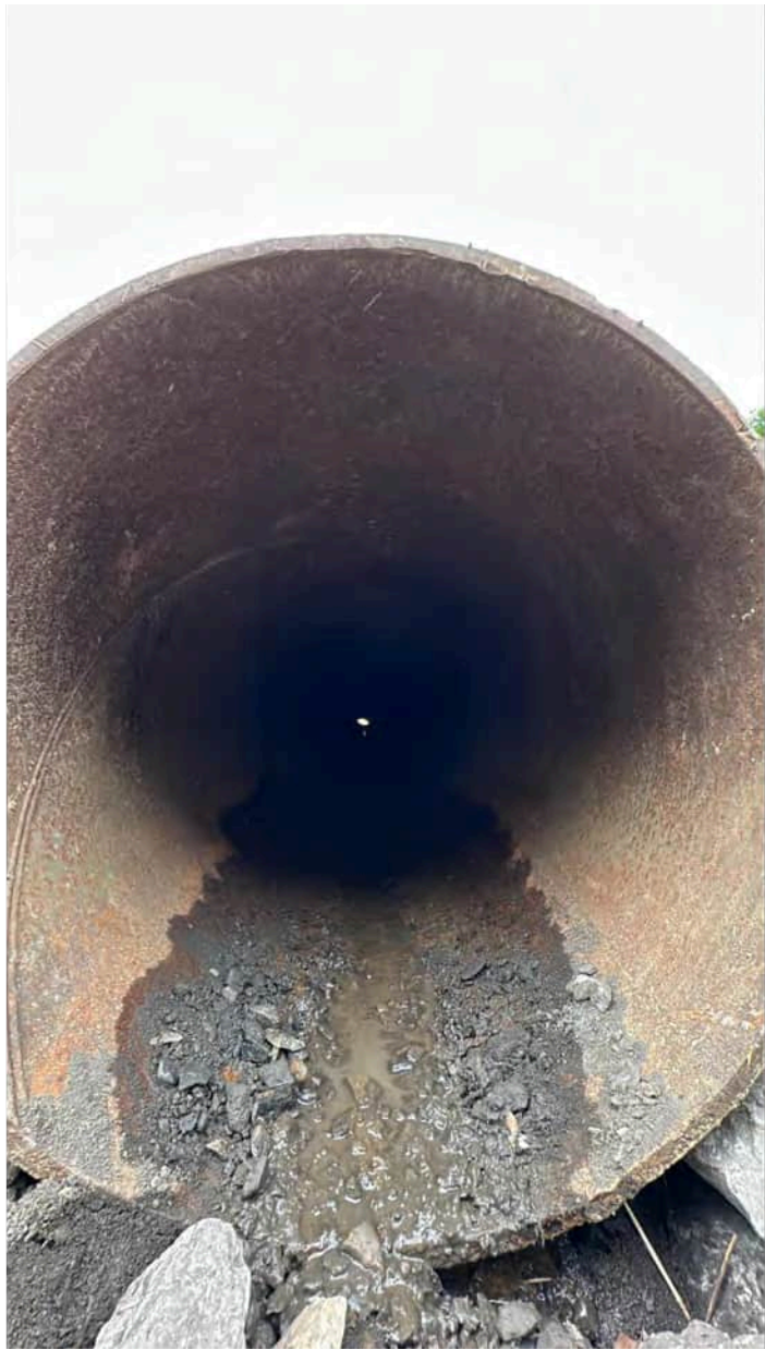
Picture 2: View of 36'x 67'' culvert south of Bailey Road at WQS point number 2.
