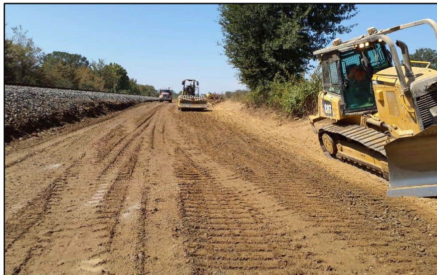
Figure 8. Cut and fill grading using fill from the borrow pit; view facing southwest. (Photograph by R. Campbell 9/6/23.)
