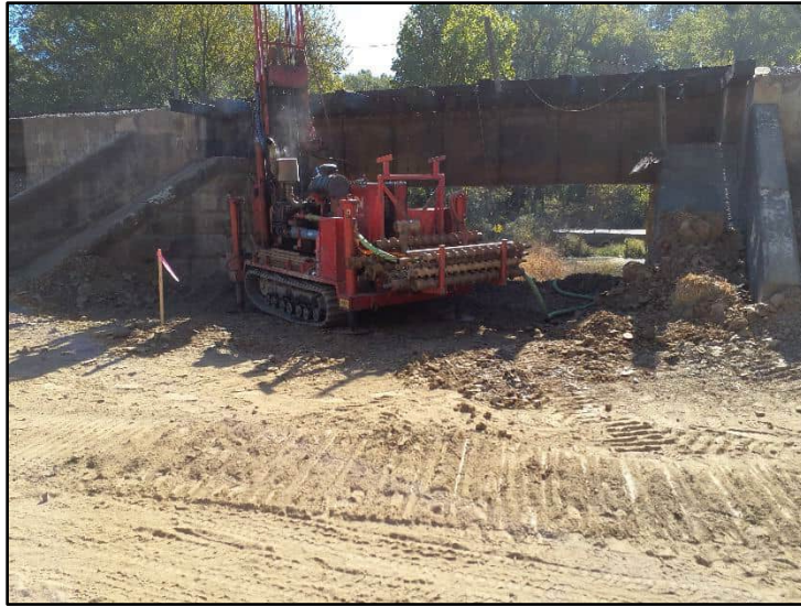
Figure 13. Drilling for core samples near bridge to be replaced; view facing southeast. (Photograph by R. Cline 10/17/23.)
