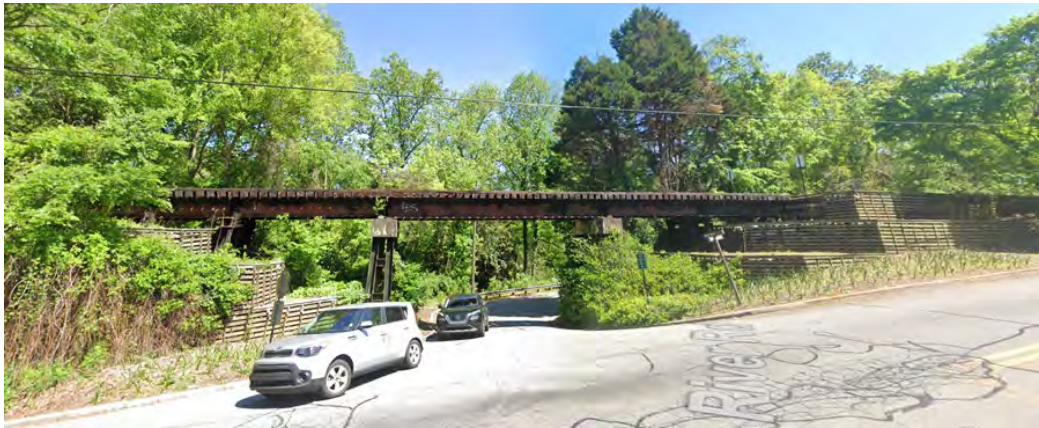
Figure 2. River Road Trestle
