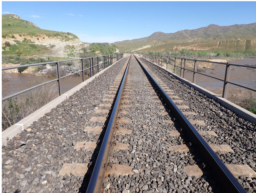
Figure 16: Bridge at MP 330.04
