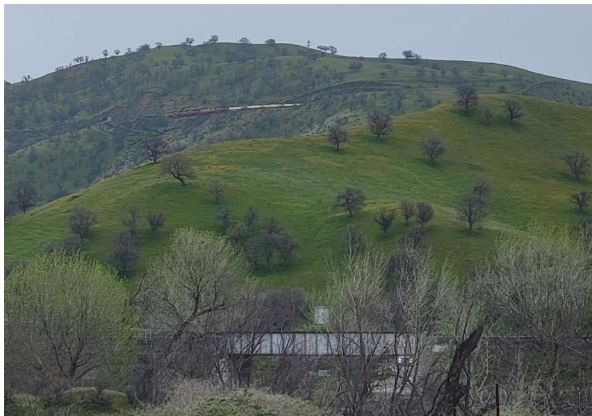
Figure 4: Near MP 335.2 (Bridge in foreground; BNSF train in background)
