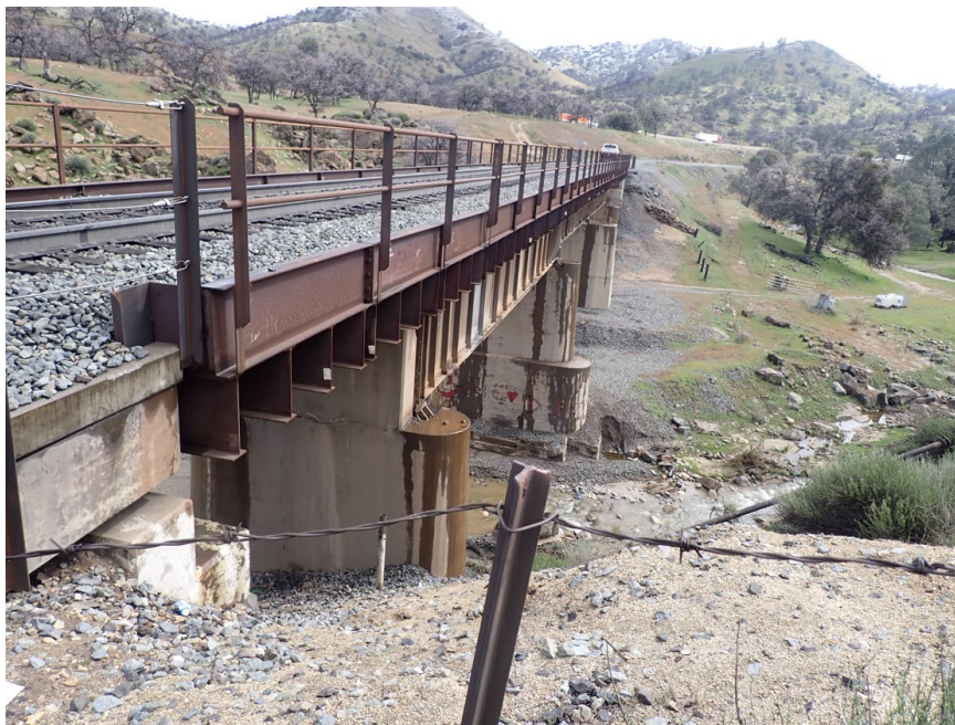
Figure 18: Bridge at MP 349.74
