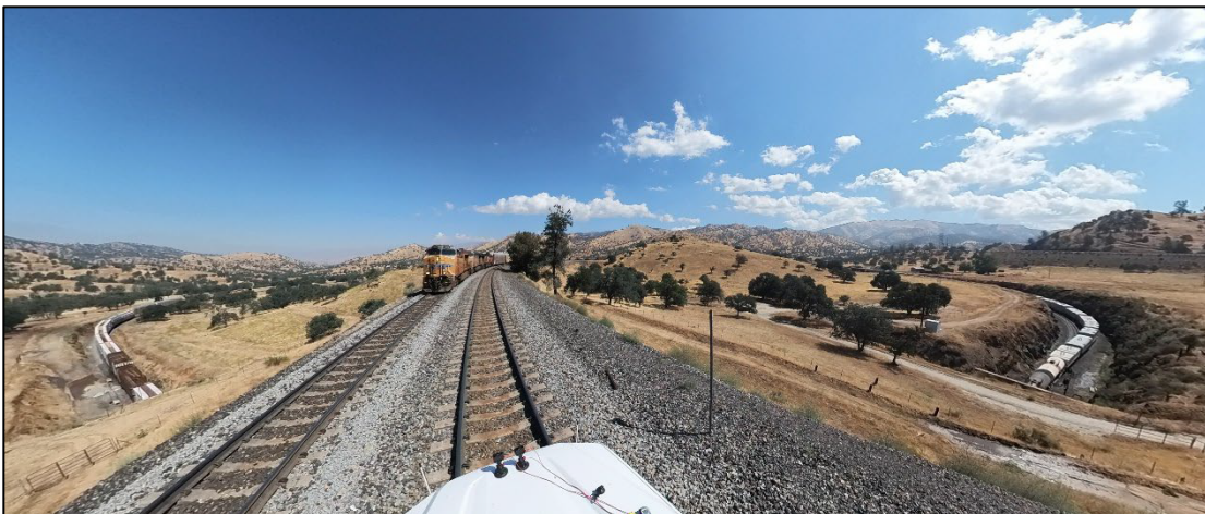
Photo 9. Looking north from MP 351.71 (above MP 351) at the top of the Tehachapi Loop. Note that the train extends from the west (left) through the tunnel to the east (right) and its head end is to the north. 8/22/2023.
