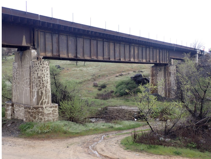
Figure 17: Bridge at MP 346.83
