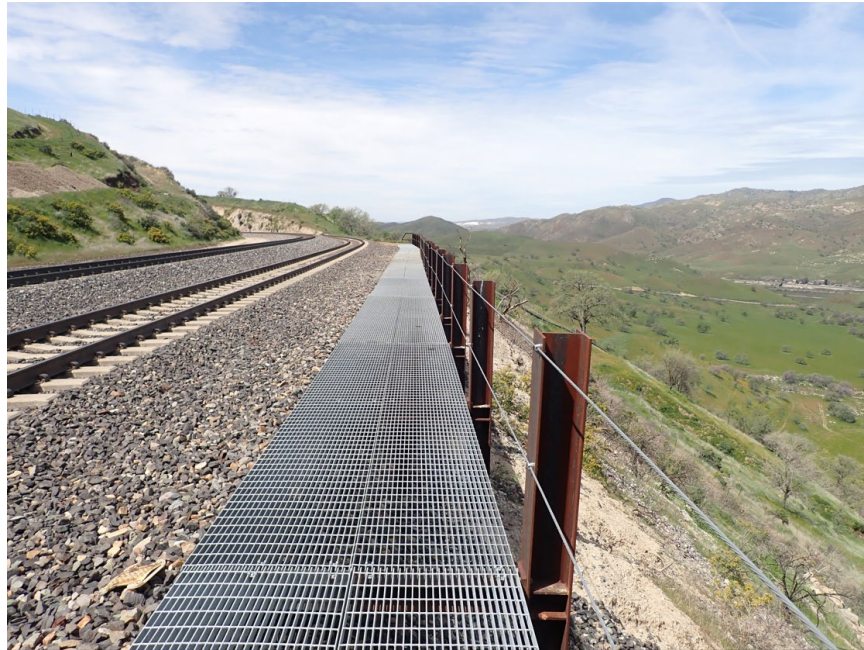
Figure 20: View of Elevated Walkway
