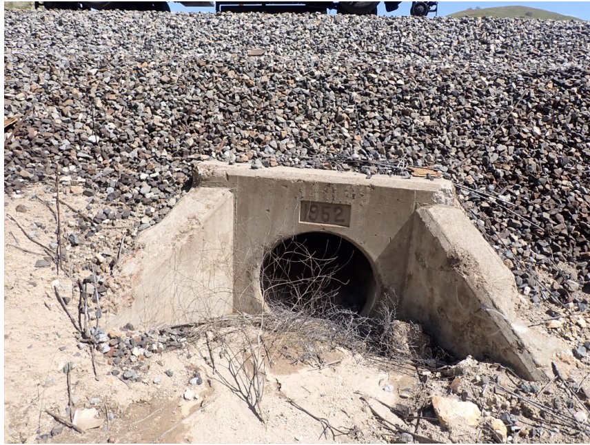
Figure 11: Corrugated Metal Pipe Culvert at MP 340.99
