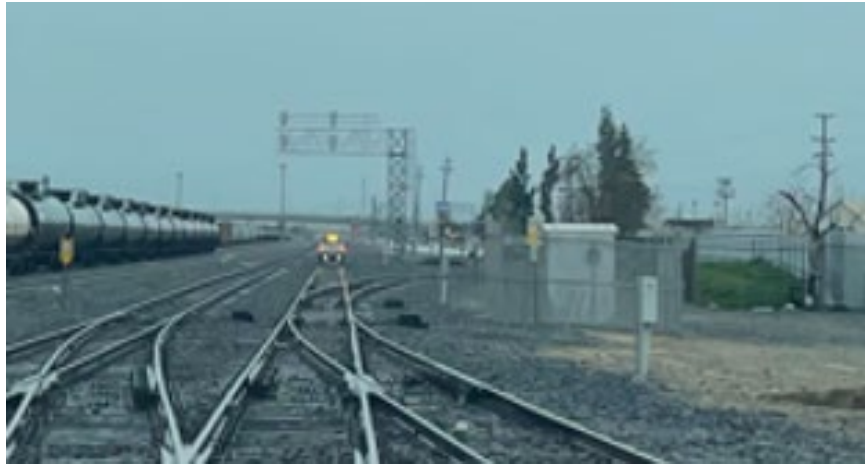
Figure 24: Cantilevered Signal at Kern Junction
