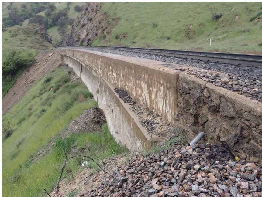
Figure 14: Cast-In-Place Concrete Wall at MP 343.83
