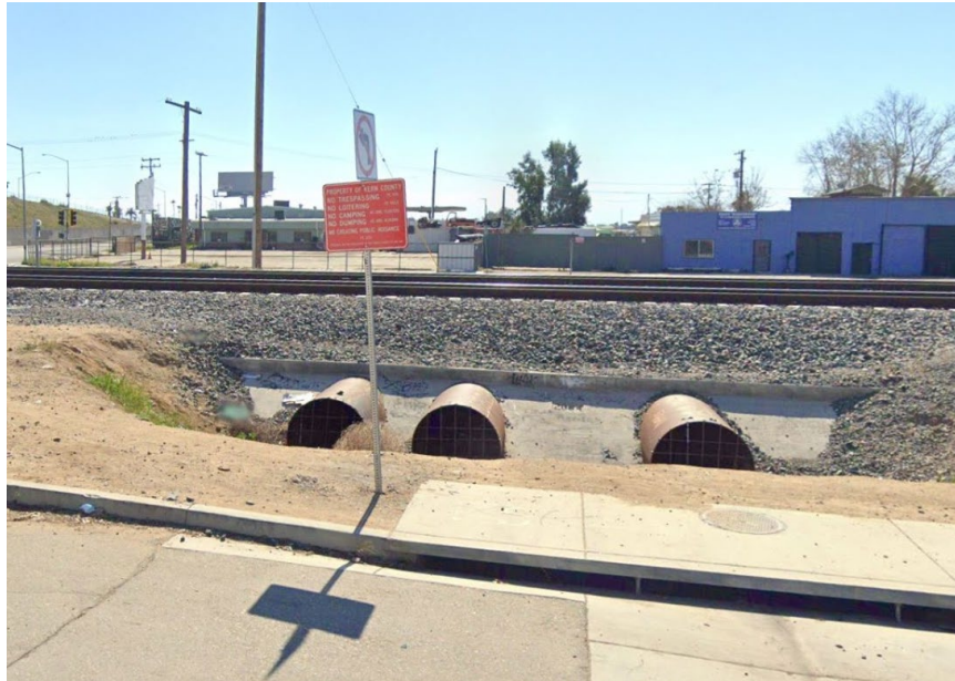
Figure 9: Smooth Steel Pipe Culvert at MP 316.45
