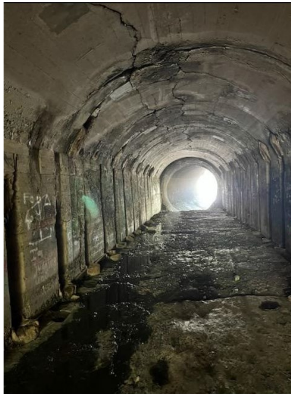
Figure 10: Concrete Arch Culvert at MP 358.27
