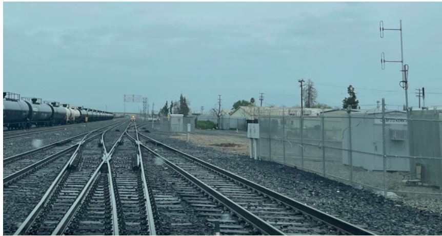
Figure 1: Kern Junction, near MP 313.56, looking east
