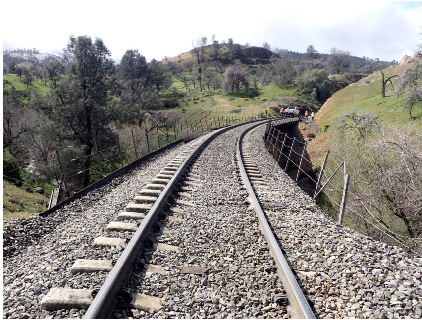
Figure 19: Bridge at MP 350.28
