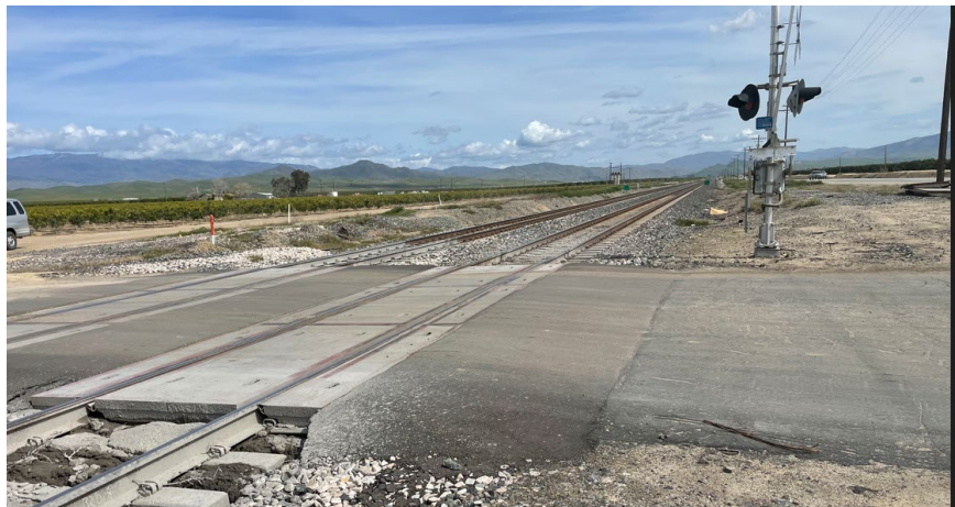
Figure 2: Between Kern Junction and Bena, looking east
