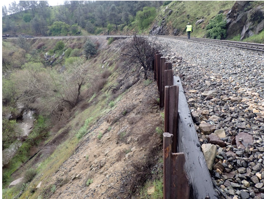
Figure 15: Rail Pile Wall at MP 344.66
