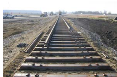
Figure 14 - Steel tie construction at the Manly Logistics Park, 2014
