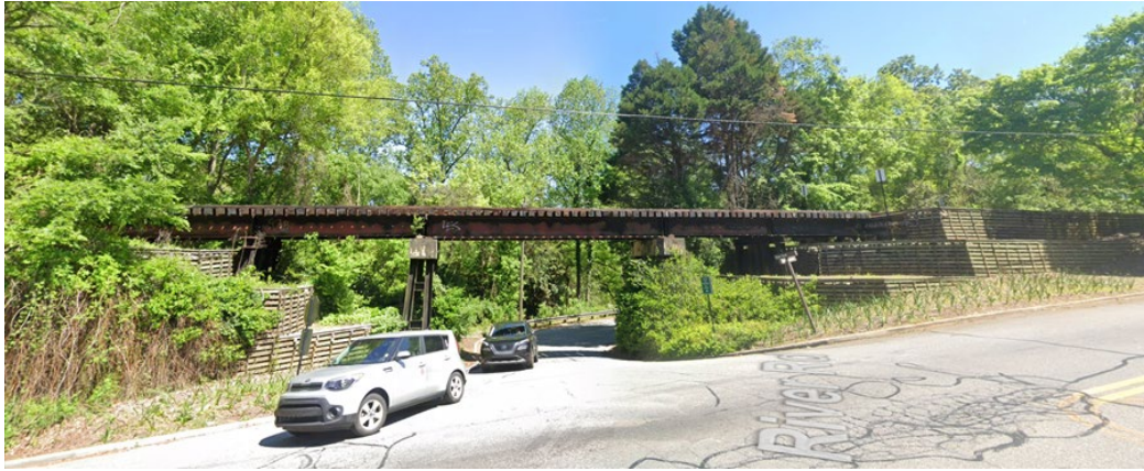
Figure 2. River Road Trestle
