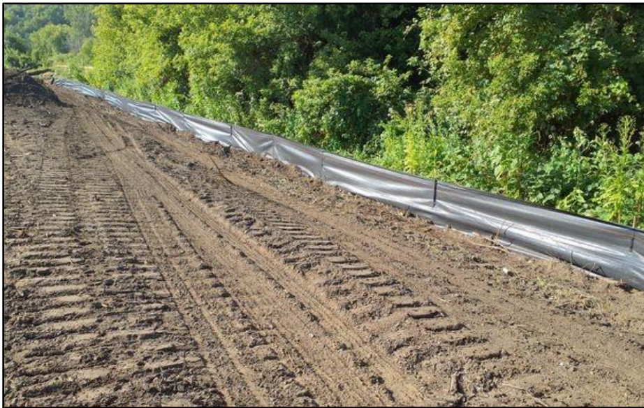
Figure 4. Silt fence installation progress; view facing south. (Photo by C. Christiansen September 14, 2023).
