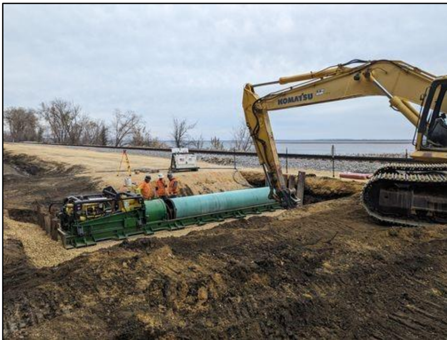
Figure 7. Drilling rig preparing to drill the culvert; view facing northeast. (Photo by S. Peterson November 16, 2023).
