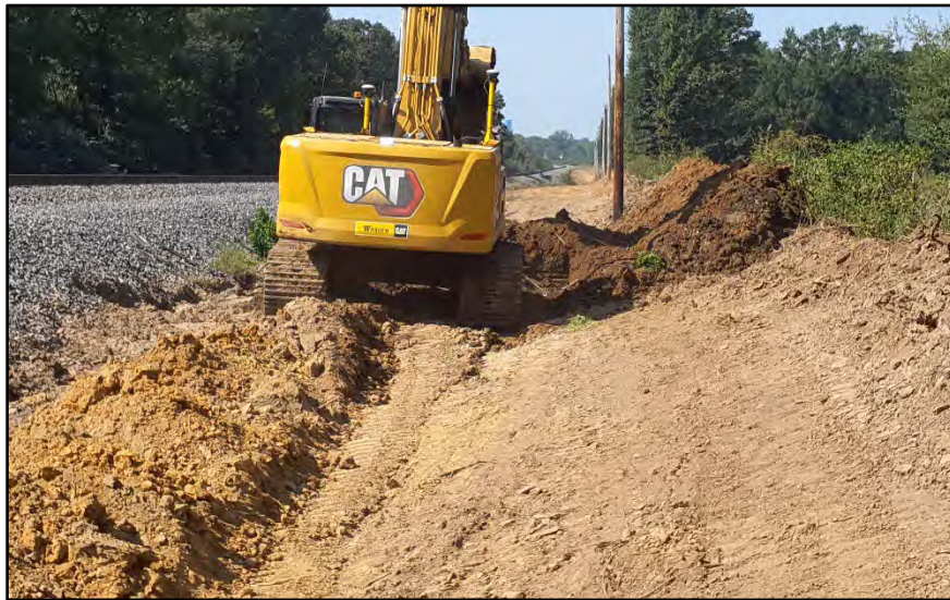
Figure 2. Excavating along the right-of-way; view facing southwest. (Photograph by T. Himebaugh 8/24/23.)
