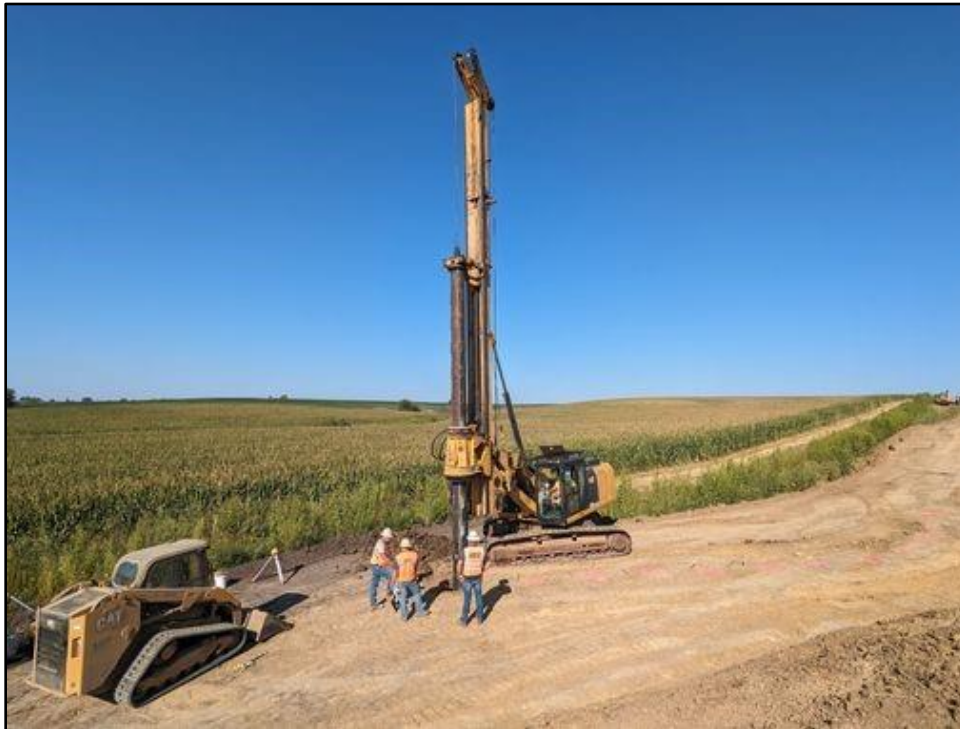
Figure 4. Overview of the bore crew drilling holes for wall beams; facing northeast. (Photograph by S. Peterson, August 30, 2023.)
