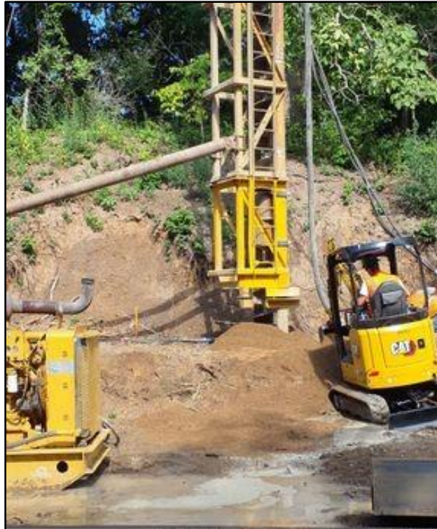
Figure 5. Drilling a hole for the retaining wall; view facing northwest. (Photograph by Randy Teboe, August 11, 2023.)
