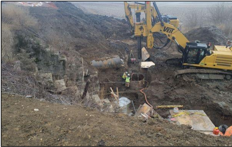
Figure 11. Drilling and construction area undergoing routine prep work; view facing west. (Photograph by T. Himebaugh, December 4, 2023.)
