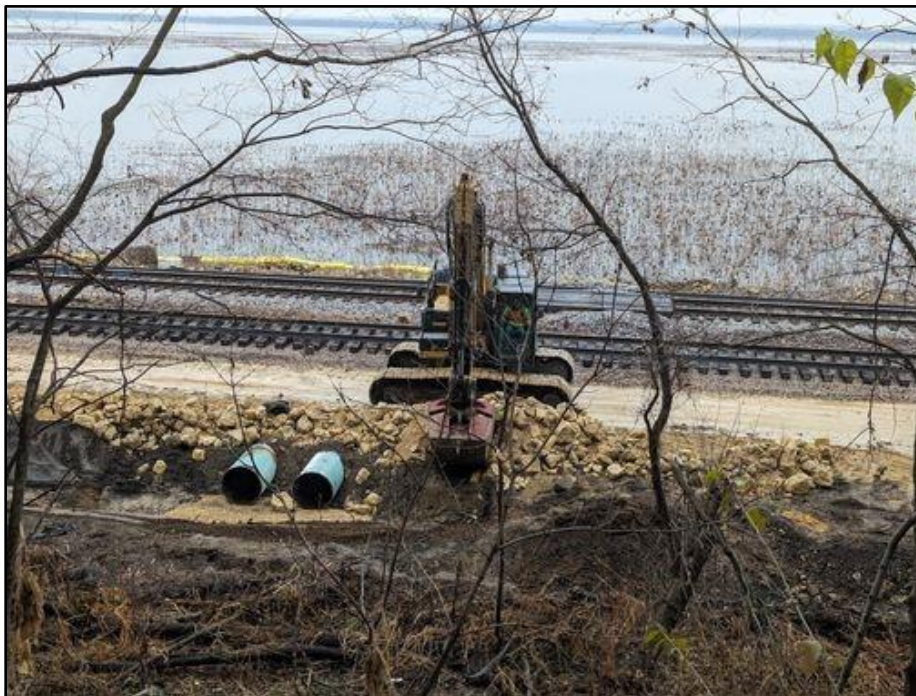
Figure 9. Rail installation and culvert cleanup; view facing west. (Photo by S. Peterson December 2, 2023).
