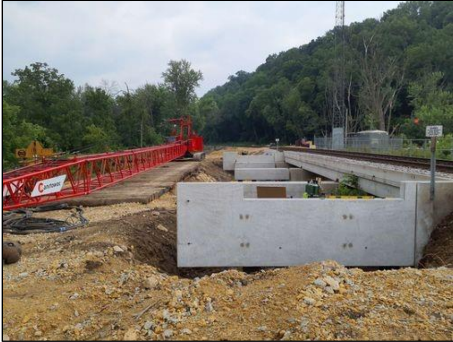
Figure 3. Bridge construction progresses toward the end of the workday; view facing south. (Photo by T. Schade June 26, 2023).
