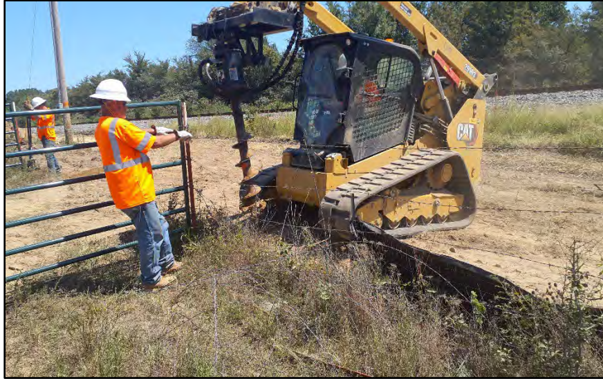
Figure 5. Drilling for post installation; view facing east. (Photograph by T. Himebaugh 9/1/23.)
