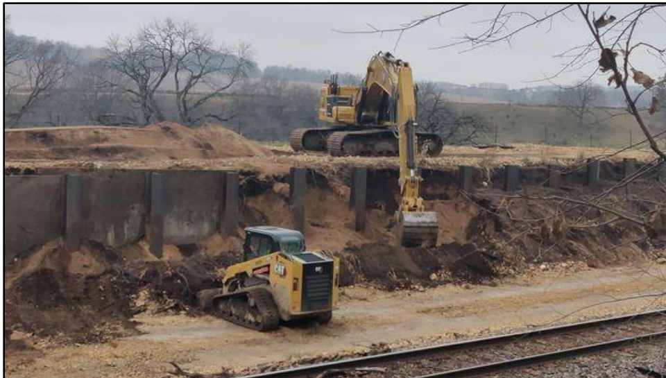
Figure 9. Continued excavation from above and below retaining wall; view facing northwest. (Photograph by Monica Zsigmond, December 5, 2023.)
