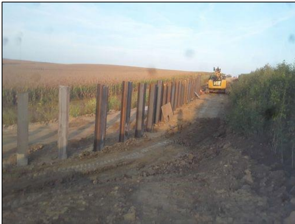
Figure 6. Drilling continues throughout the day, wall installation; view facing east. (Photograph by S. Cohen, September 18, 2023.)
