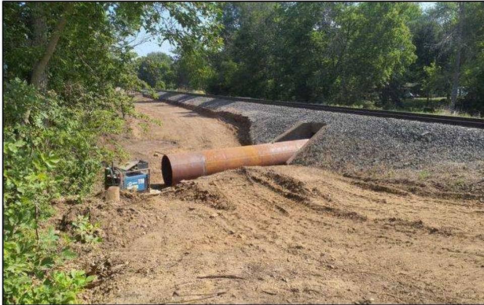
Figure 3. Culvert installation; view facing north. (Photograph by Wyatt Benson, June 21, 2023.)
