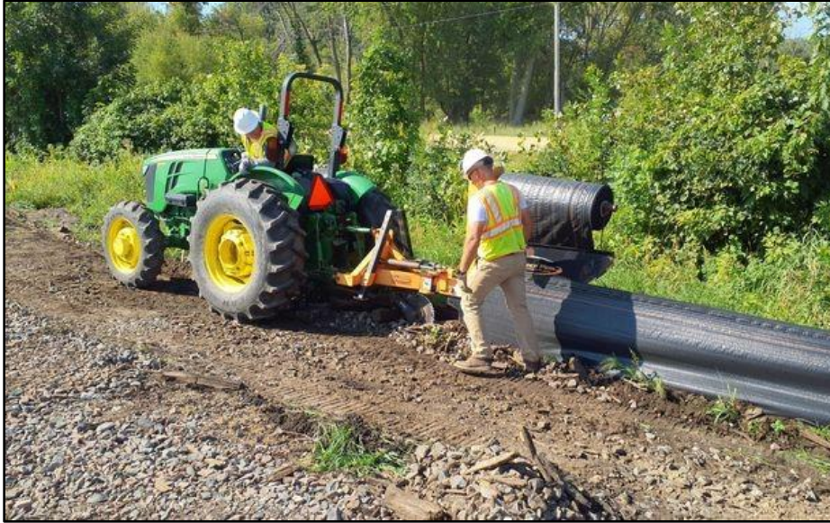
Figure 4. Silt fence installation progresses; view facing southeast. (Photo by C. Christiansen September 15, 2023).
