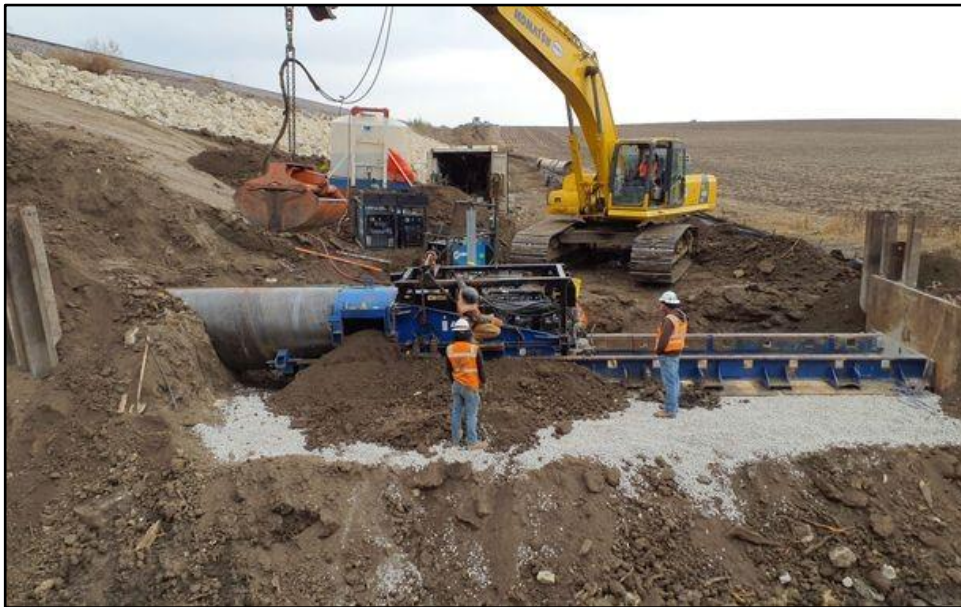
Figure 8. Pipe boring under the track. First run is all backfill, containing 20 percent large ballast rock; view facing east. (Photograph by T. Schade, October 18, 2023.)
