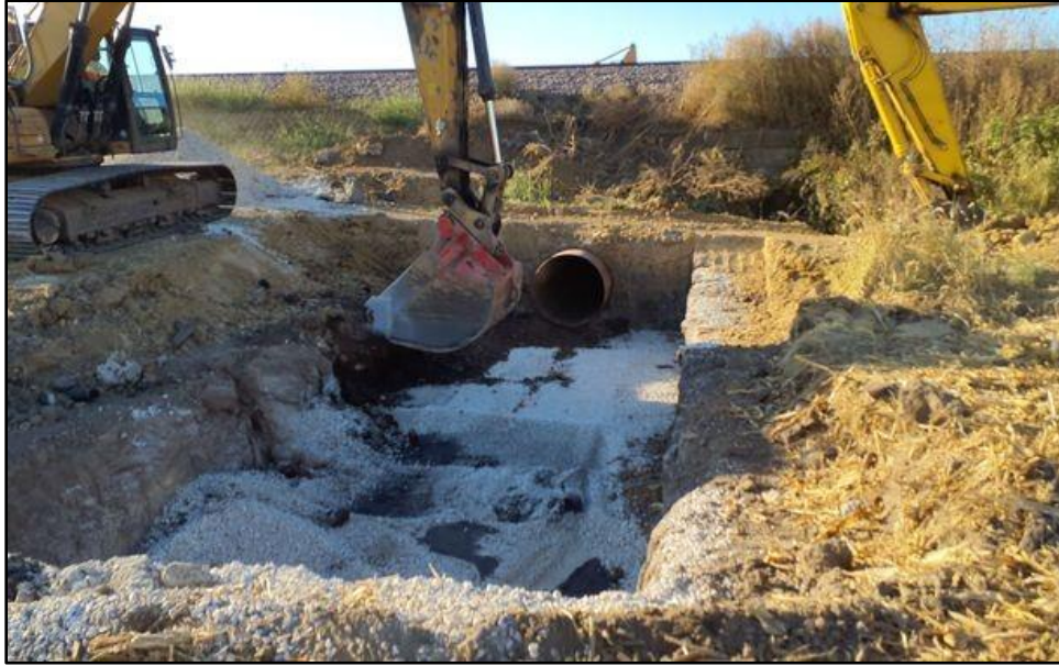
Figure 7. Trenching progress around culvert; view facing south. (Photograph by T. Schade, October 9, 2023.)
