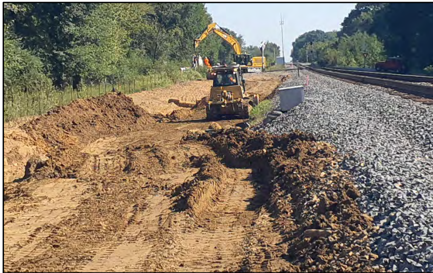
Figure 10. Spreading fill dirt along the right-of-way; view facing northeast. (Photograph by T. Himebaugh 9/27/23.)
