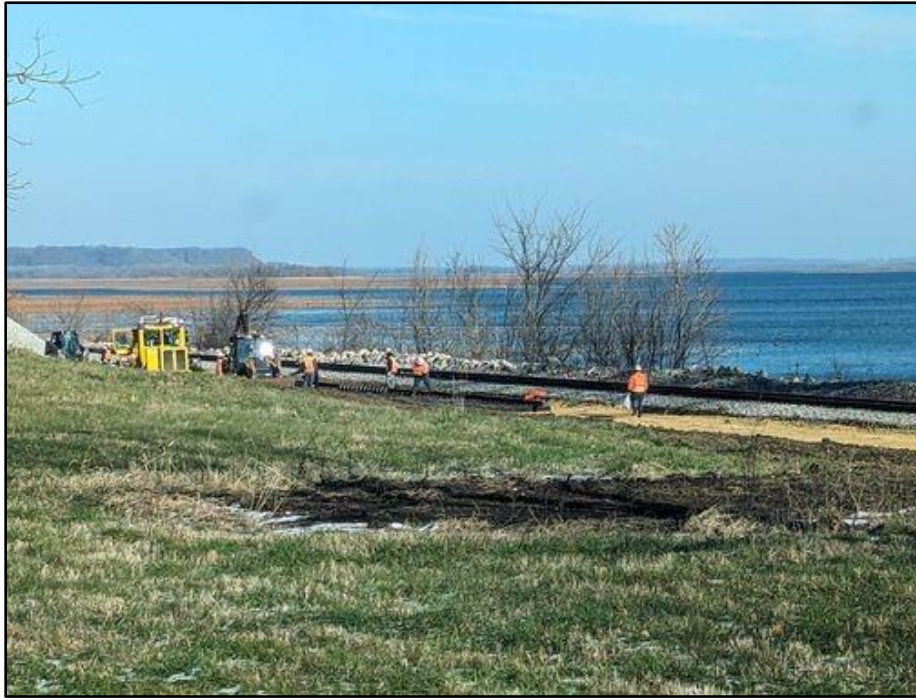
Figure 8. Rail installation; view facing northeast. (Photo by S. Peterson November 30, 2023).
