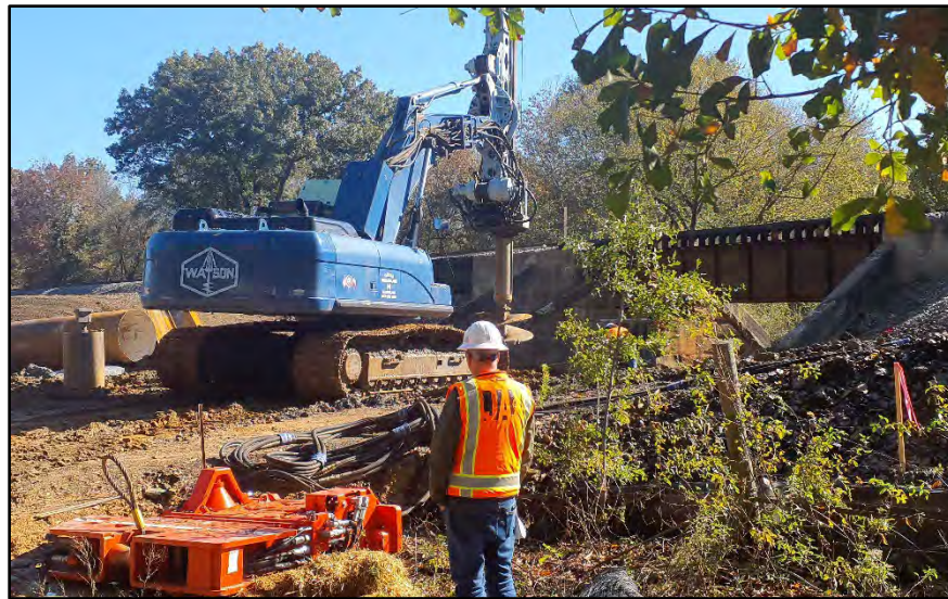
Figure 14. Drilling for beam installation; view facing east. (Photograph by T. Himebaugh 10/30/23.)
