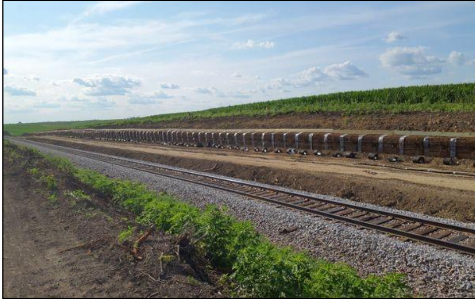
Figure 3. Overview of mesh soil fence; facing northwest. (Photograph by T. Schade, June 26, 2023.)
