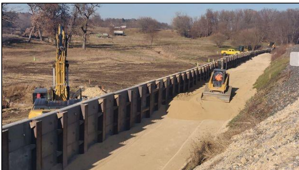
Figure 10. Continued excavation of borrow pit; view facing north. (Photograph by Monica Zsigmond, December 14, 2023.)
