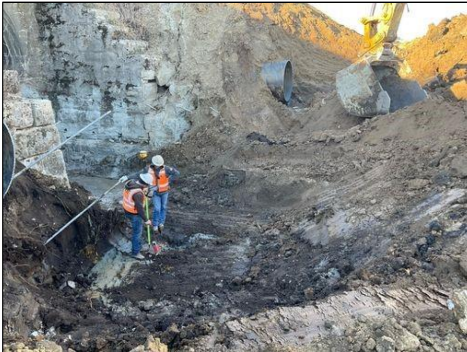
Figure 10. Overview of the culvert installation and cleanup work; facing west.
