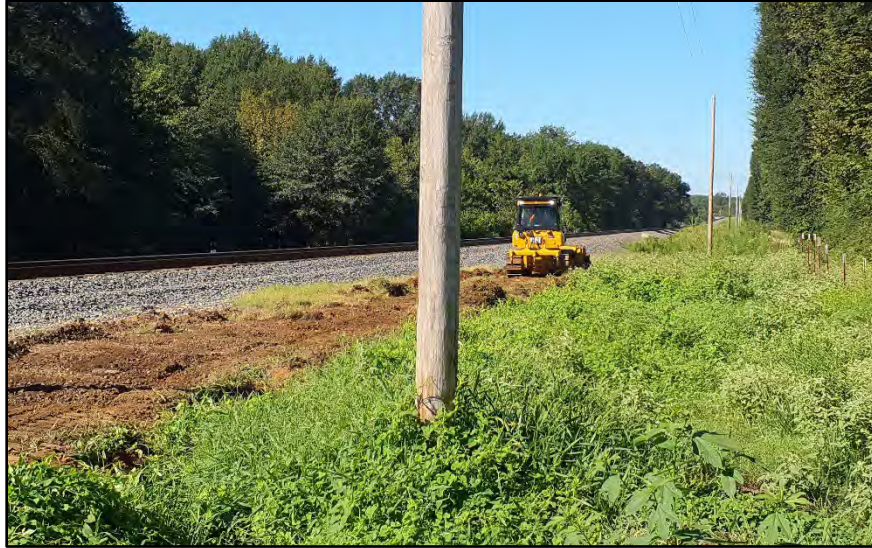
Figure 1. Initial topsoil clearance by a bulldozer; view facing southwest. (Photograph by T. Himebaugh 8/15/23.)
