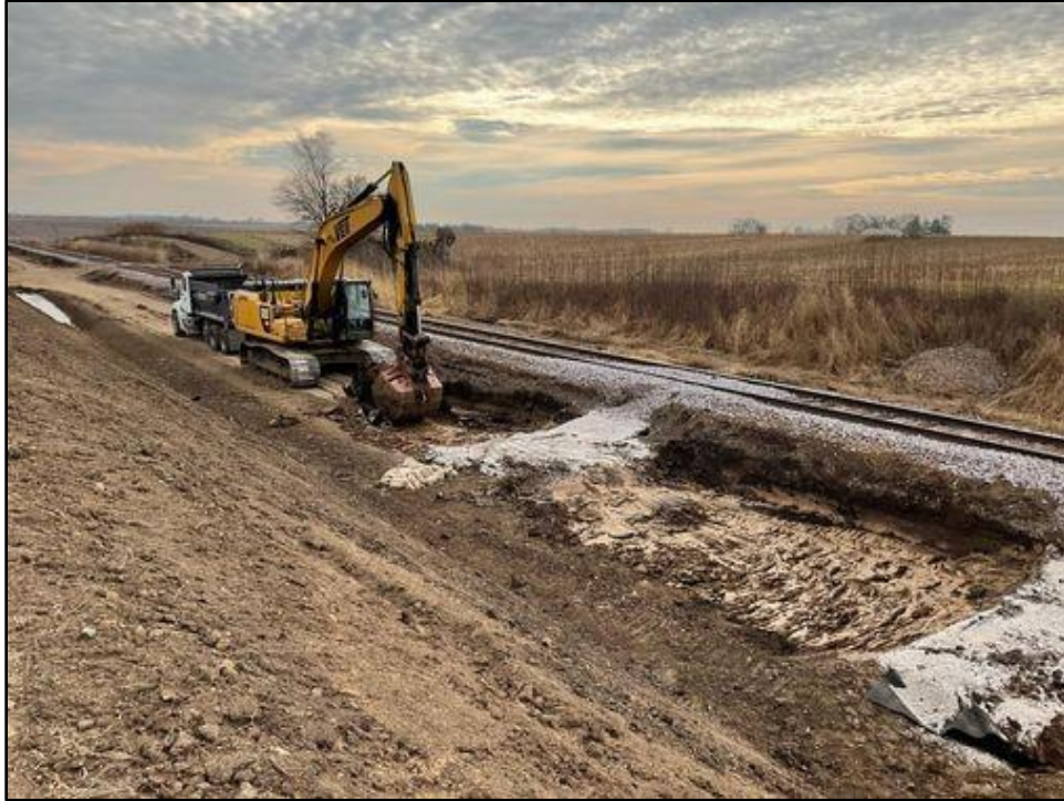
Figure 9. Overview of the excavations for the access road; facing southwest.
