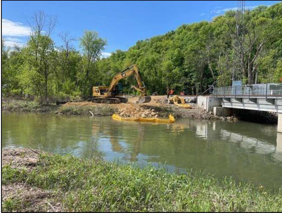
Figure 1. Track hoe laying rock to build up pad for bridge on south bank; view facing south (Photo by S. Cohen May 16, 2023).
