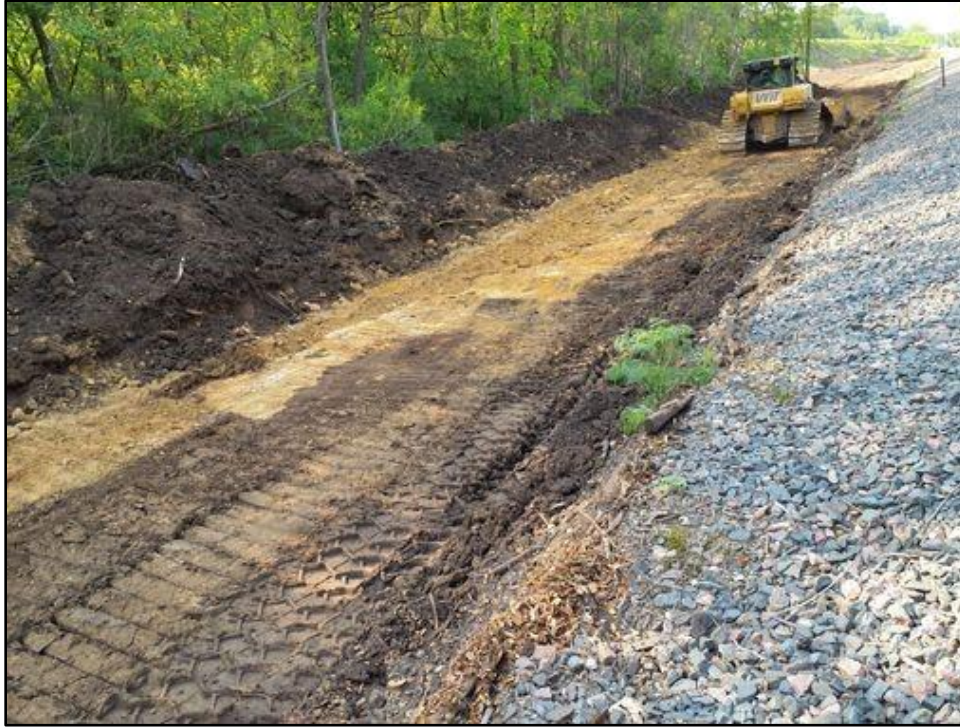
Figure 1. Initial topsoil clearance and stump removal by bulldozer; view facing southwest. (Photograph by Tatiana Hargrove, May 23, 2023.)
