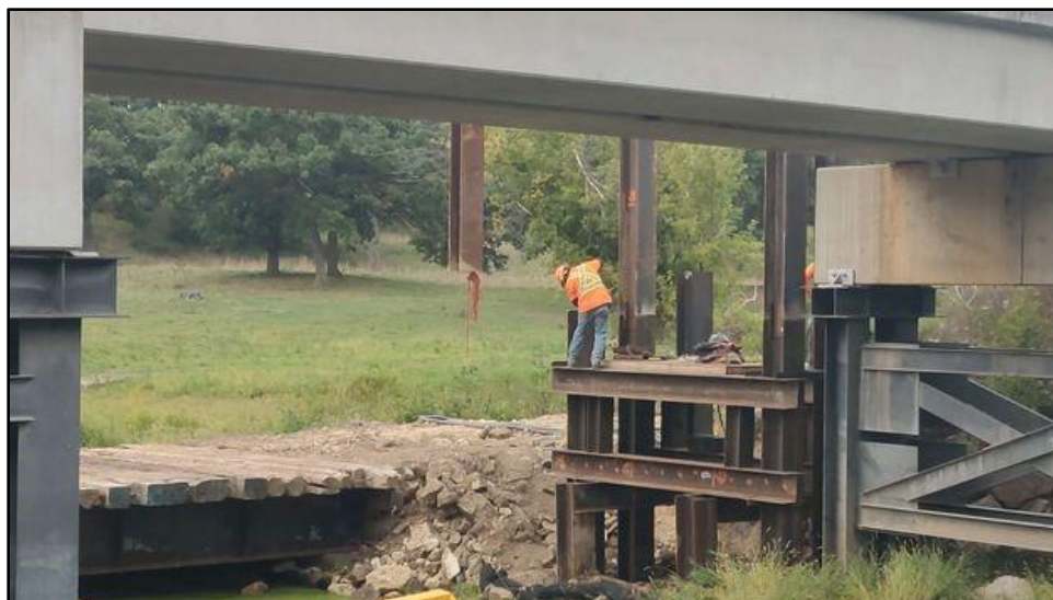
Figure 6. Preparing to begin driving pylon; view facing east. (Photograph by Monica Zsigmond, September 26, 2023.)
