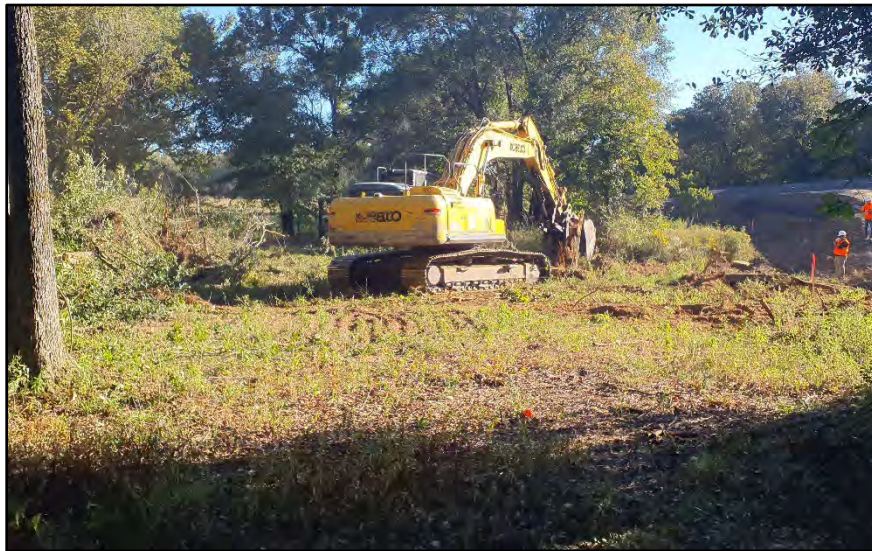
Figure 12. Tree limbing to assist with inserting culvert pipe extension; view facing northeast. (Photograph by T. Himebaugh 10/9/23.)
