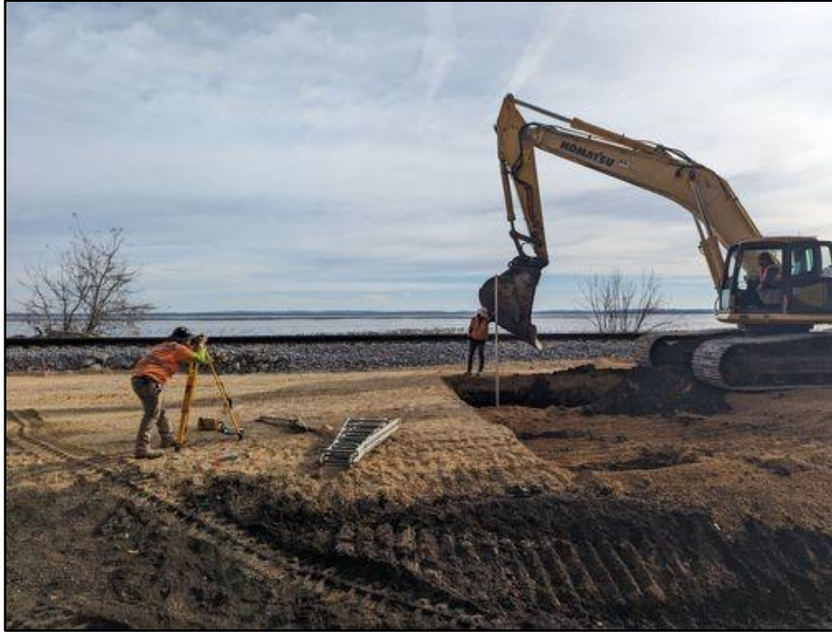
Figure 6. Digging a pit for culvert drilling operations; view facing east. (Photo by S. Peterson November 16, 2023).
