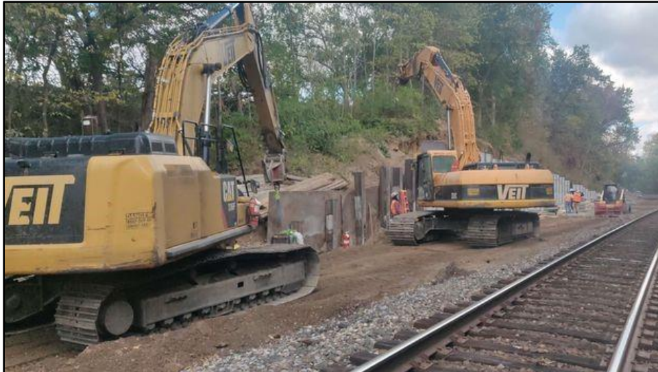
Figure 7. Excavation between pilings, installation of wall panels; view facing northwest. (Photograph by Monica Zsigmond, October 7, 2023.)
