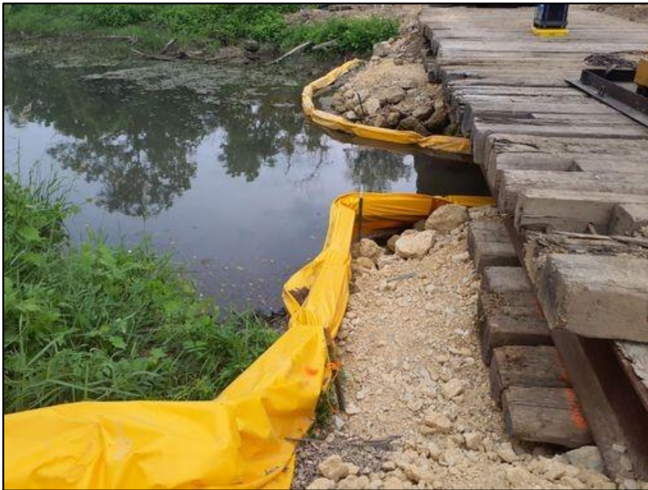
Figure 2. Example of turbidity curtains/silt screens set up along Deer Creek on either side of area of potential effects where bridge is being installed around MP 152; view facing south. (Photo by H. MacIsaac June 7, 2023).
