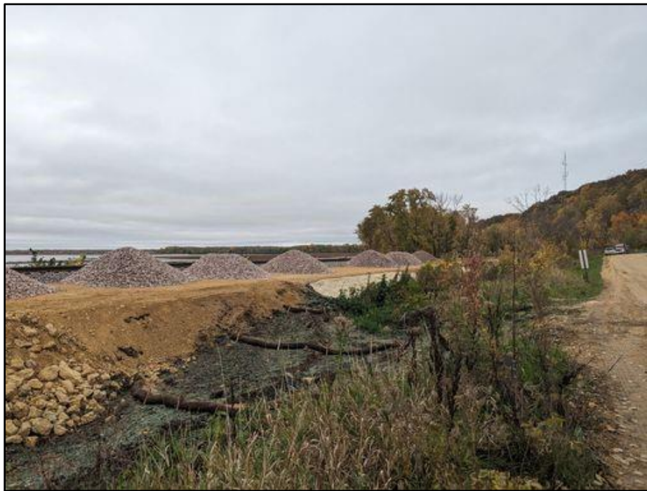
Figure 5. Track ballast stone installation progress; view facing north. (Photo by S. Peterson October 27, 2023).
