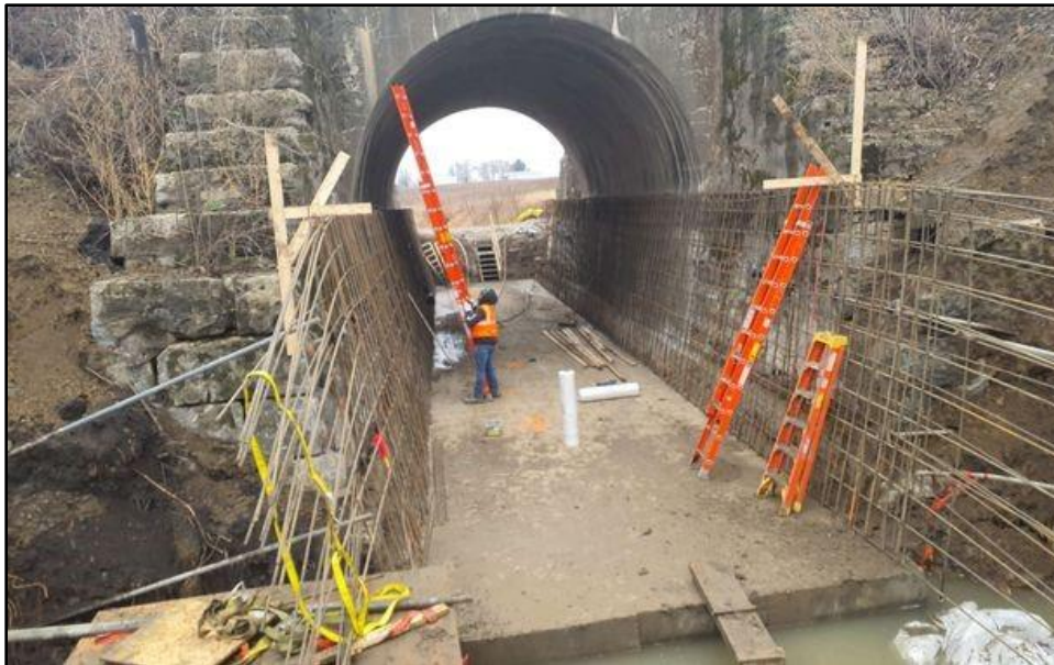
Figure 12. Overview of progress on rebar mesh; facing south. (Photograph by T. Himebaugh, December 5, 2023.)
