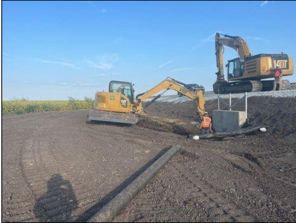
Figure 5. Excavator moving topsoil by a culvert on west side of project area; view facing east. (Photograph by S. Cohen, September 5, 2023.)
