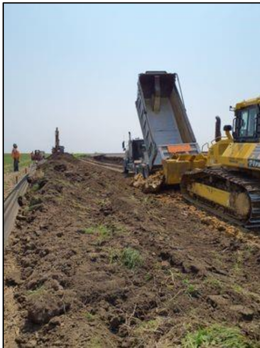
Figure 2. Bulldozer and dump truck adding rock fill to areas where topsoil was removed; view facing east. (Photograph by R. Teboe, June 22, 2023.)
