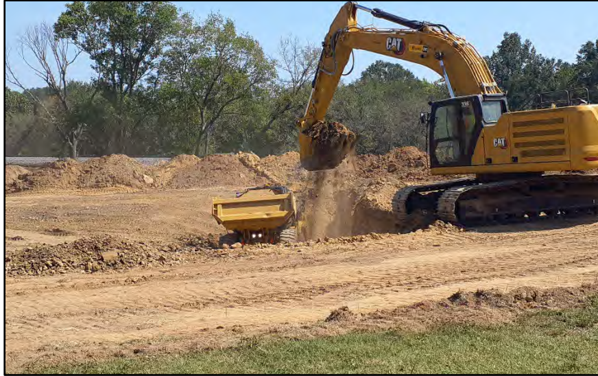
Figure 9. Continued excavation of borrow pit; view facing southeast. (Photograph by T. Himebaugh 9/18/23.)
