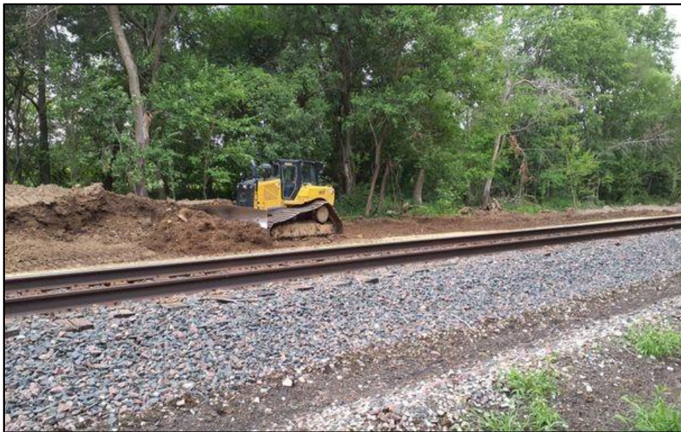
Figure 4. Topsoil and stump removal; view facing west. (Photograph by Wyatt Benson, July 5, 2023.)
