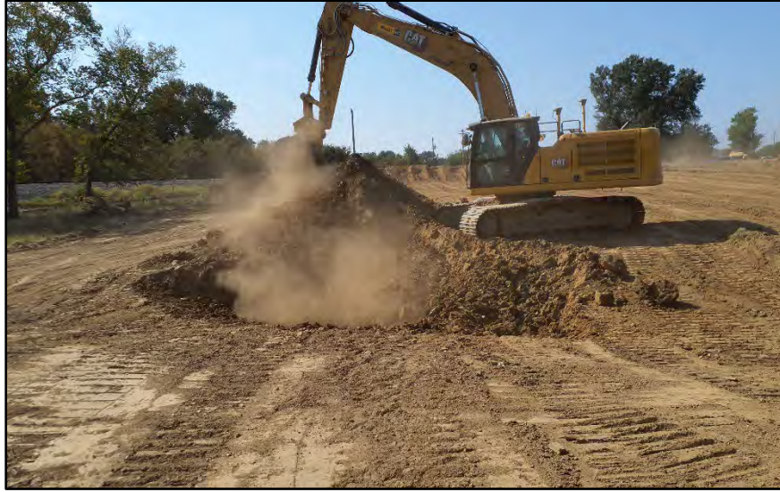
Figure 7. Excavation of borrow pit after topsoil clearance; view facing southwest. (Photograph by R. Campbell 9/5/23.)
