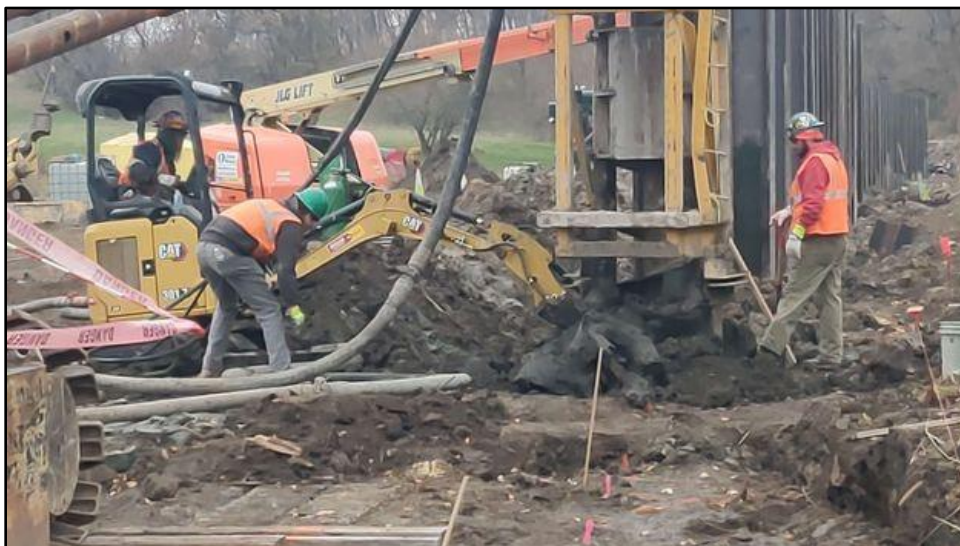
Figure 8. Drilling to prepare for pylon installation; view facing southwest. (Photograph by Monica Zsigmond, November 8, 2023.)
