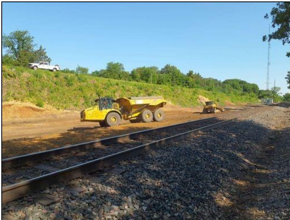
Figure 2. Initial stump removal by excavator; view facing northwest. (Photograph by Matthew Denno, June 12, 2023.)
