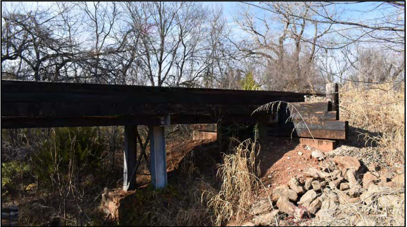
Streetscape Payne County, Stillwater, Oklahoma Along ATSF Bridge 4 east piers and north wingwall. Matt Corpolongo--ODOT Cultural Resources Program
