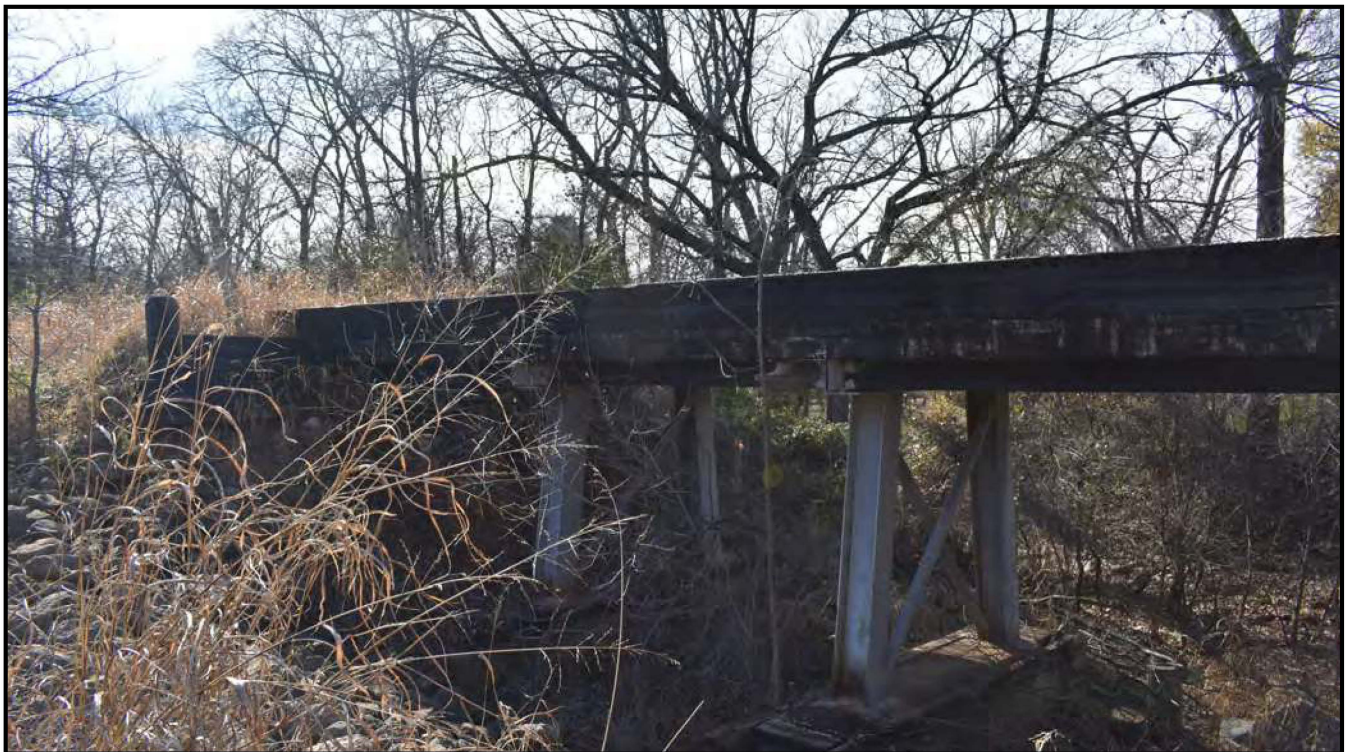
Streetscape Payne County, Stillwater, Oklahoma Along ATSF Bridge 4 east piers and south wingwall. Matt Corpolongo--ODOT Cultural Resources Program
