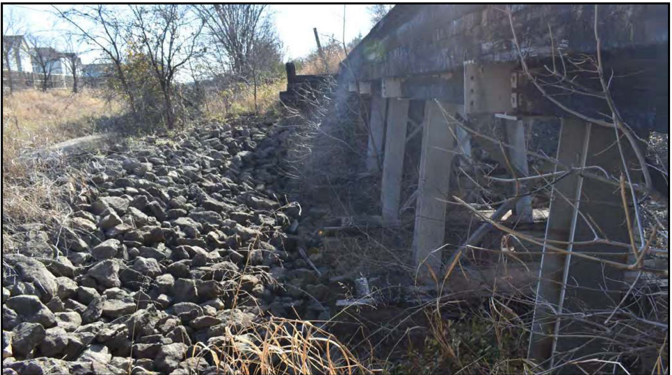
Streetscape Payne County, Stillwater, Oklahoma Along ATSF Bridge 4 east piers and deck. Matt Corpolongo--ODOT Cultural Resources Program
