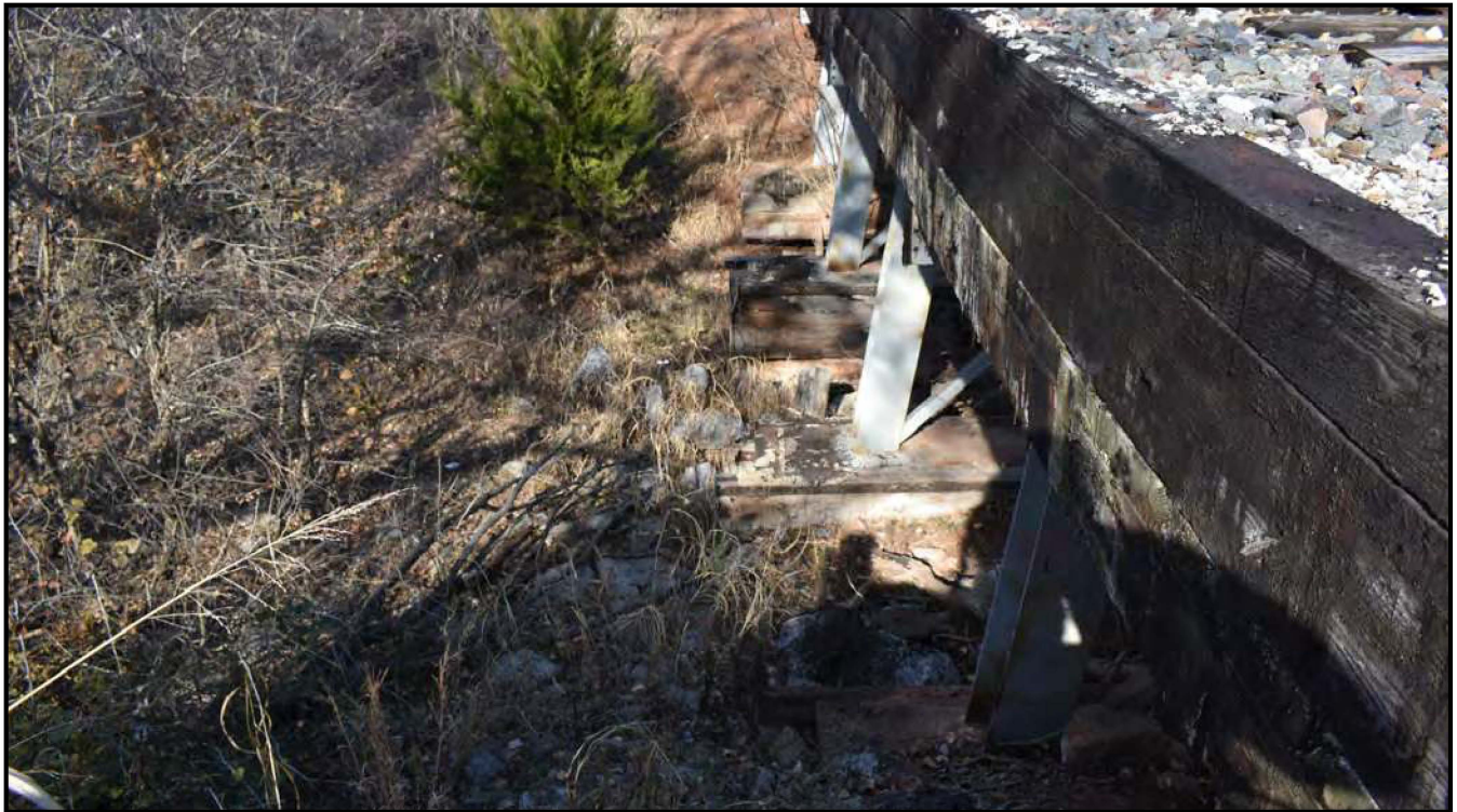
Streetscape Payne County, Stillwater, Oklahoma Along ATSF Bridge 4 west piers and deck. Matt Corpolongo--ODOT Cultural Resources Program
