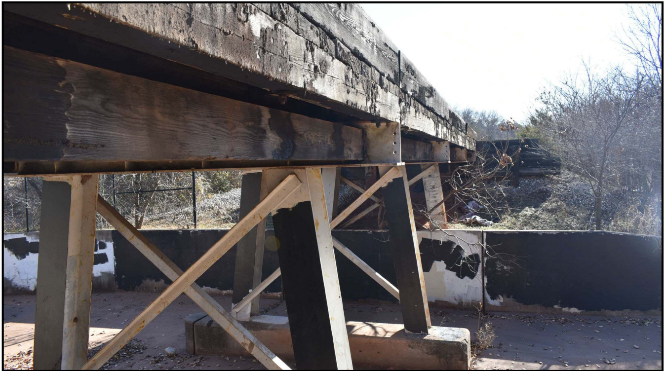
Streetscape Payne County, Stillwater, Oklahoma Along ATSF Bridge 3 west piers and deck. Matt Corpolongo—ODOT Cultural Resources Program
