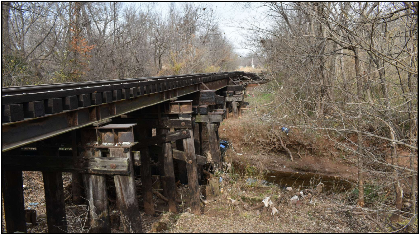
Streetscape Payne County, Stillwater, Oklahoma Along ATSF Bridge 1 piers and deck, east side. Matt Corpolongo--ODOT Cultural Resources Program
