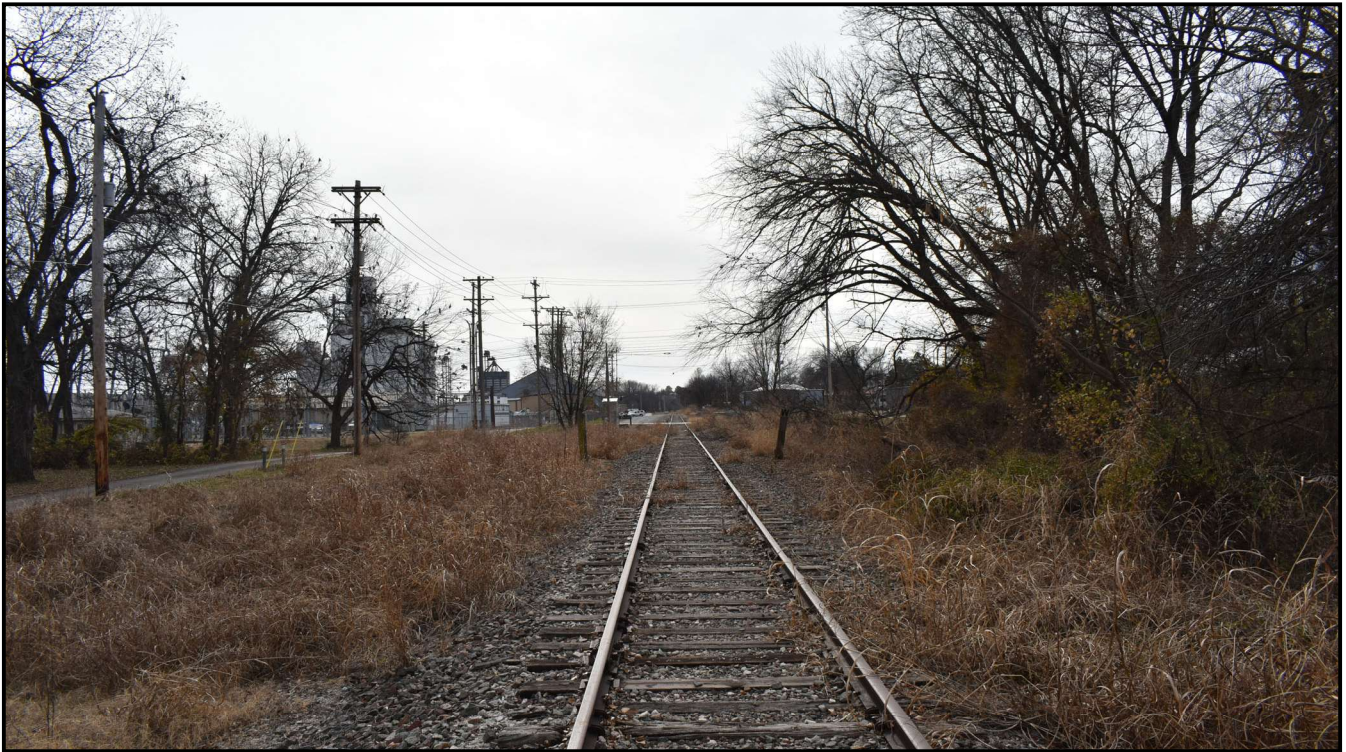
Streetscape Payne County, Stillwater, Oklahoma Along ATSF at E. Maple Ave. Matt Corpolongo--ODOT Cultural Resources Program
