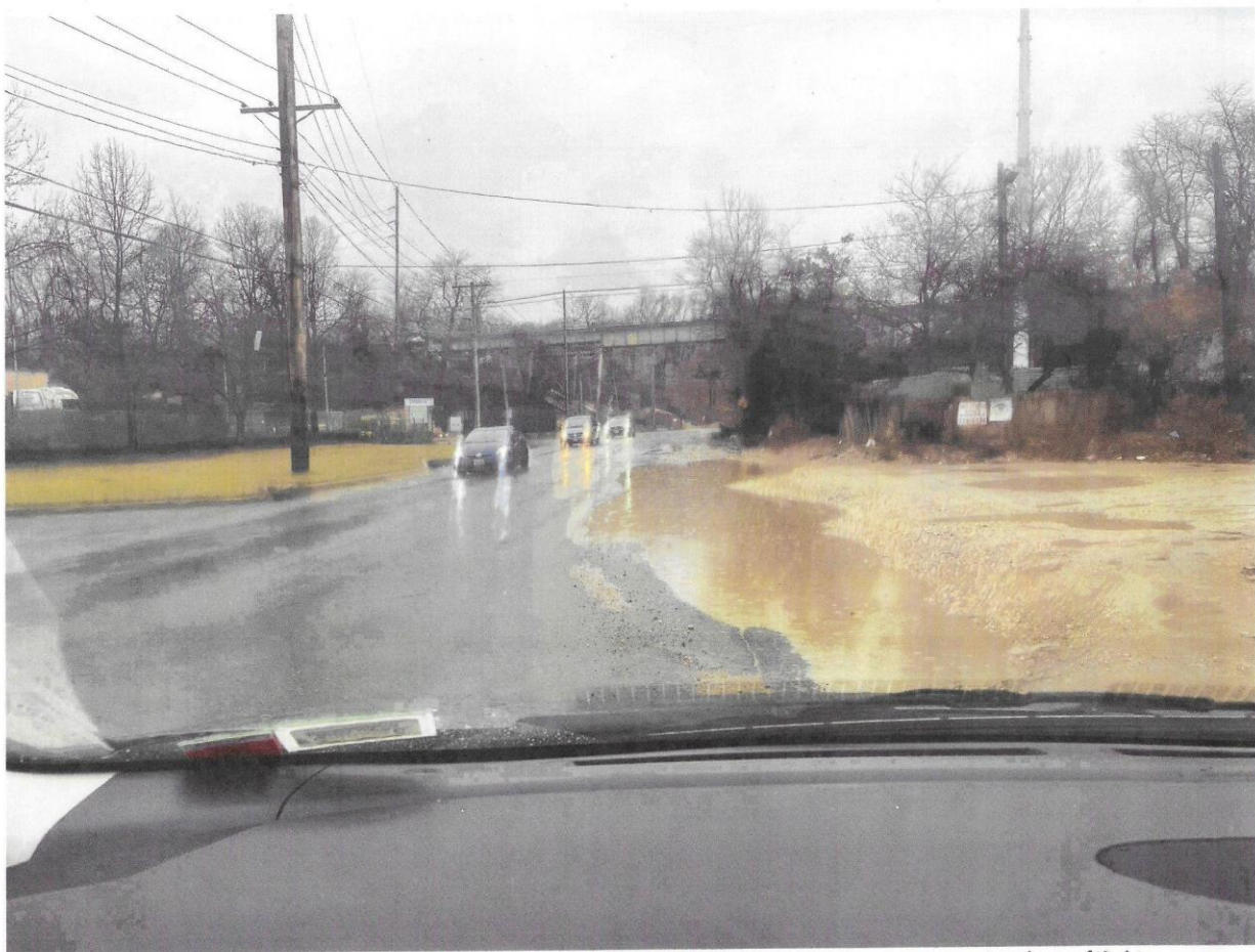
FLOODING ON TOWN LINE RD ACROSS FROM COUNTRY BEFORE RAILROAD BRIDGE
