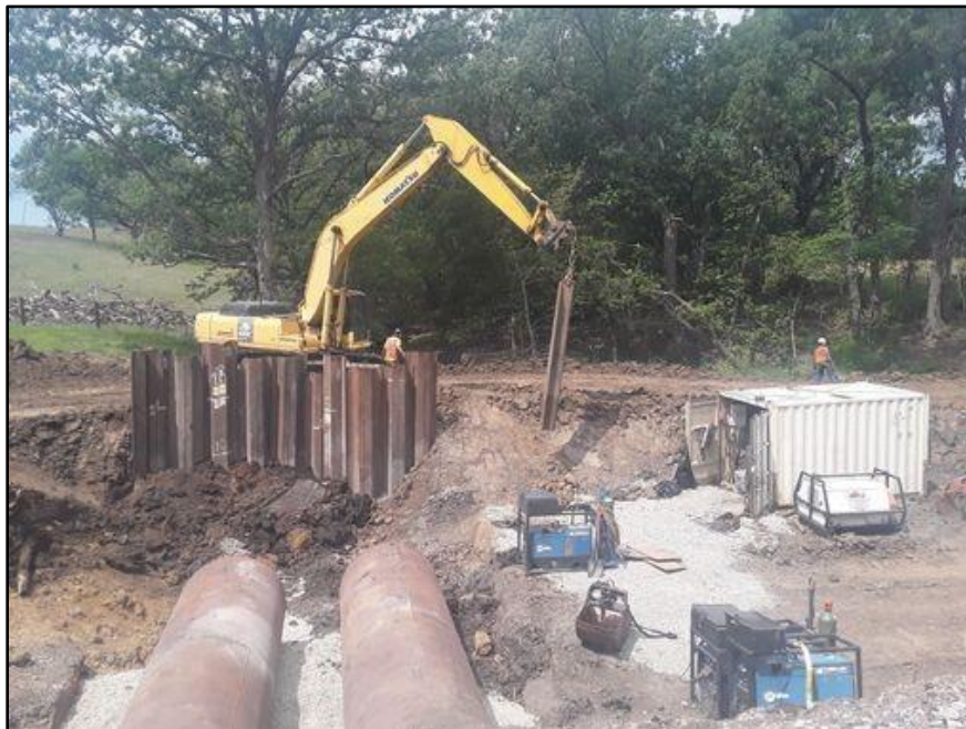
Figure 10. Iowa Trenchless finishing activities at the first culvert site; view facing northwest. (Photograph by S. Peterson 7/20/23.)
