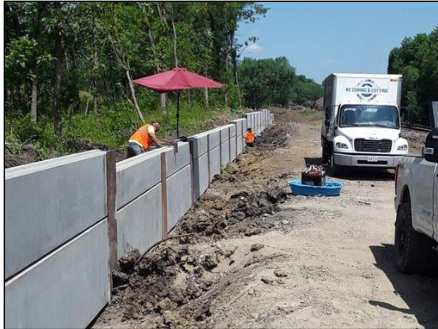
Figure 7. Crew placing the northern portion of the retaining wall north of the rail crossing; view facing north. (Photograph by S. Peterson 6/22/23.)
