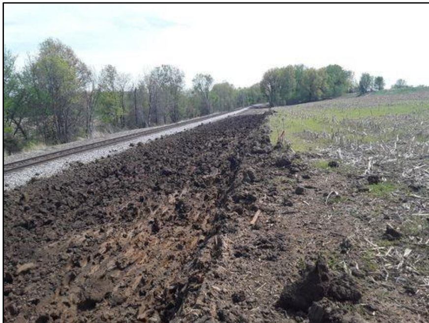
Figure 2. Topsoil removal continues toward the south end of the right-of-way; view facing south. (Photograph by S. Peterson 5/4/23.)
