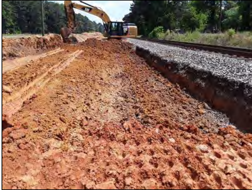
Figure 5. Excavator digging a trench; view facing east. (Photograph by R. Jenson May 18, 2023.)
