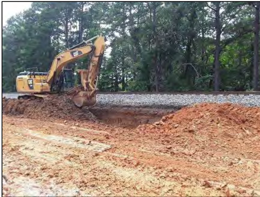
Figure 8. Cut-and-fill grading using fill from the borrow pit; view facing southwest. (Photograph by D. Holubar June 13, 2023.)
