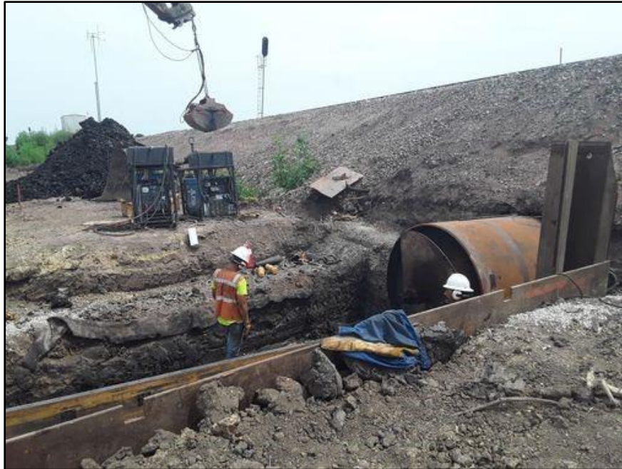
Figure 11. Close-up of the trenching pit and the culvert; view facing northeast. (Photograph by S. Peterson 7/25/23.)
