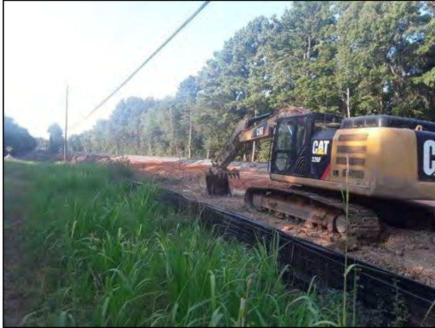
Figure 9. Continued excavation of borrow pit; view facing southeast. (Photograph by H. Moore July 28, 2023.)
