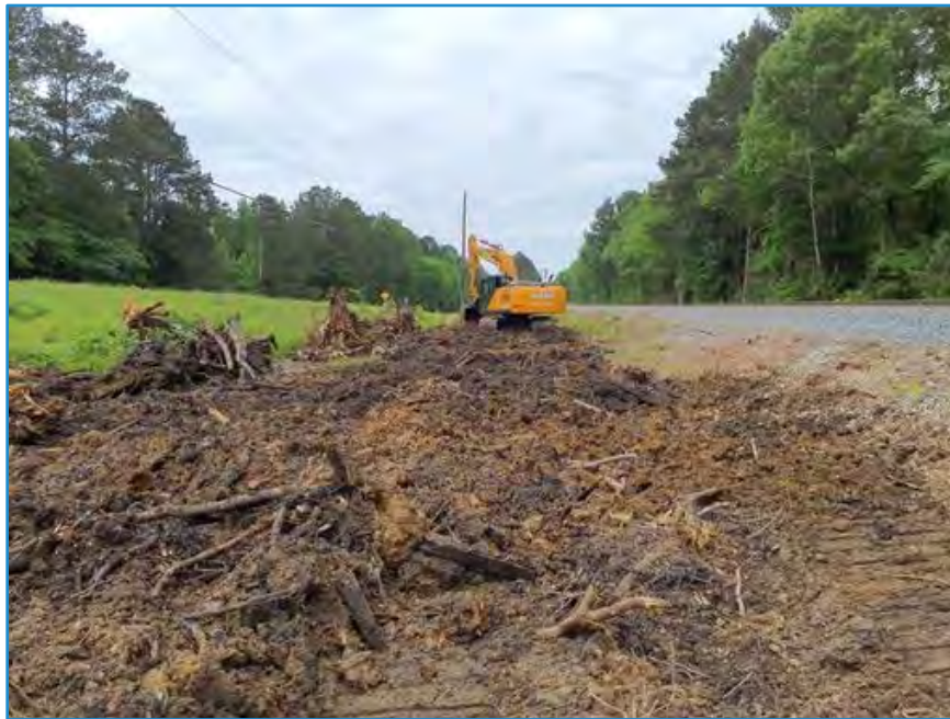
Figure 2. Initial stump removal by an excavator; view facing southwest. (Photograph by H. MacIsaac April 24, 2023.)
