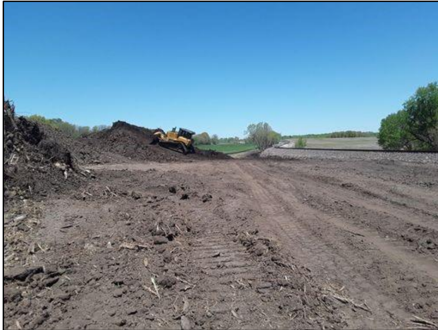
Figure 1. Bulldozer stockpiling topsoil on the right-of-way; view facing north. (Photograph by S. Peterson 5/3/23.)
