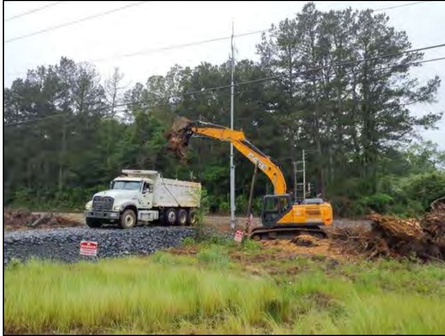
Figure 3. Tree removal by excavator; view facing southwest. (Photograph by H. MacIsaac April 29, 2023.)
