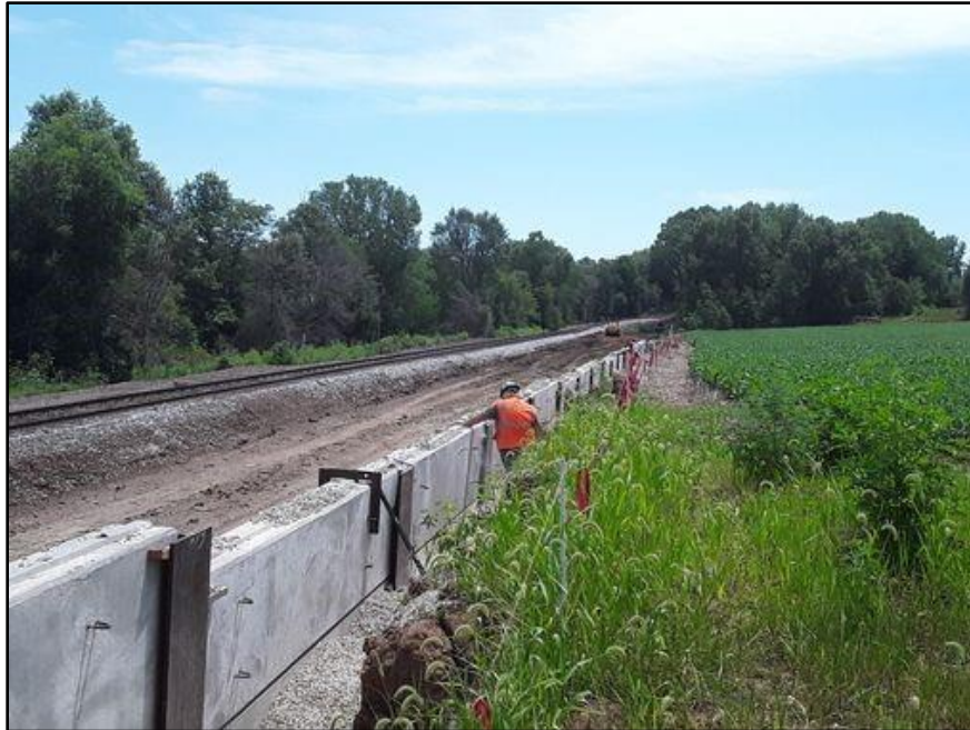
Figure 9. Foundation crew working on the southern portion of the retaining wall; view facing southeast. (Photograph by S. Peterson 7/14/23.)
