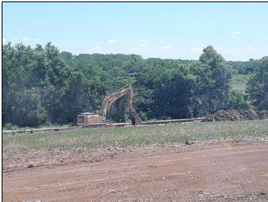
Figure 6. Trenching along the corridor; view facing east. (Photograph by S. Peterson 6/19/23.)
