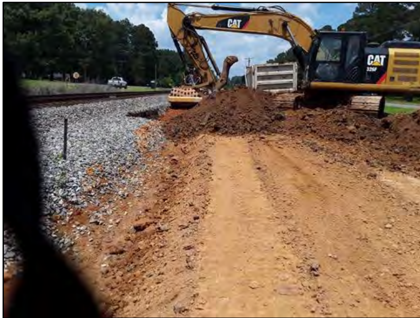
Figure 6. Excavator digging a culvert installation trench; view facing east. (Photograph by R. Jenson May 18, 2023.)
