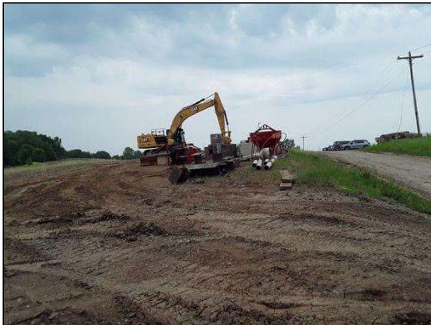
Figure 4. Construction staging area on top of the hill; view facing south. (Photograph by S. Peterson 6/7/23.)
