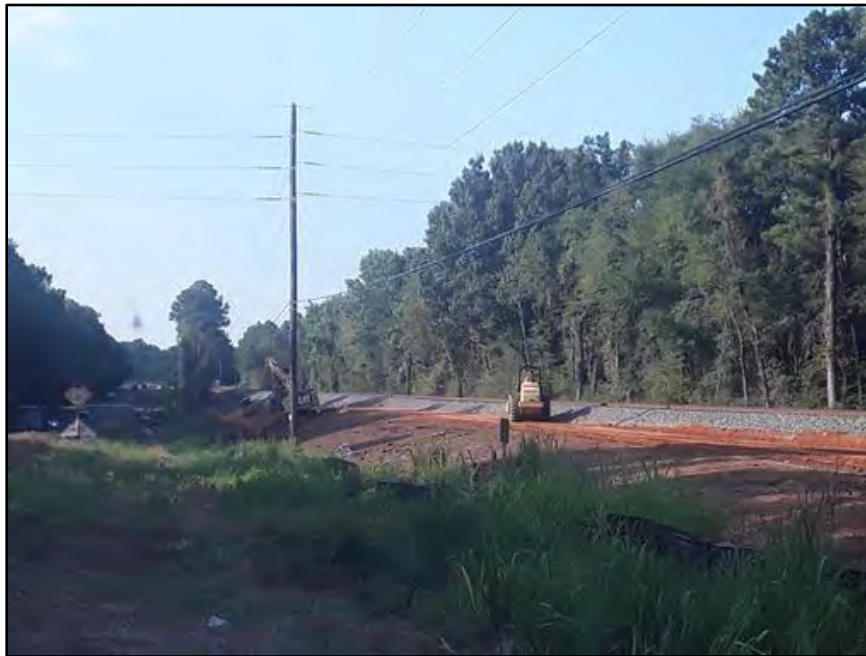
Figure 10. Continued excavation of borrow pit; view facing southeast. (Photograph by H. Moore August 3, 2023.)
