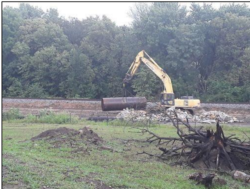
Figure 12. Iowa Trenchless hauling pipe to the bore pit; view facing east. (Photograph by S. Peterson 8/2/23.)
