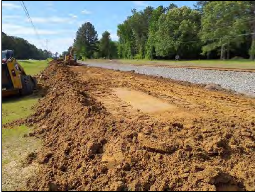
Figure 1. Initial topsoil clearance by a bulldozer; view facing southwest. (Photograph by H. MacIsaac April 24, 2023.)
