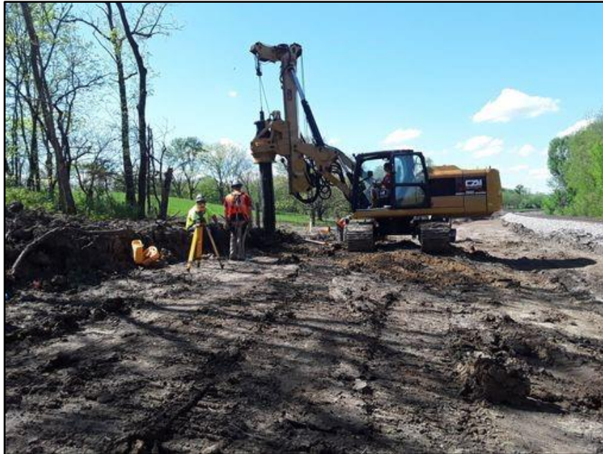
Figure 3. Foundation crew drilling holes to set H-beams for the foundation walls; view facing north. (Photograph by S. Peterson 5/13/23.)
