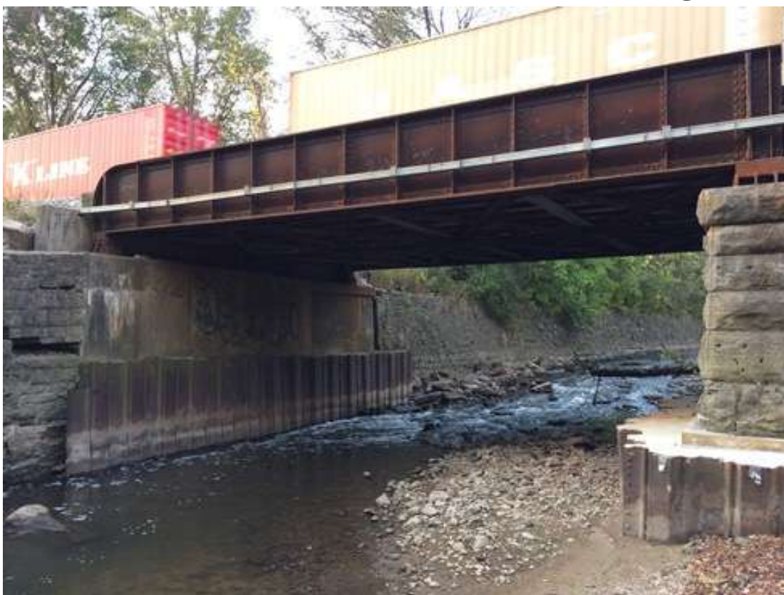
Photo 1 – Looking southeast at Abutment 1 of BR 88.74.
