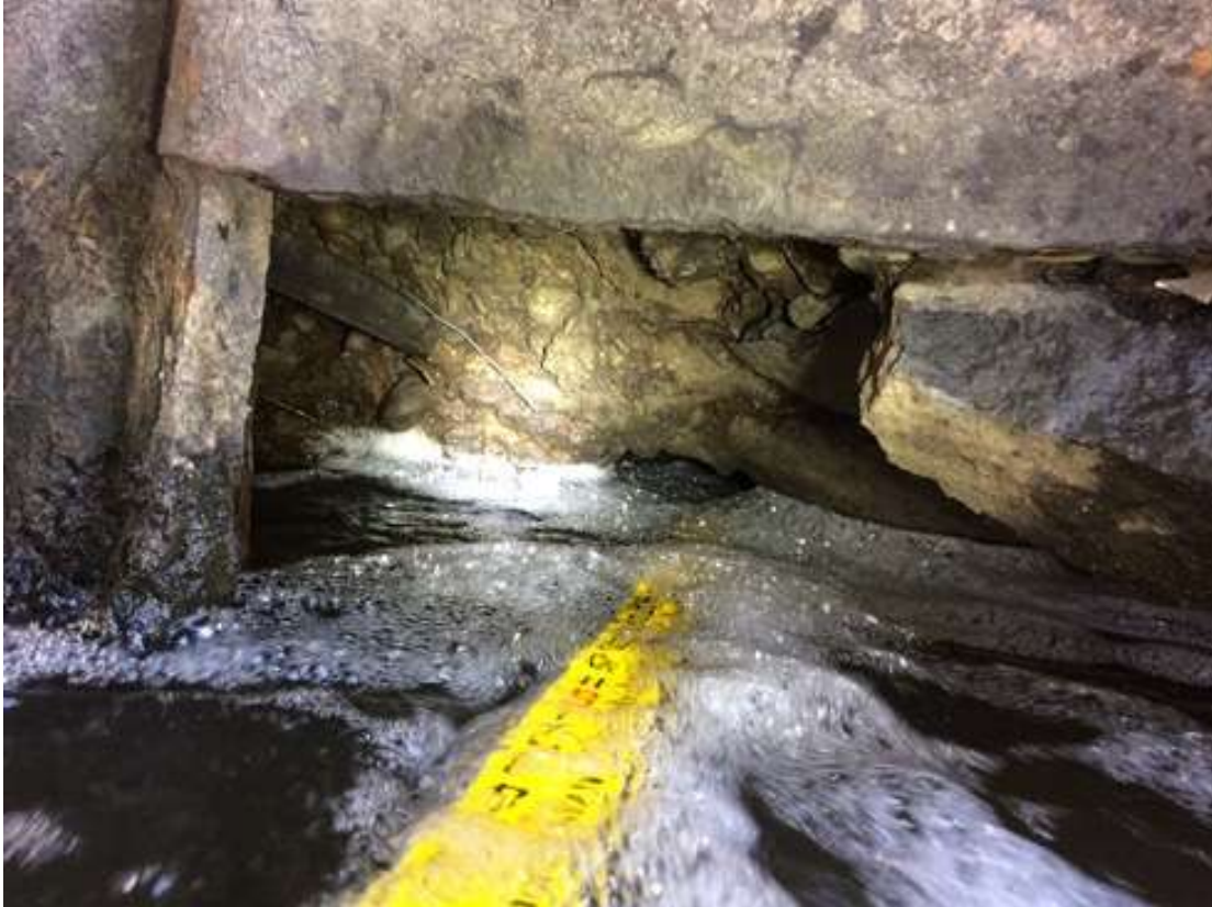
Photo 4 – Looking below the bottom of the sheet piling and into the void beneath the footing of Abutment 1.
