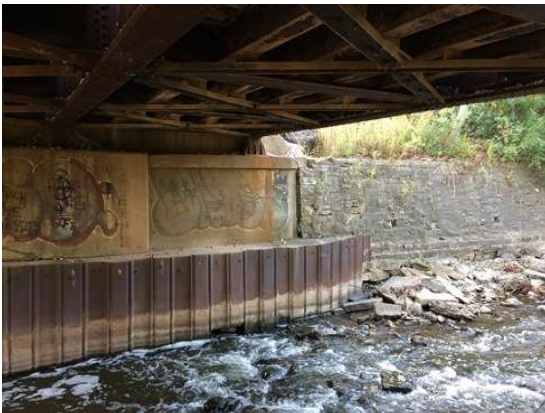
Photo 2 – Looking southeast at Abutment 1 of BR 88.74.
