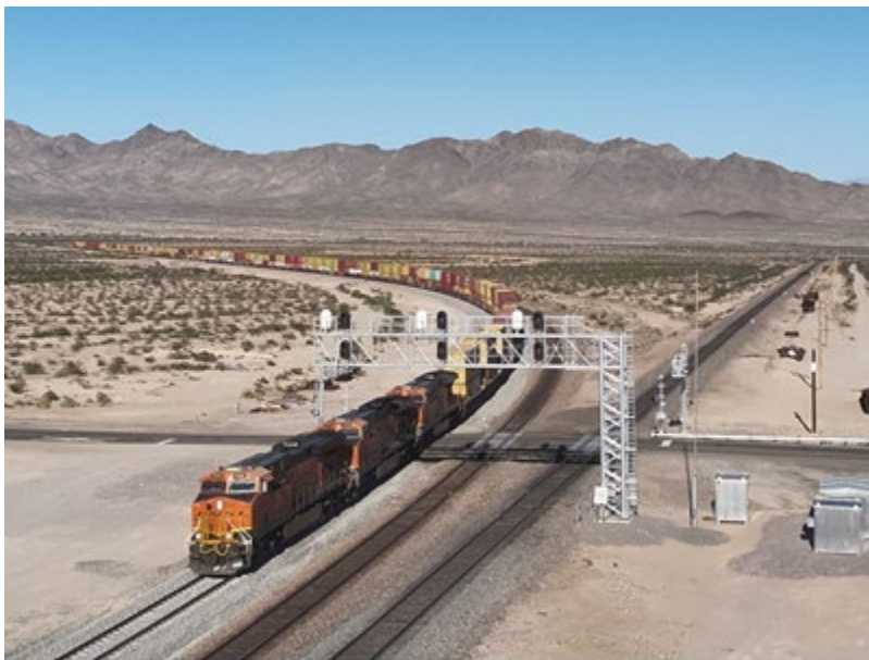
The first BNSF train traversing the newest triple-track section of the Needles Subdivision in September.
