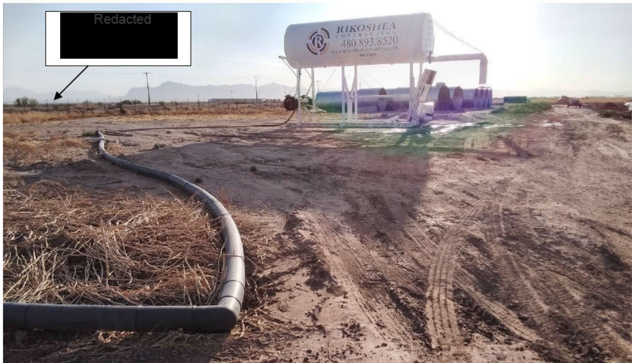
Damage Area 3. Post-disturbance in August 2023 [Redacted] along the proposed PIRATE alignment showing grading [Redacted] Pipes and a water tank have been placed within UP's right-of-way. View is to east-northeast.
