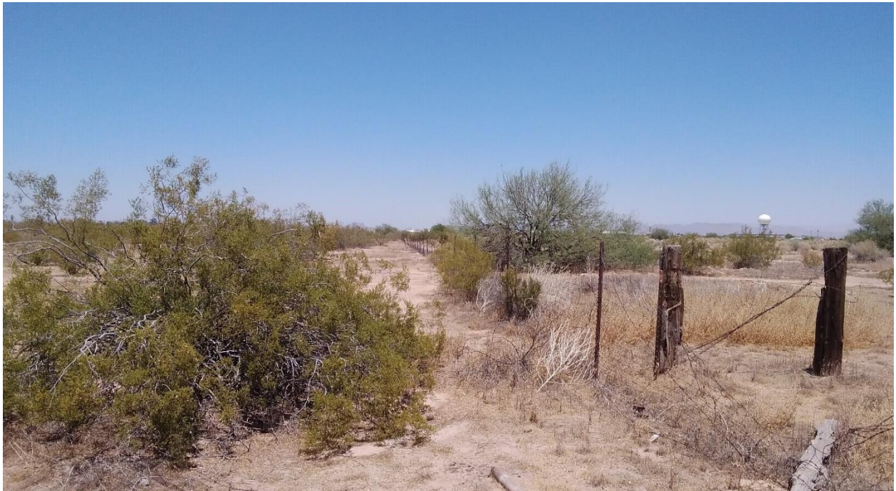
Damage Area 4. Pre-disturbance in May 2022. [Redacted] view to north. Overview of existing fence partially removed by Clayco, the general contractor for the adjacent Pecos Pacific development.
