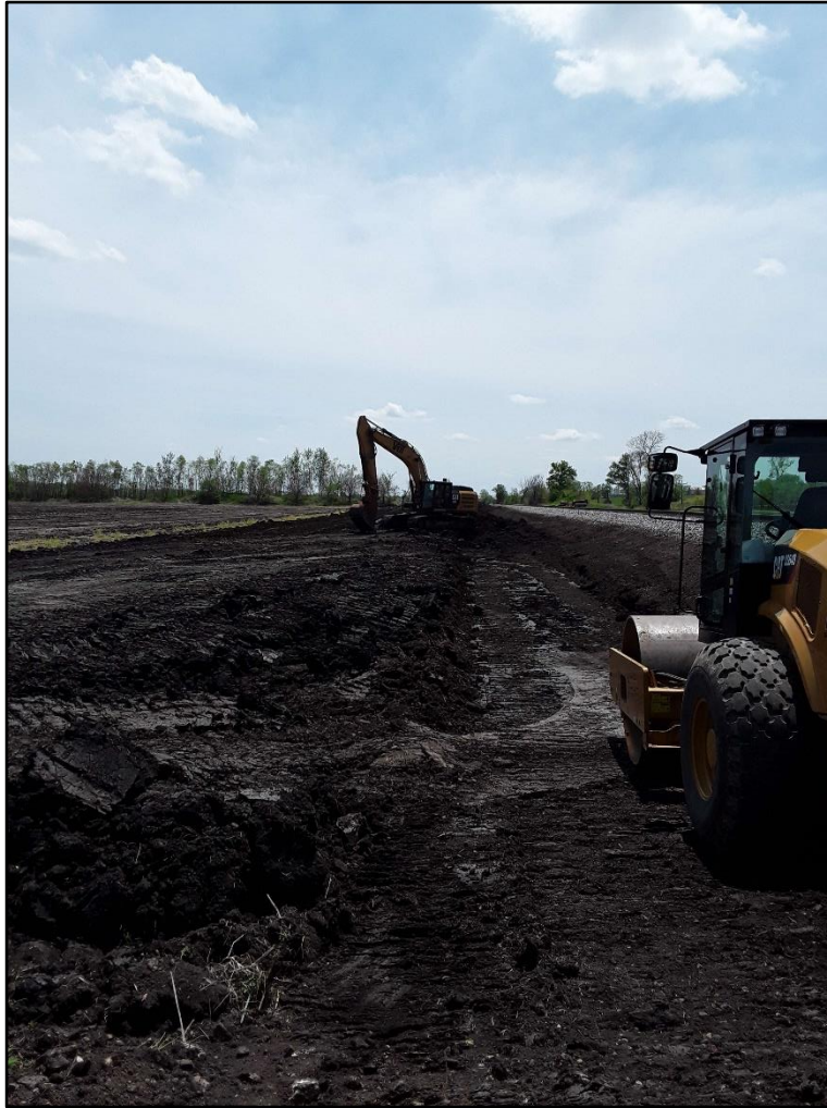
Figure 2. Image shows right-of-way clearance using trackhoe in preparation for the arrival of gravel to be laid down; view facing south (Photograph by J. Cropper May 10, 2023).
