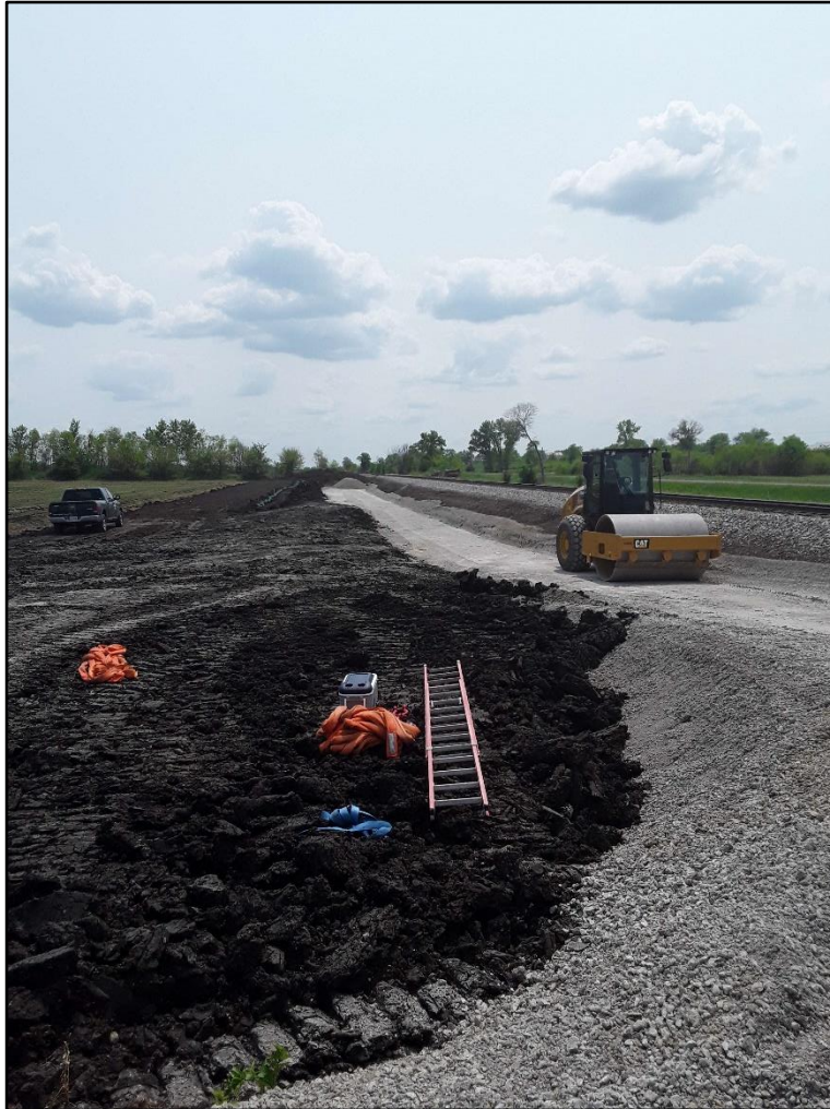
Figure 4. Image shows cleared right-of-way after gravel has been laid down, with roller smoothing the gravel path; view facing south (Photograph by J. Cropper May 17, 2023).
