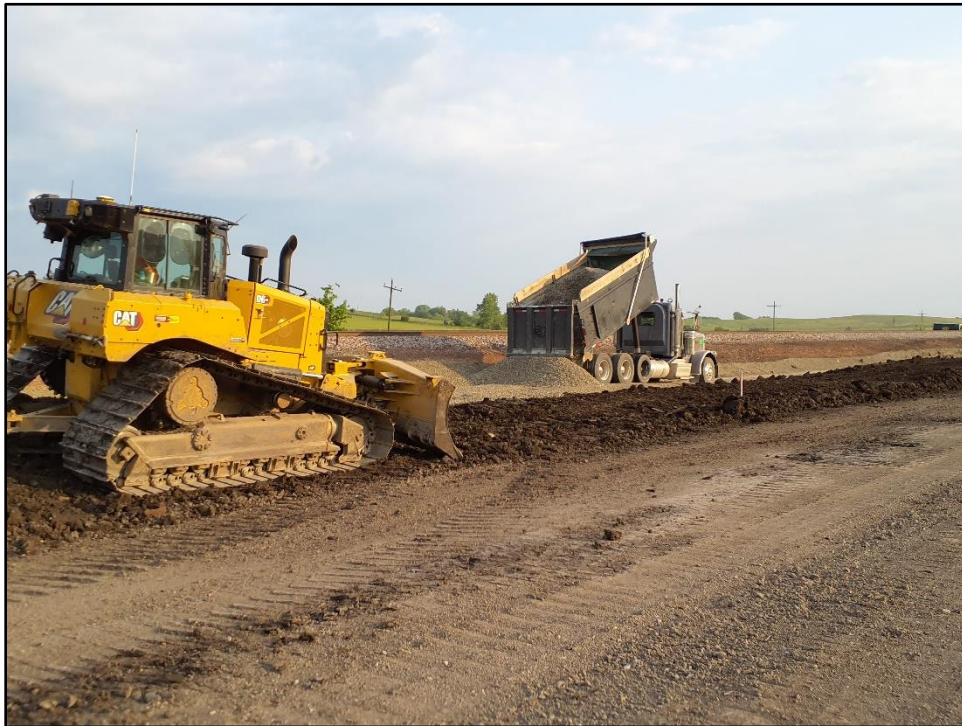
Figure 6. Image shows truck dumping rocks for bulldozer to flatten scatter on fill embankment; view facing northwest (Photograph by R. Campbell May 25, 2023).
