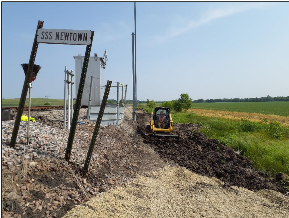
Figure 12. Image shows cutting and grading on the eastern side of the railroad track; view facing north (Photograph by R. Campbell June 9, 2023).
