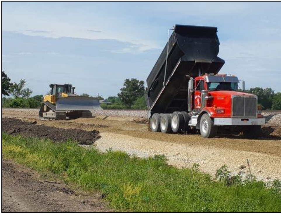
Figure 7. Image shows truck dumping rocks for bulldozer to flatten scatter on fill embankment; view facing southwest (Photograph by R. Campbell May 31, 2023).
