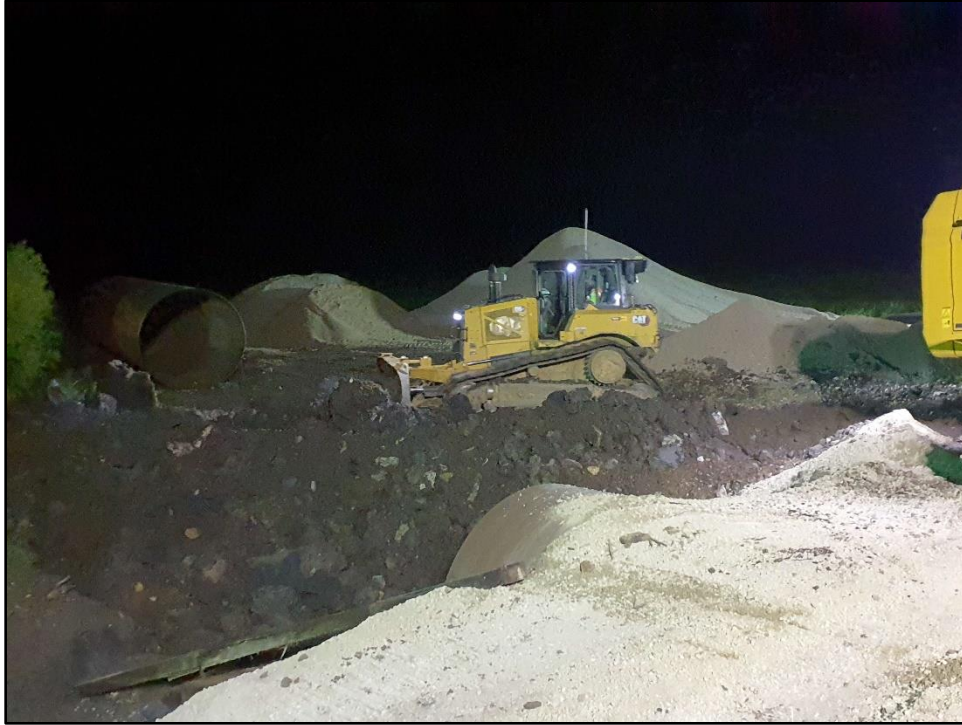
Figure 13. Image shows bulldozer pushing excavated soils from nighttime culvert installation into a nearby pile; view facing east. The pile was visually and manually inspected post excavation for any cultural resources, though none were found (Photograph by R. Campbell June 13, 2023).
