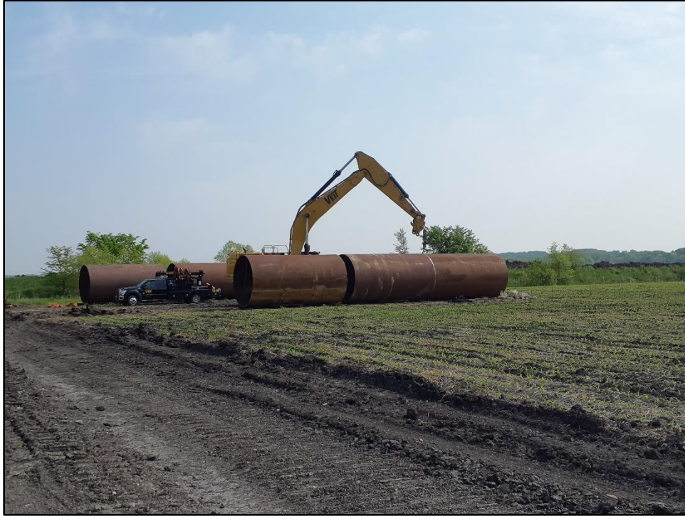
Figure 5. Image shows welding of culvert sections to replace wooden bridge; view facing northeast (Photograph by R. Campbell May 22, 2023).
