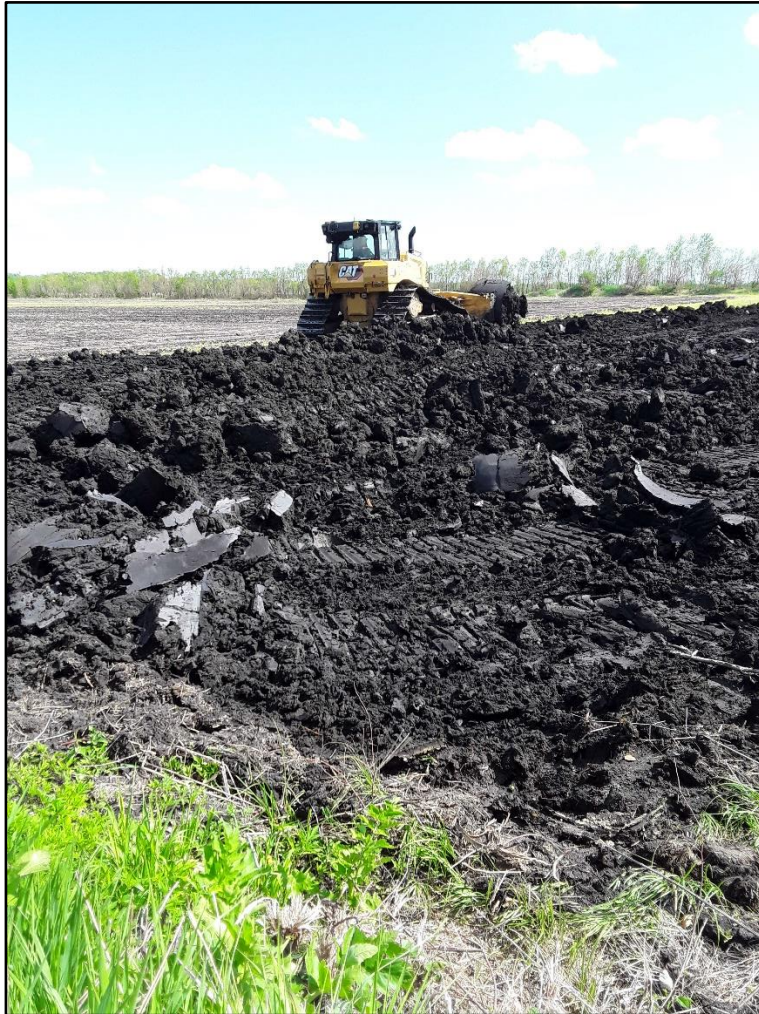
Figure 1. Image shows initial right-of-way clearance by bulldozer; view facing southeast (Photograph by J. Cropper May 8, 2023).
