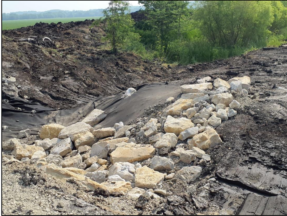
Figure 15. Image shows the large rocks being put down by the trackhoes to cover padding and create a stable ground surface around the culvert entrance; view facing northeast (Photograph by R. Campbell June 16, 2023).
