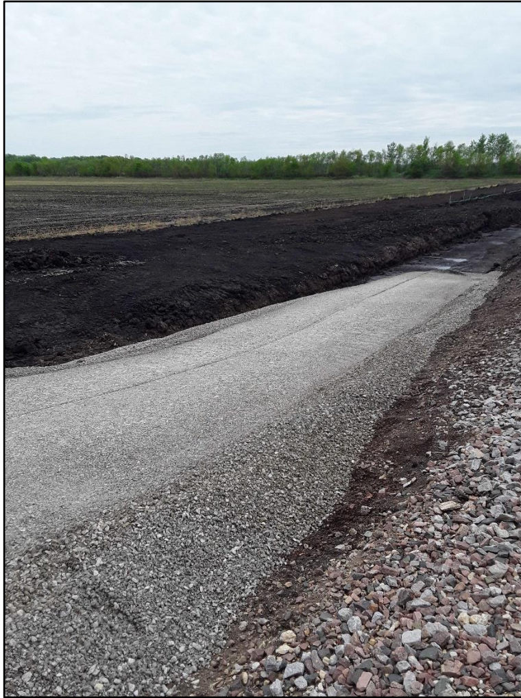
Figure 3. Image shows cleared right-of-way after gravel has been laid down; view facing southeast (Photograph by J. Cropper May 16, 2023).
