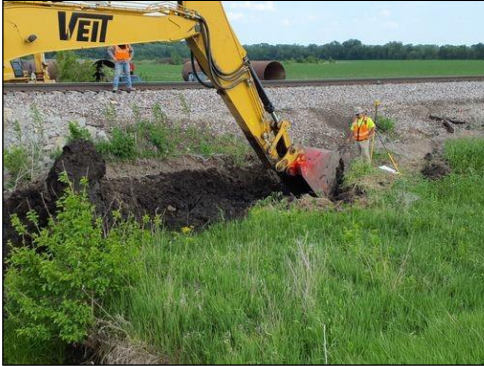
Figure 8. Temporary excavation/disturbed area was refilled with excavated topsoil; view facing southeast. This action was performed to test the soils for the upcoming culvert installations (Photograph by R. Campbell May 30, 2023).
