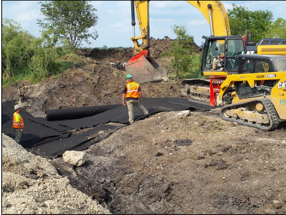
Figure 14. Image shows construction workers laying down pads to lay fill upon and create a stable surface as part of cleanup from culvert installation; view facing northeast (Photograph by R. Campbell June 15, 2023).
