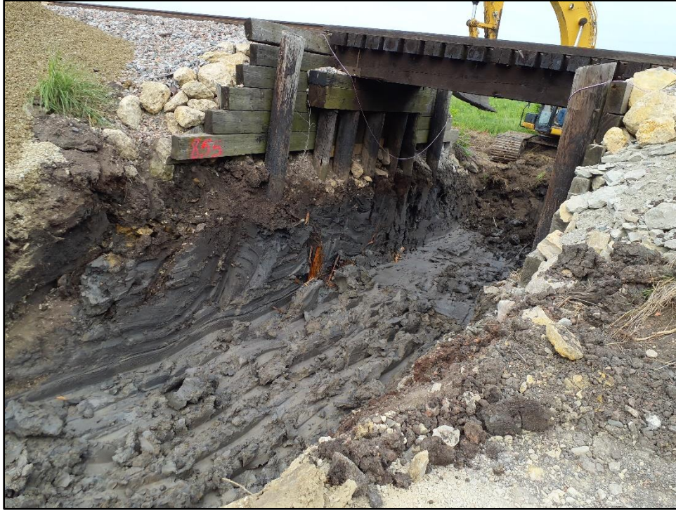
Figure 10. Image shows trench dug by trackhoe for culvert installation; view facing west. Soils were 10 YR dark grey alluvial clay with large amounts of wood and rocks included (Photograph by R. Campbell June 7, 2023).
