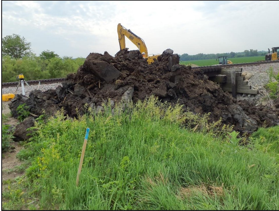
Figure 11. Image shows one of two soil piles made from excavated soils under wooden bridge; view facing east. Both piles were visually and manually inspected post excavation for any cultural resources, though none were found (Photograph by R. Campbell June 7, 2023).
