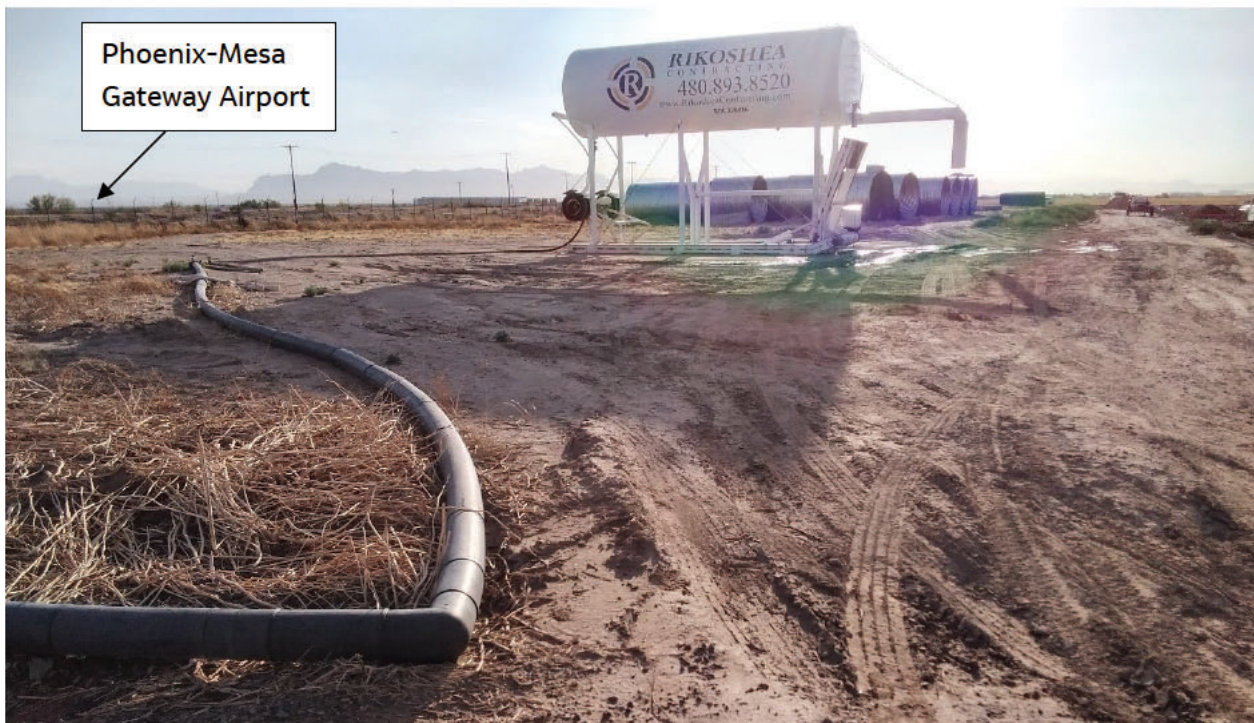
Phoenix-Mesa Gateway Airport Damage Area 3, post-disturbance, [REDACTED] [REDACTED] showing grading [REDACTED]. Pipes and a water tank have been placed within UP's right-of-way. View is to east-northeast.
