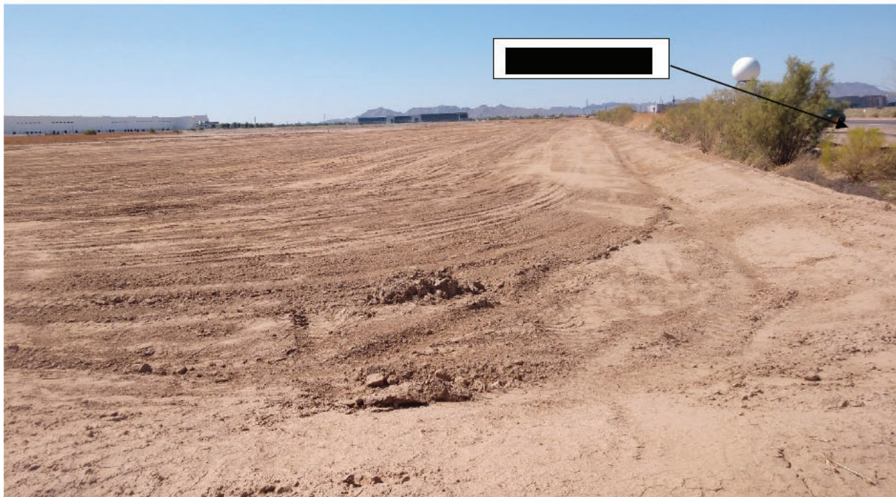
Damage Area 2, post-disturbance, [REDACTED] [REDACTED] showing retention basin cut, view south, August 2023.
