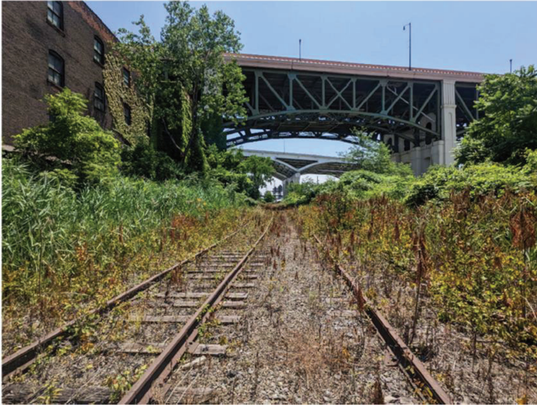
BBJ 74.00-0 , Carnegie Avenue Overhead Bridge. Reverse Track View, from high milepost facing low milepost
