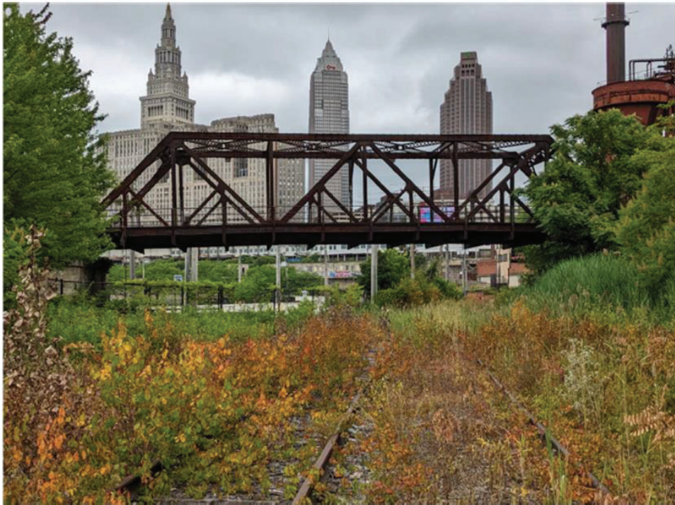
BJB 74.25, Stones Levee Overhead Bridge in Cleveland, Ohio – Track View
