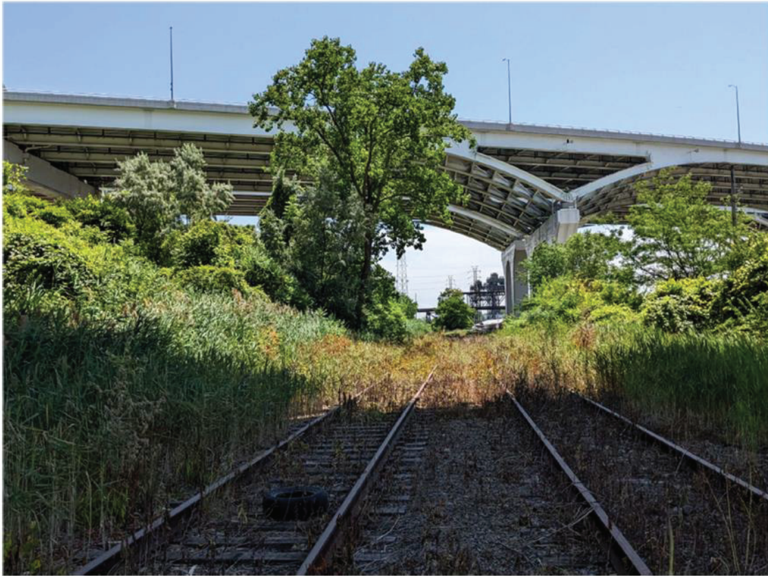
BJB 73.80-0 , I-90 Overhead Bridge. Reverse Track View, From high milepost facing low milepost.
