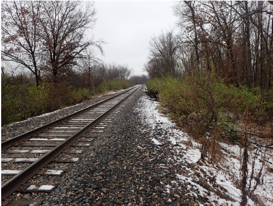
Photograph 12: Overview of the planned Mexico Capital Improvement ROW; Camera facing east
