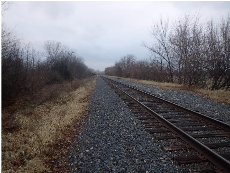
Photograph 8: Overview of the planned Harmony Capital Improvement ROW; Camera facing east
