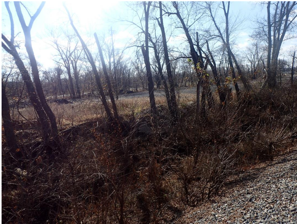
Photograph 4: Overview of planned Grain Valley Capital Improvement ROW showing adjacent ditch (foreground) and road (background); Camera facing south
