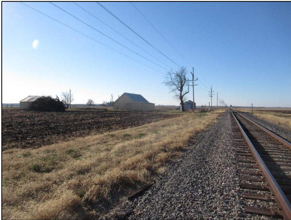
Photograph 3: Overview of the planned Roodhouse Capital Improvement ROW, camera facing south.
