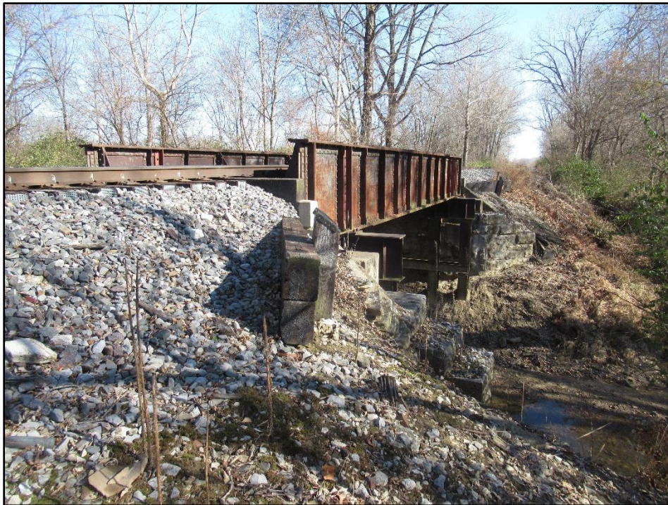
Photograph 5: Overview of the planned Pleasant Hill Capital Improvement ROW, camera facing northeast. Bridge carries the line over unnamed tributary of Bay Creek.
