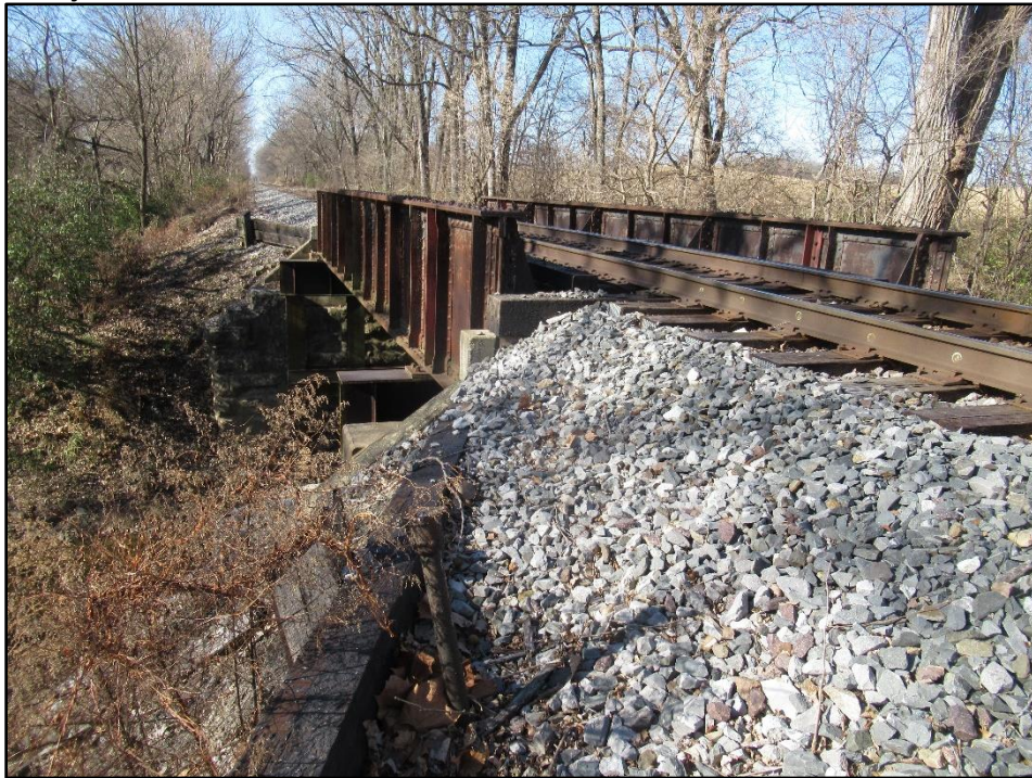
Photograph 6: Overview of the planned Pleasant Hill Capital Improvement ROW, camera facing north. Bridge spans unnamed tributary of Bay Creek.
