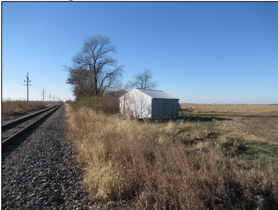
Photograph 4: Overview of the planned Roodhouse Capital Improvement ROW, camera facing southwest. Machine shed in centerground is of recent construction.
