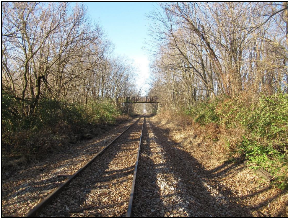
Photograph 1: Overview of the planned Cockrell Capital Improvement ROW, facing west.
