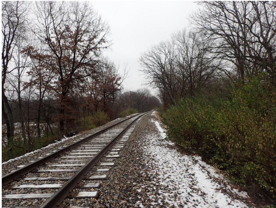
Photograph 10: Overview of the planned Mexico Capital Improvement ROW; Camera facing east
