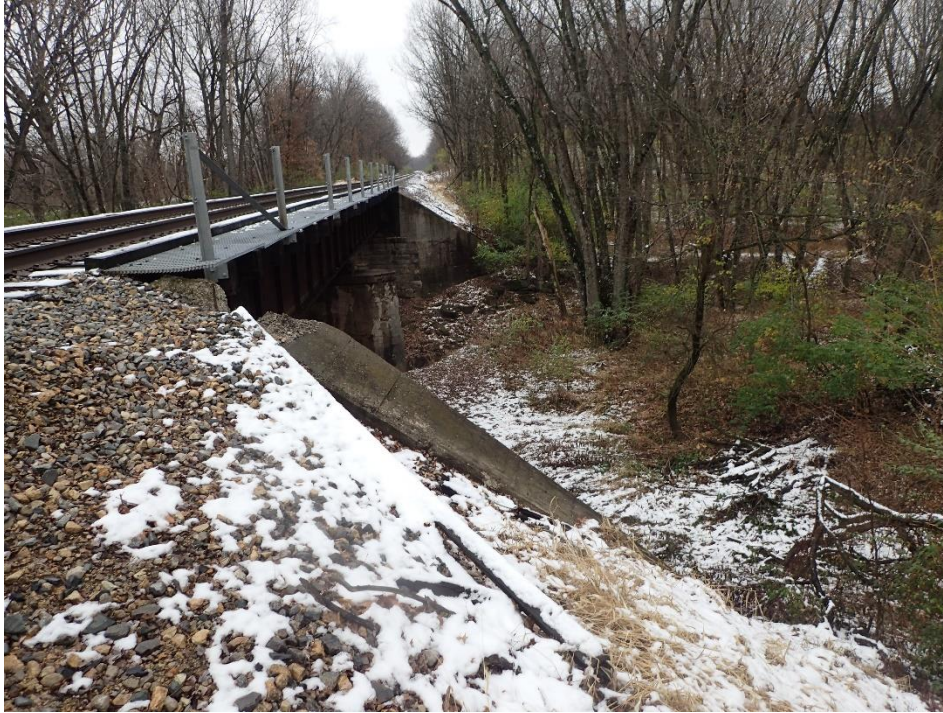
Photograph 11: Overview of the planned Mexico Capital Improvement ROW showing fill and bridge structure over Davis Creek; Camera facing east
