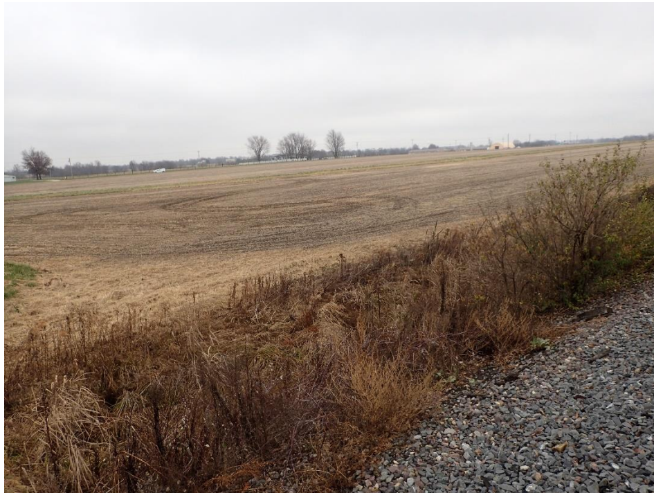
Photograph 16: Overview of the planned Bowling Green Capital Improvement ROW illustrating slope and elevated railroad grade; Camera facing north
