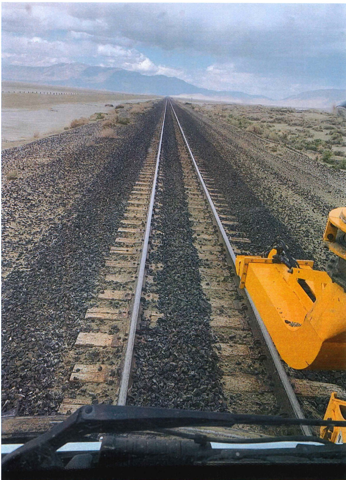
Figure 1- Prior to Track Raise
