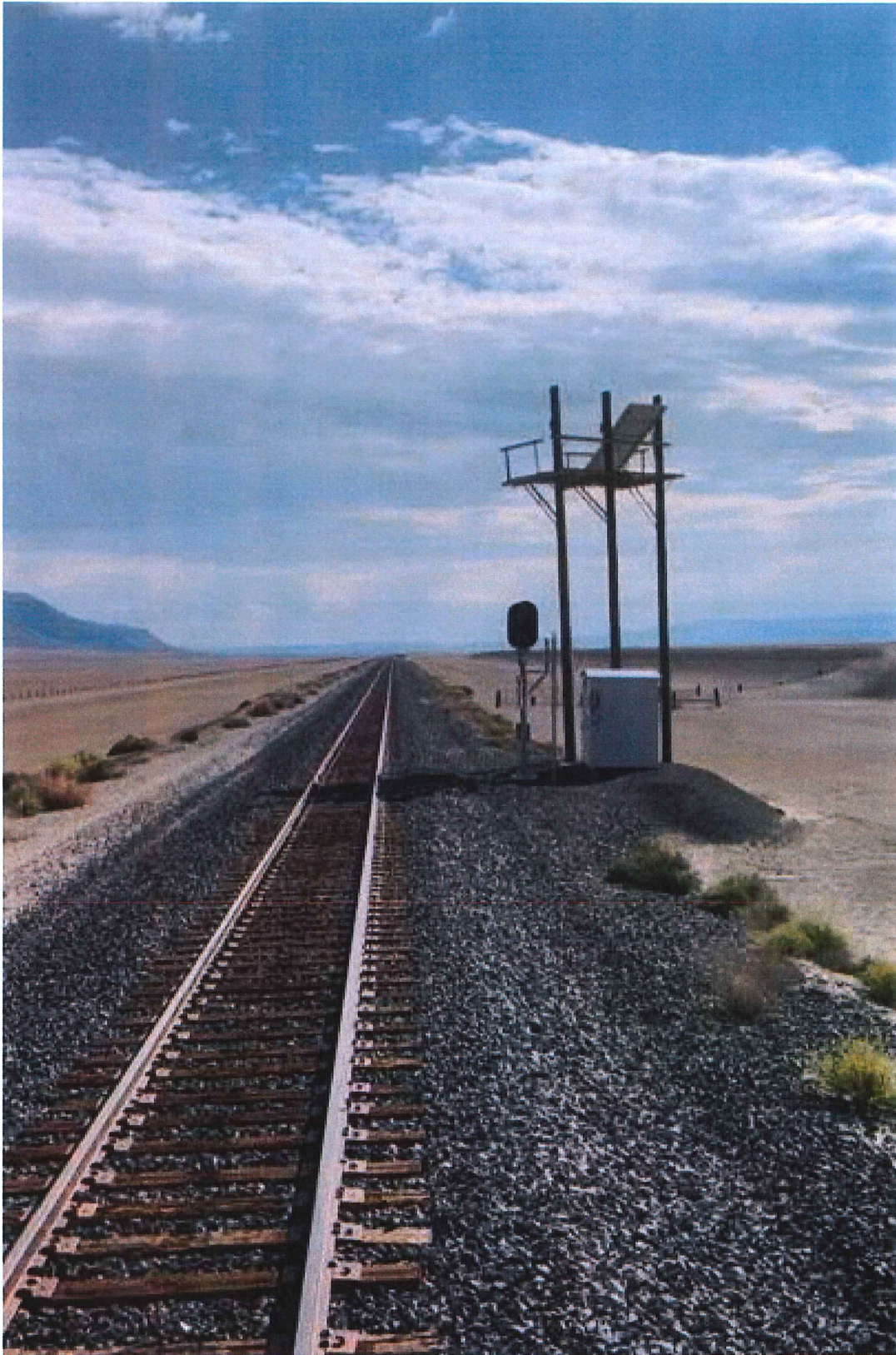
Figure 4 - Final Track Raise
