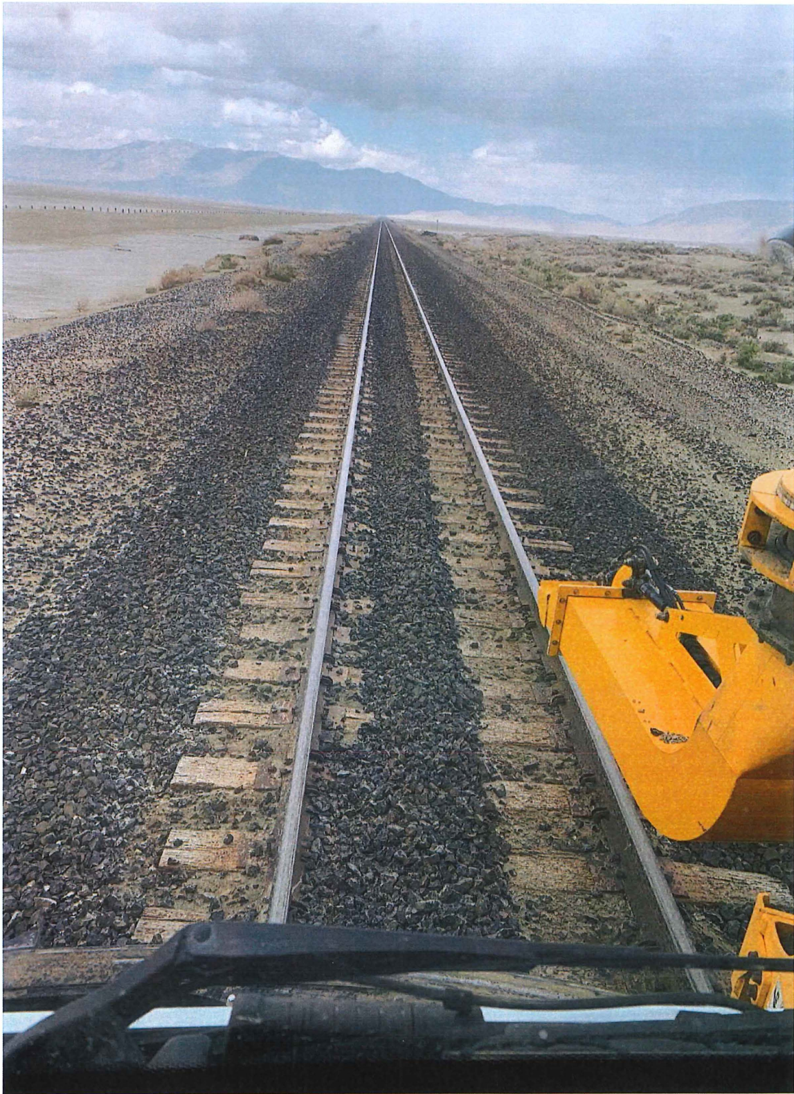
Figure 1- Prior to Track Raise
