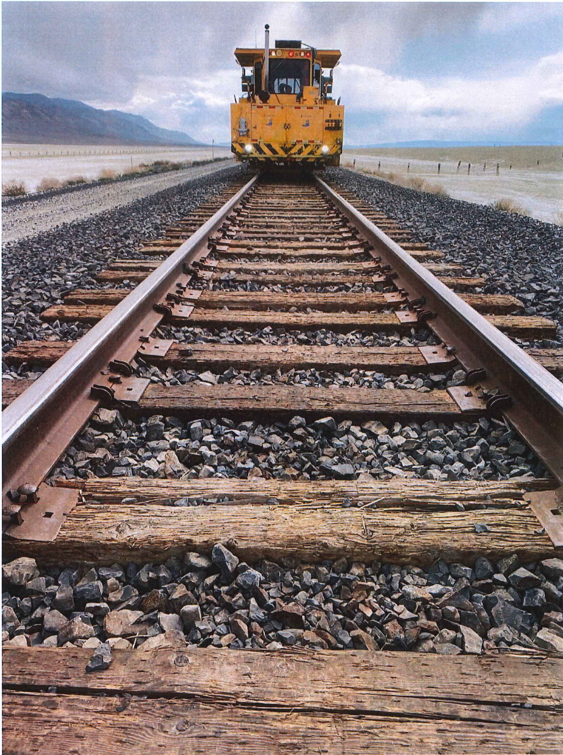
Figure 3 – Final Track Raise
