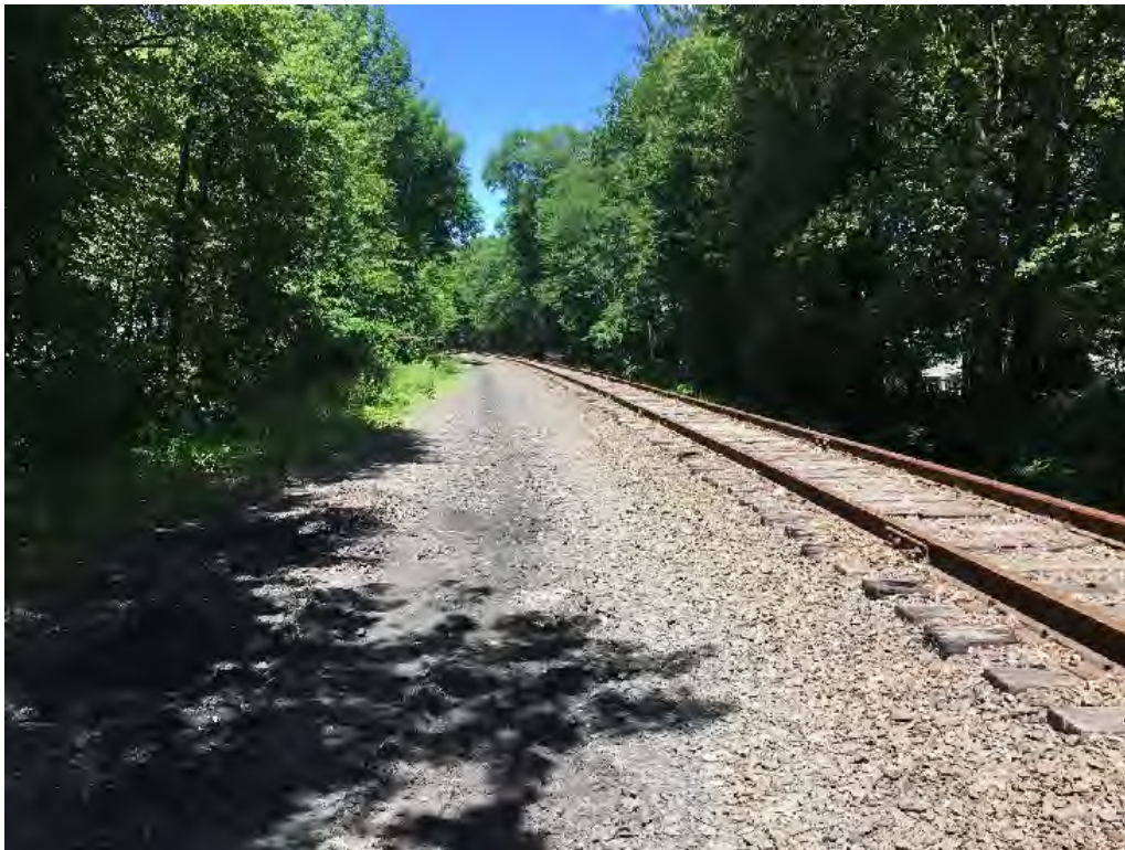
Photo 16. View of the existing railroad as it extends north passed the Trailhead 5 APE on the left.
