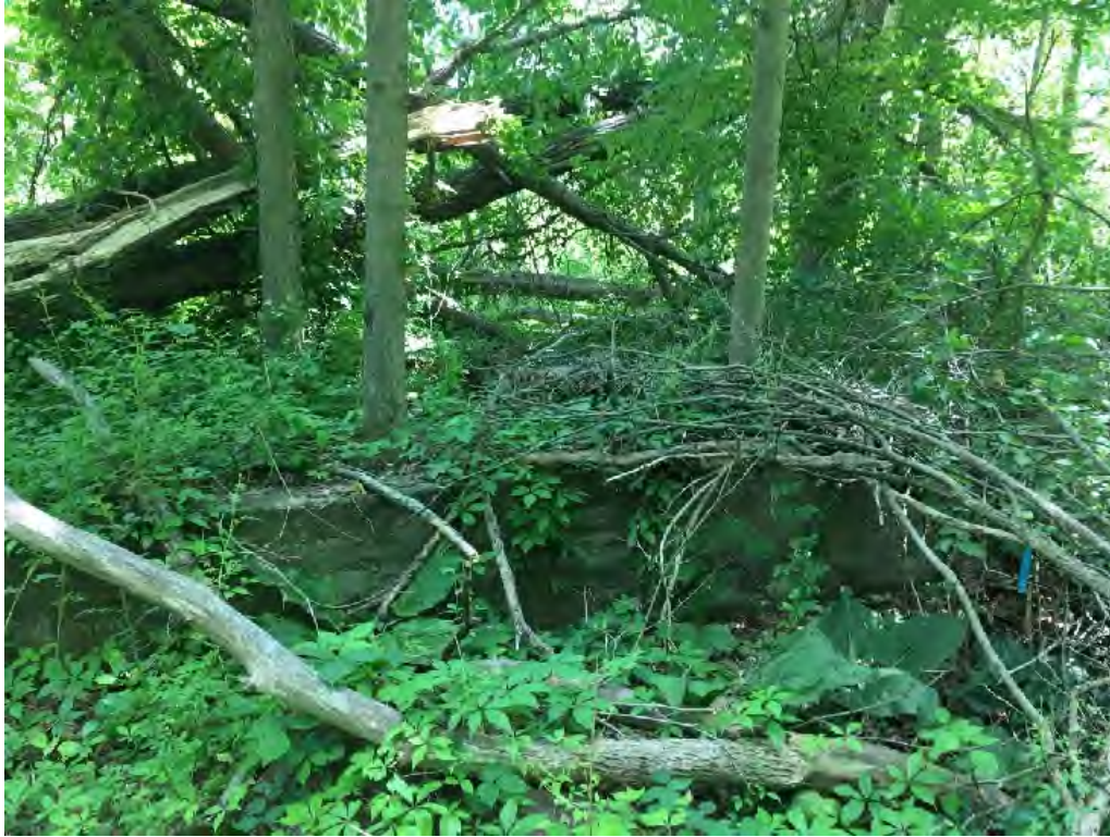
Photo 15. View of the west wall of a concrete foundation that for a smaller building within the depot.
