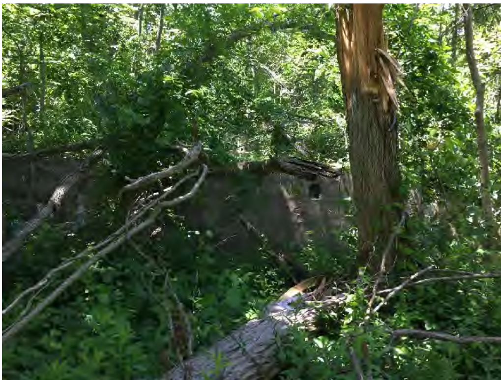
Photo 14. View of the east wall of a large concrete foundation, likely of the old depot building that was located within Trailhead 4.
