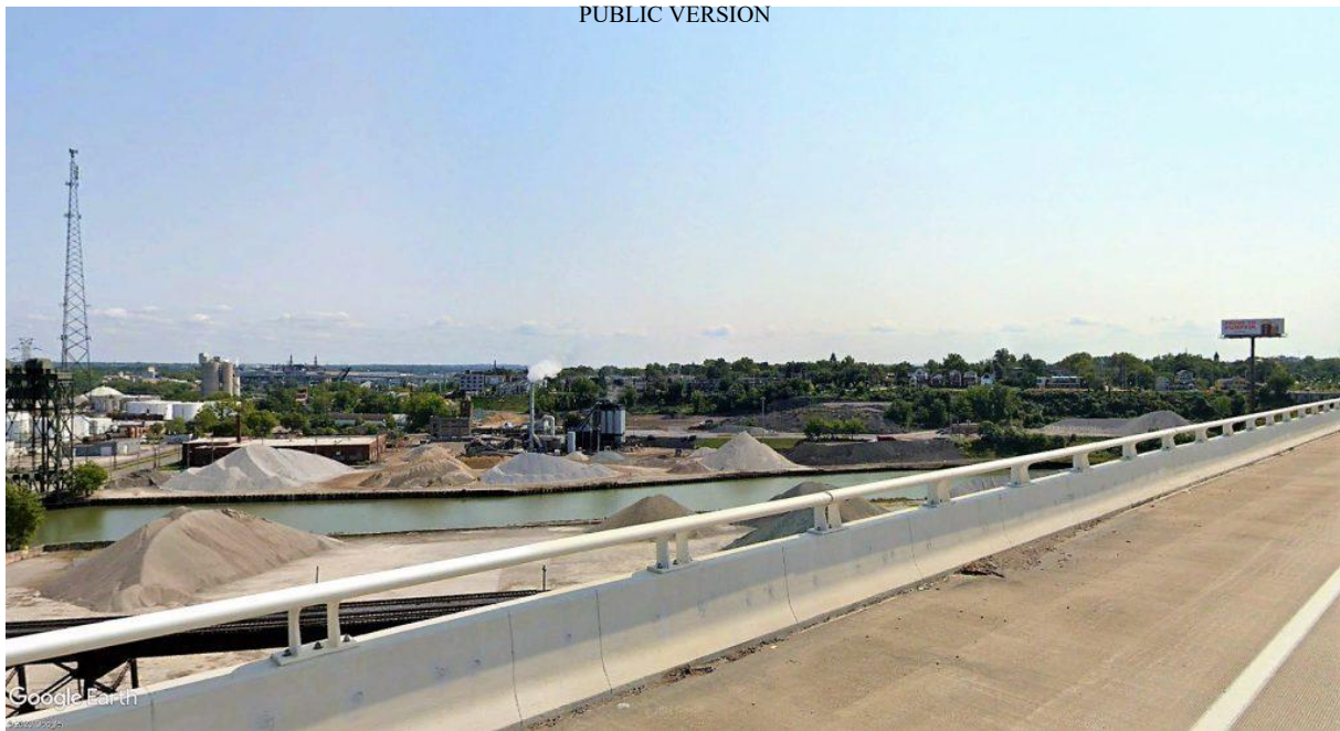
The Tremont hillside redevelopment site is visible from Interstate 90's George Voinovich Bridges. The site extends from the West 3rd Street lift bridge at left to the elevated billboard sign at right, just above the Cuyahoga River and the piles of aggregates on Lafarge Corp.'s property (Google).
