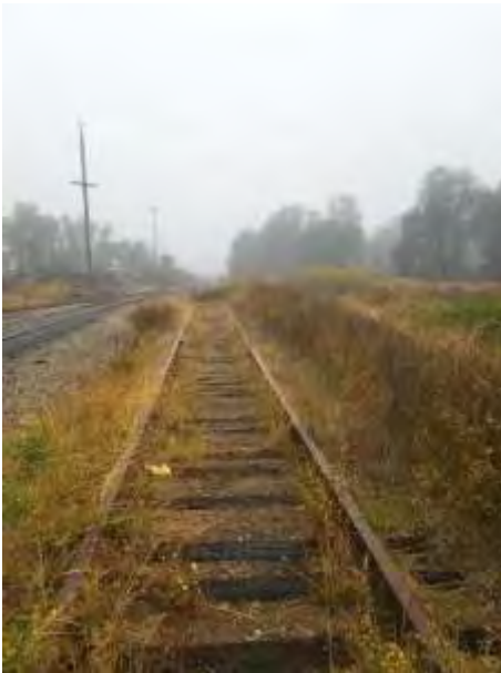
Milepost 139.8 still in Willits yard Vegetation: Poor Ties: Good Rail: 132lb. Good Condition
