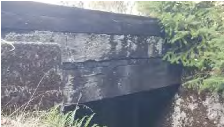
145.1 bridge 20 ft long concrete post in good condition, timbers, and cap in good condition
