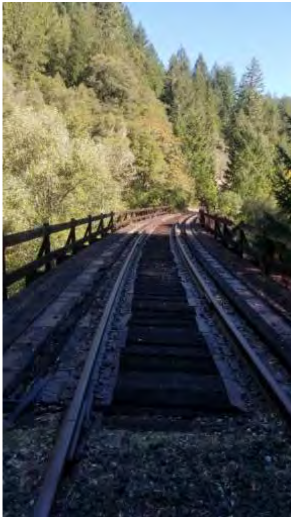
Bridge milepost 147.8 160 ft long, 131 lb rail in good condition. Deck ties are in good condition, metal girders are in good condition concrete pilings are in good condition.
