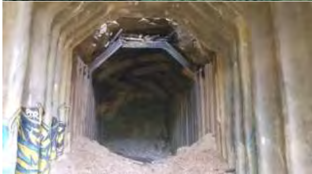
North end of the tunnel
