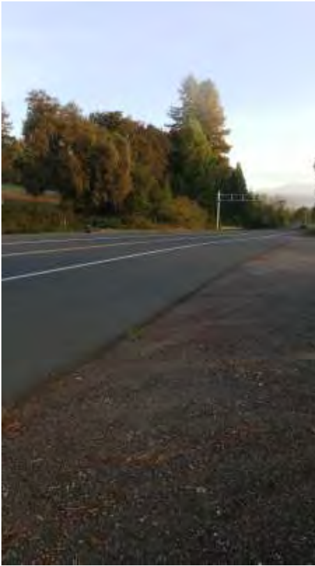
The crossing at highway 101 was completely removed
