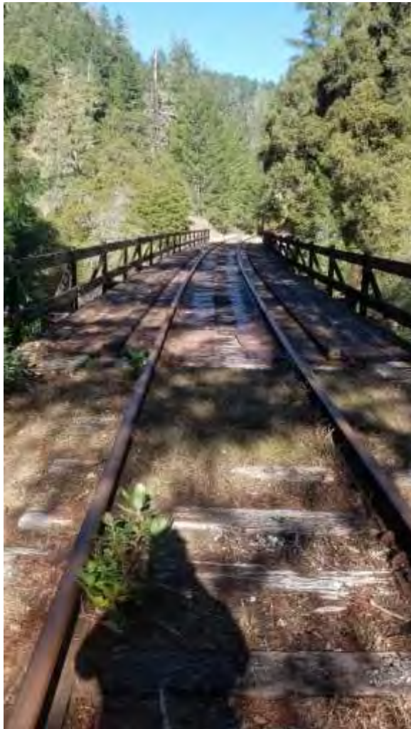
Bridge 147.1 deck ties good condition rail 131 lb and good condition the Metal girder is in good condition, concrete posts are in good condition
