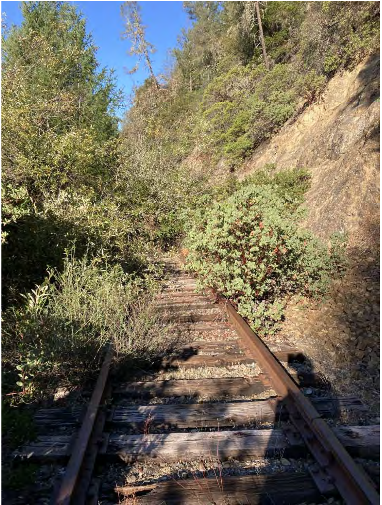
Milepost 150.3, 110 lb rail in good condition. The tie condition is good but would need joint ties for class 1
