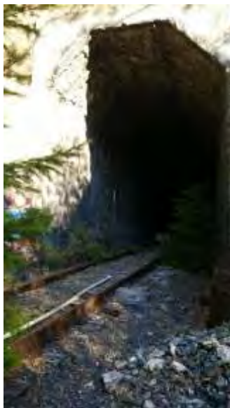
Milepost 148.5, vegetation condition extremely poor. 110 lb rail in good condition, tie condition covered.
