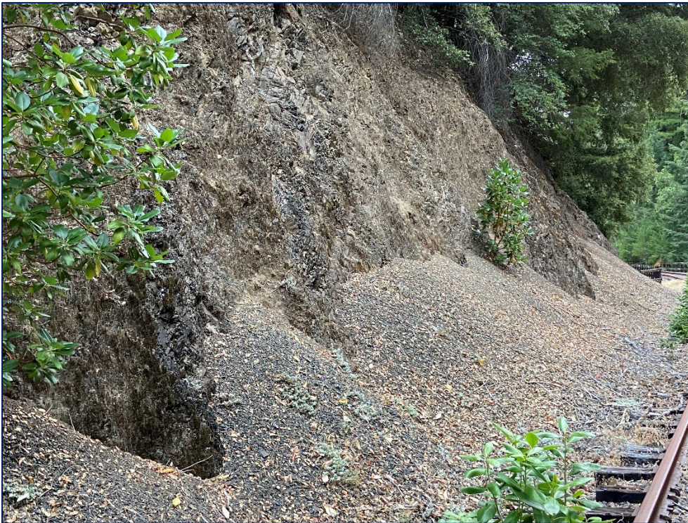
Exhibit 4-3 – Photo 65 – Fragments of highly fractured siltstone and mudstone raveling from rock slope at approx. MP 147.3
