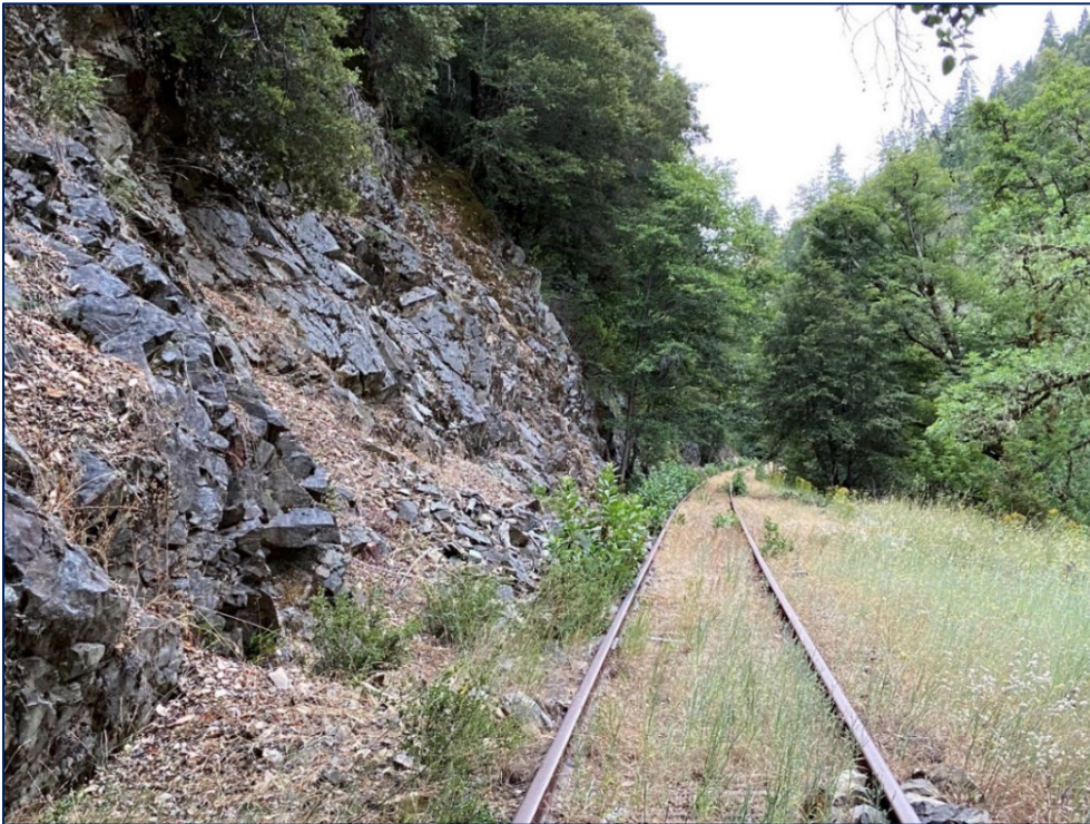
Exhibit 4-2 – Photo 60 – Blocky sandstone rock slope at approx. MP 147.5
