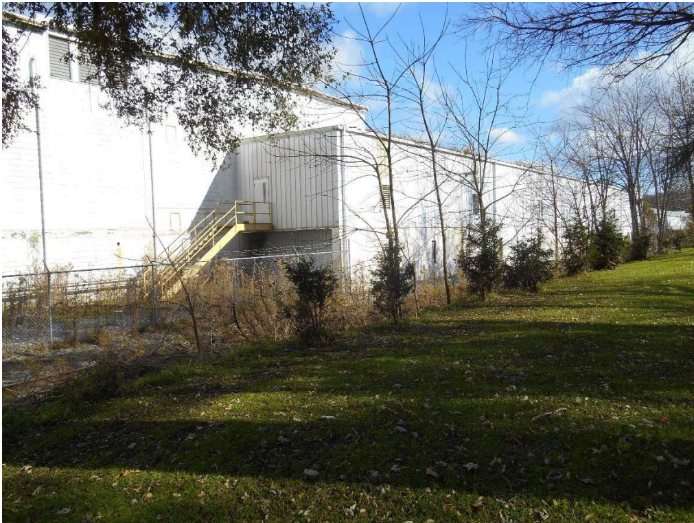
PHOTO 12: View of the Tyoga Container Company Distribution Building facing northeast.
