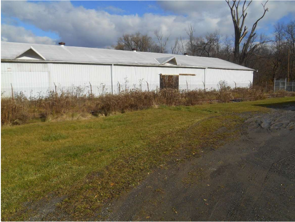
PHOTO 15: View of the Tyoga Container Company Distribution Building facing north.
