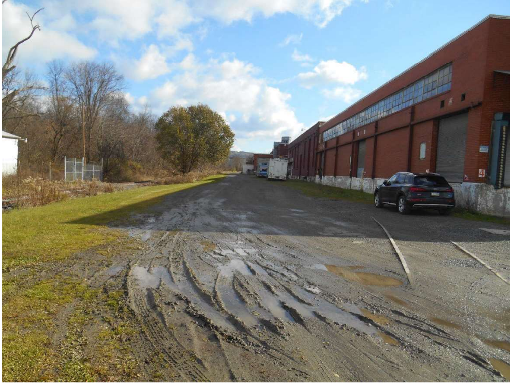
PHOTO 9: View of the Wellsboro Electric Company Building facing southeast.
