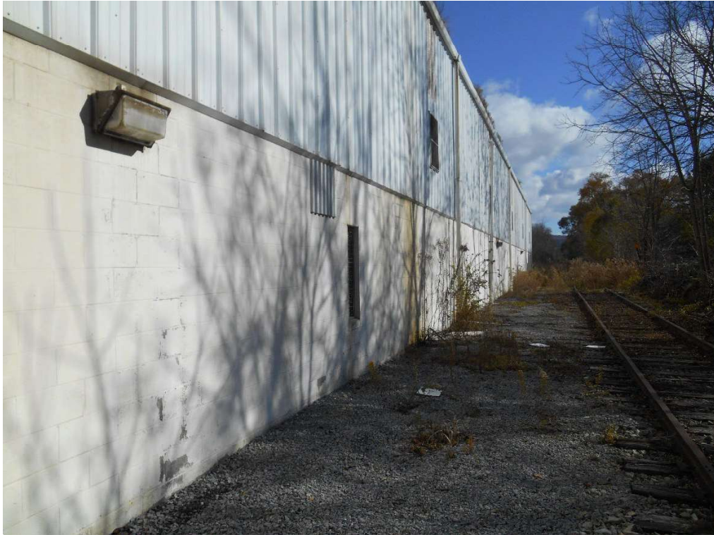
PHOTO 13: View of the Tyoga Container Company Distribution Building from rail line facing east.
