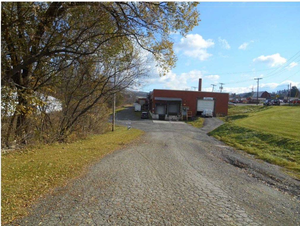
PHOTO 10: View of the Wellsboro Electric Company Building facing southeast.
