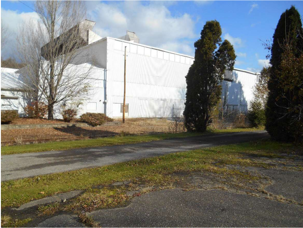
PHOTO 11: View of the Tyoga Container Company Distribution Building from rail line facing north.
