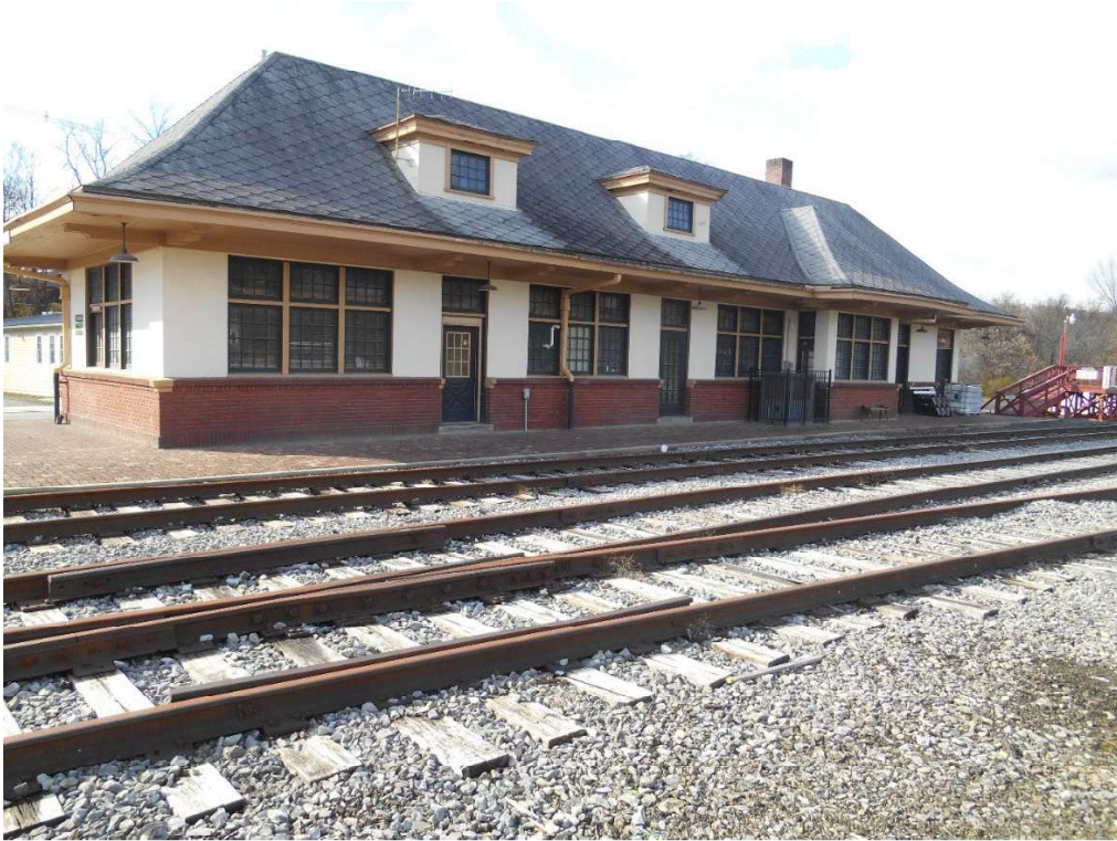
PHOTO 5: View of the Passenger Station from railroad tracks looking south.
