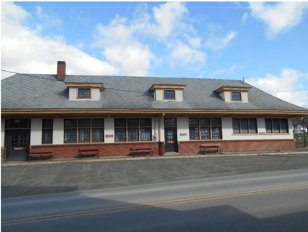
PHOTO 2: View of the Passenger Station from Charleston Street looking north.
