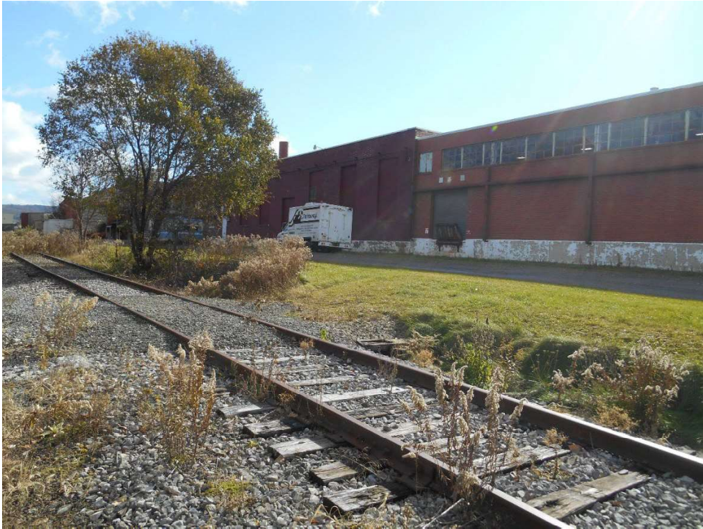
PHOTO 7: View of the Wellsboro Electric Company Building from the railroad tracks facing east.
