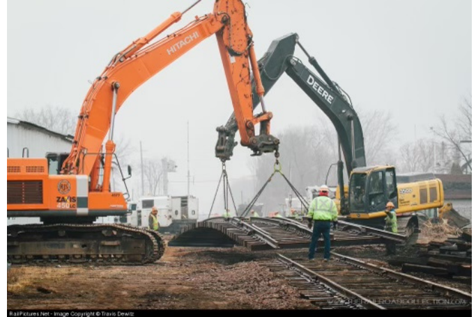
Top: CN Installing Switch South of Cameron Interchange December 1, 2012 2 Bottom: Location Photo was Taken Photo Credits Travis Dewitz
