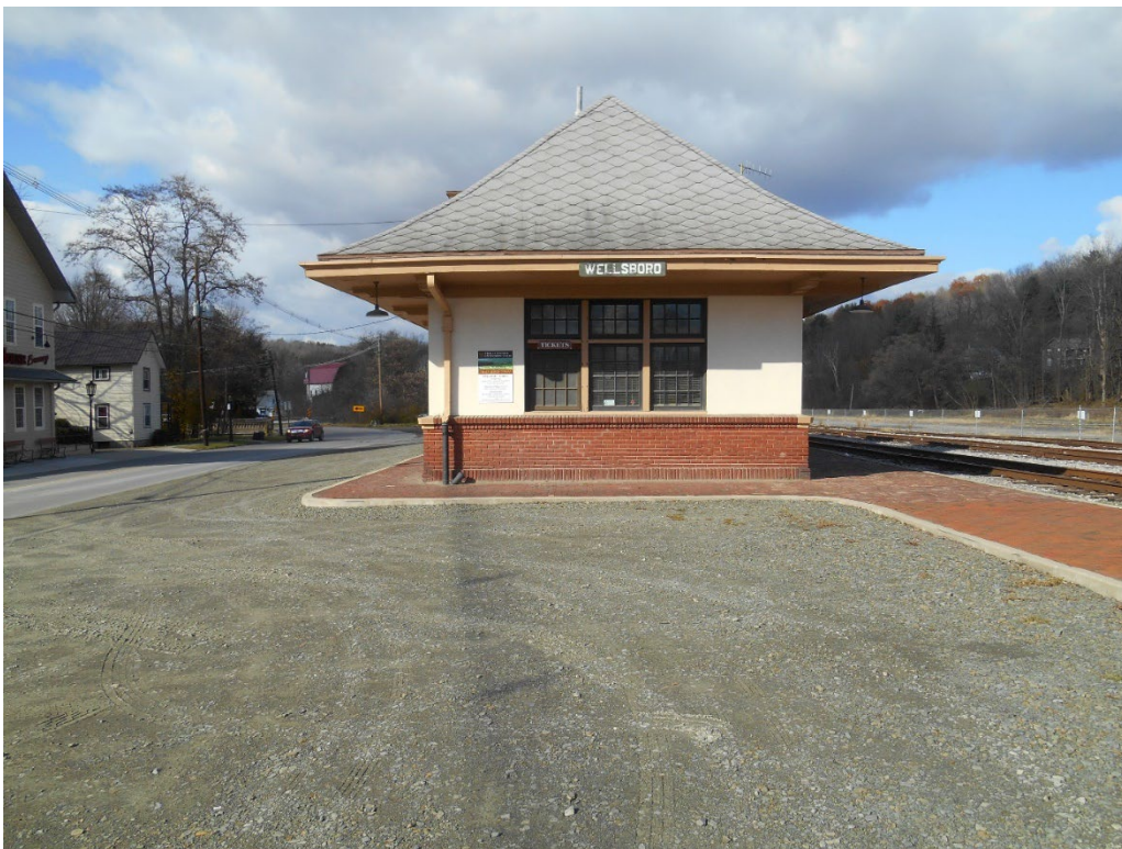
PHOTO 4: View of the Passenger Station from Charleston Street looking northwest.
