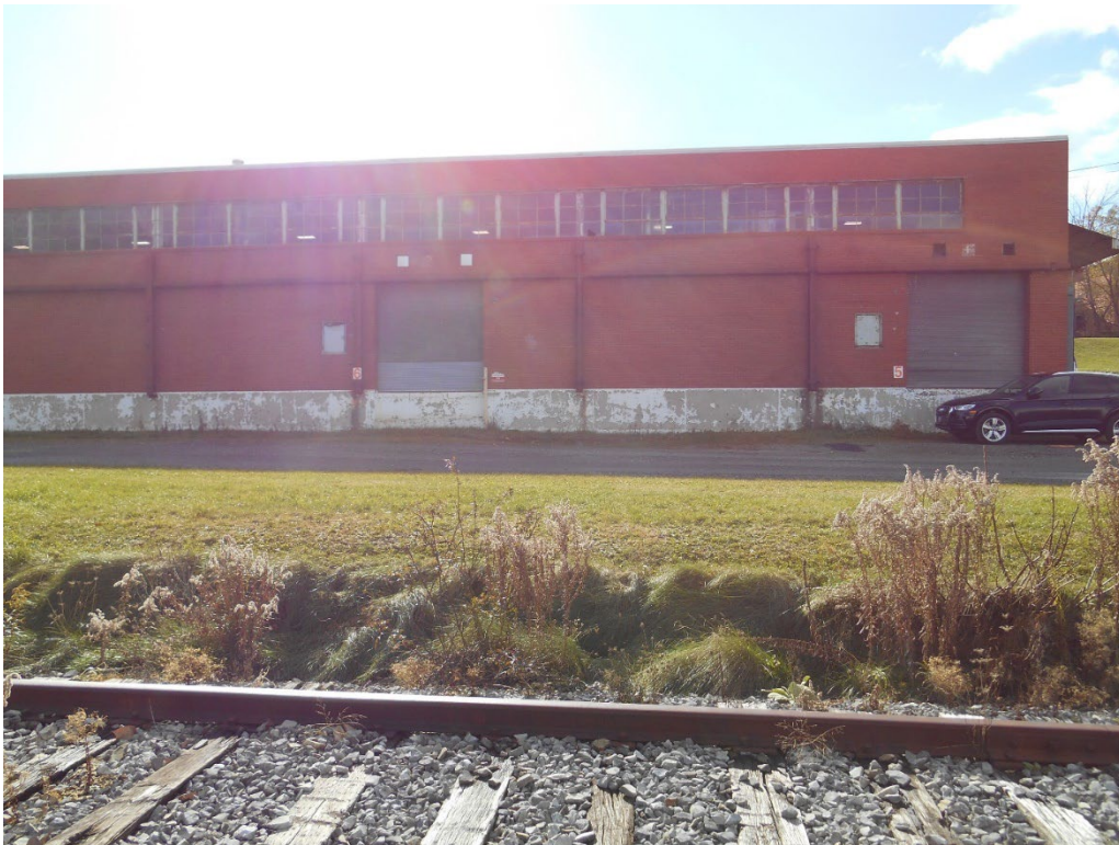
PHOTO 8: View of the Wellsboro Electric Company Building from the railroad tracks facing east.
