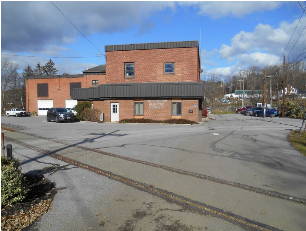
PHOTO 6: View of the Wellsboro Electric Company Building from the railroad tracks facing north.
