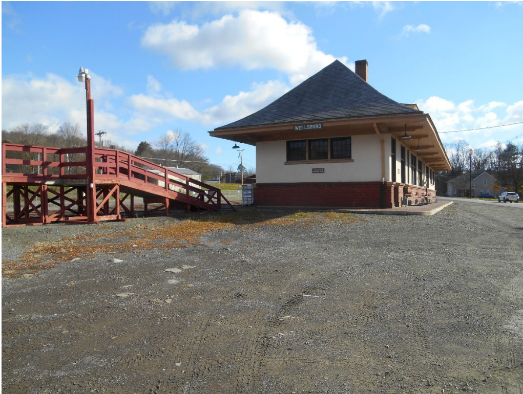
PHOTO 1: View of the Passenger Station from Charleston Street looking southeast.
