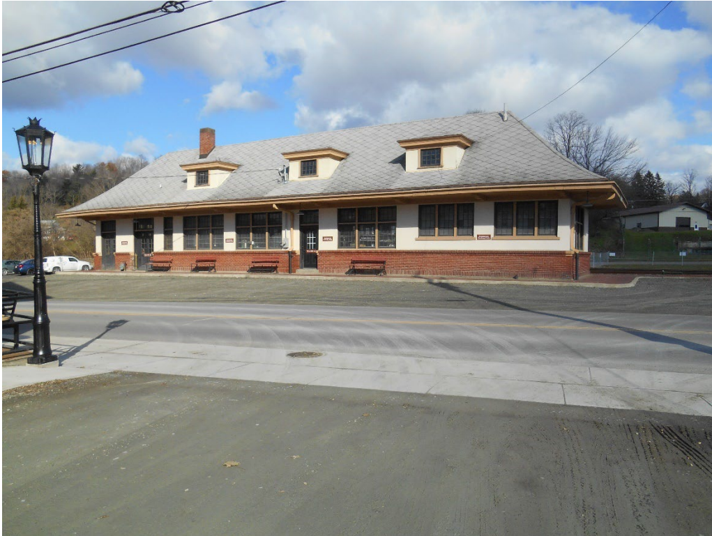
PHOTO 3: View of the Passenger Station from Charleston Street looking north.
