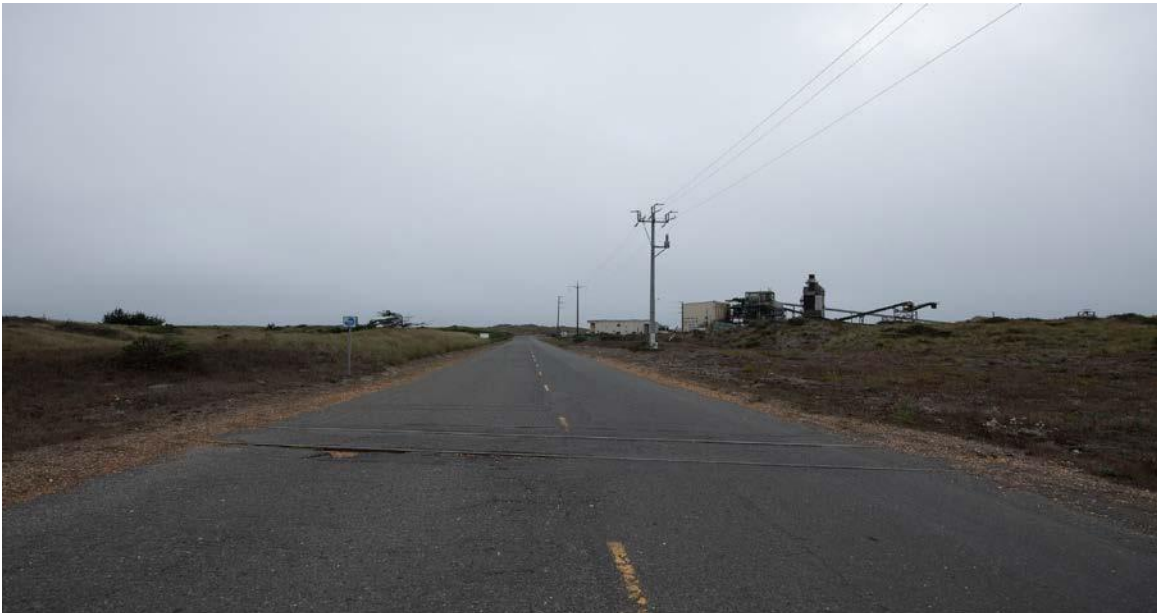
Exhibit M: The level grade crossing is located on Bay Street in Fairhaven, specifically, approximately milepost 302.0.
