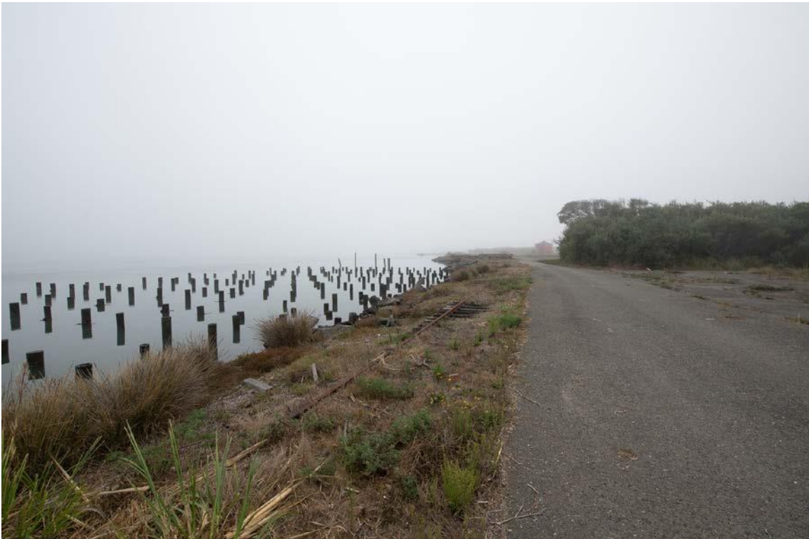
Exhibit I: This is the end of the (approximately MP 300.5) siding.
