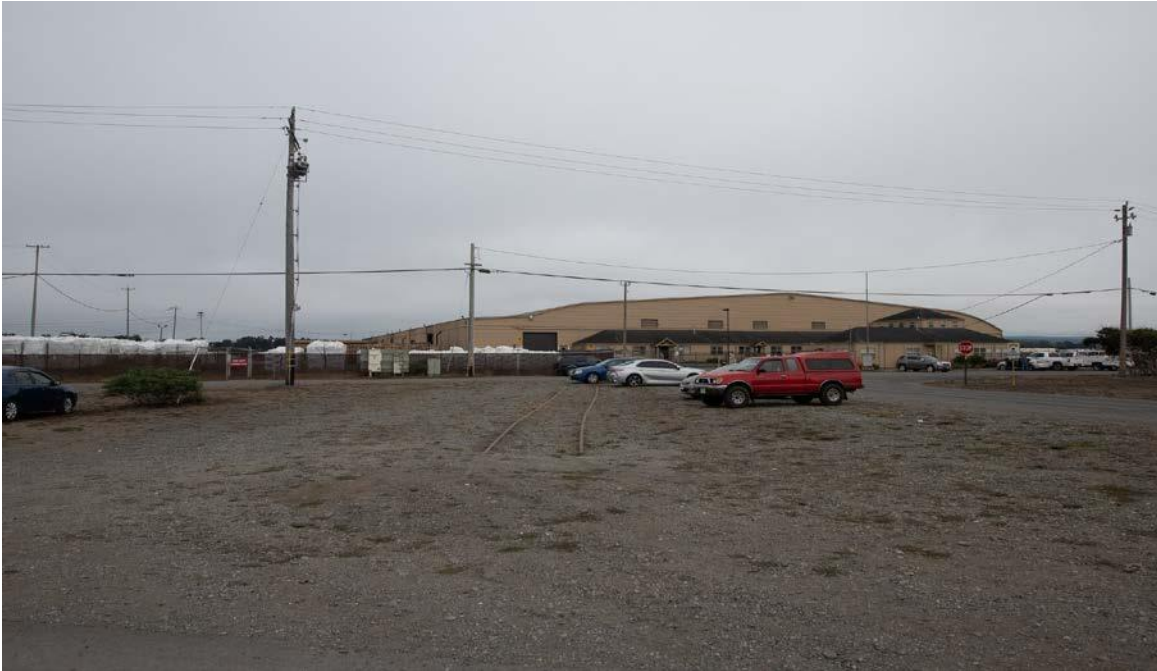
Exhibit L: This is the end-of-track point at approximately milepost 302.86 (?) within the employee parking lot of Fox Farms in Fairhaven, CA.
