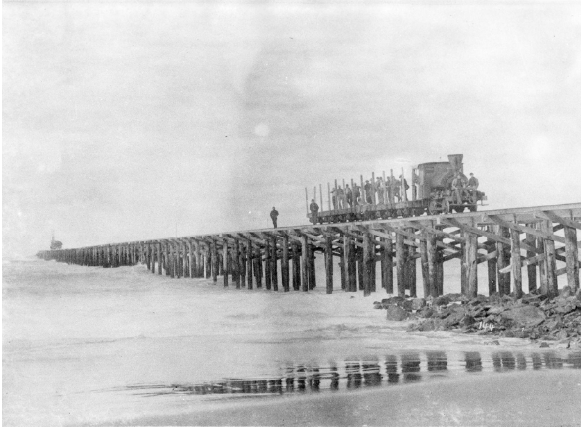
Exhibit C: Construction of the North Jetty, the railroad was extended beyond the termination point of the Samoa Branch to bring supplies to the North Jetty. Humboldt State University Special Collections Photo.
