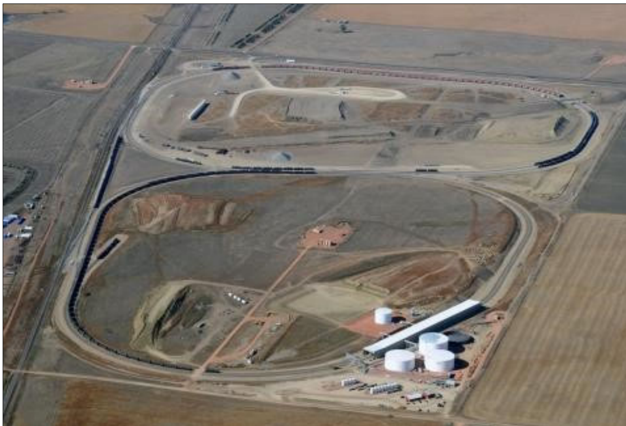
Figure 9-1 Example Crude Oil Rail Loading Terminal
