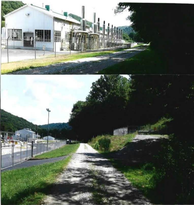
Exhibit C3 Overview of Gas Plant & ROW road Pipeline installation on upper right is part of plant. RR access road runs through center
