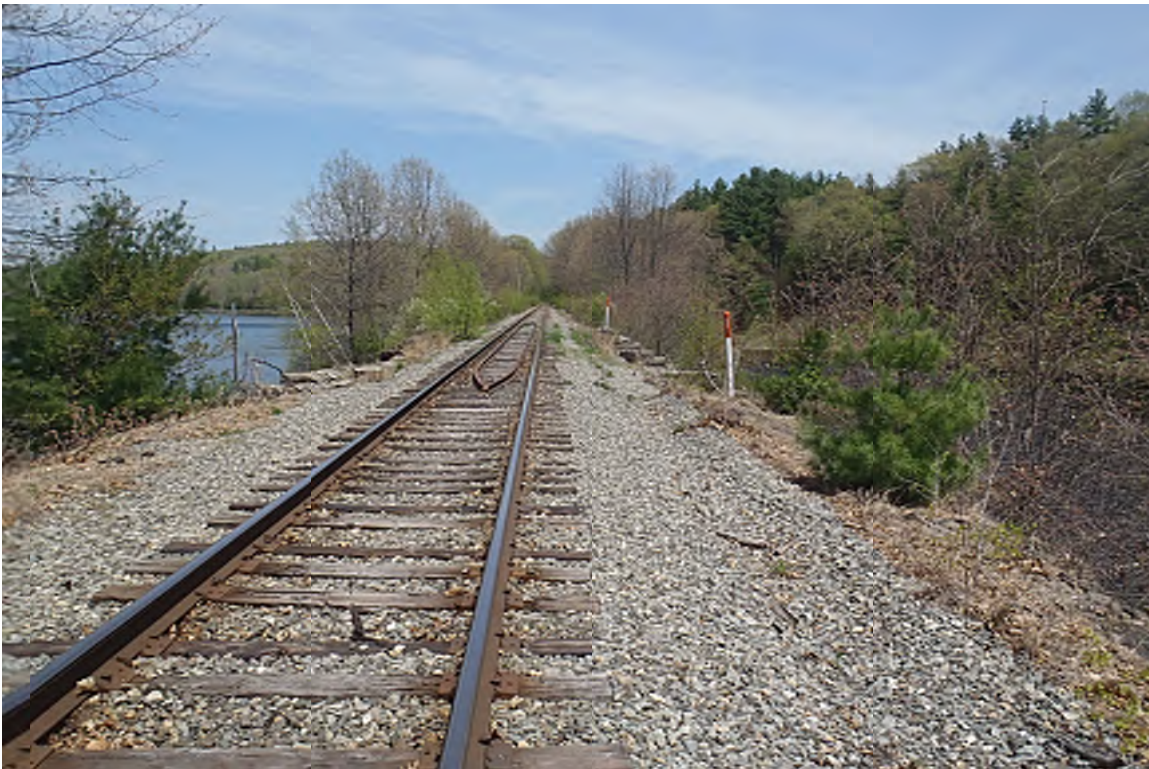
TRACK AT STONE ARCH BRIDGE OVER THE STILLWATER RIVER
