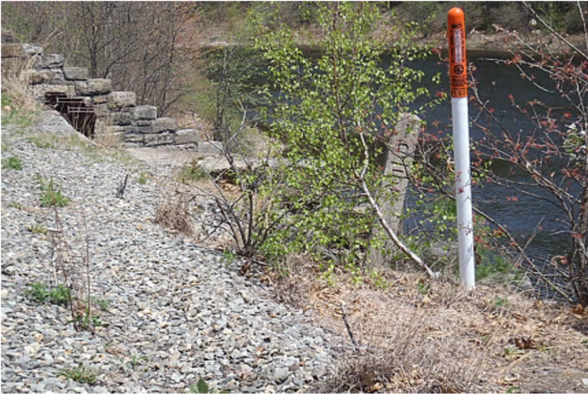
MILEPOST MARKER BY ARCH BRIDGE OVER STILLWATER RIVER
