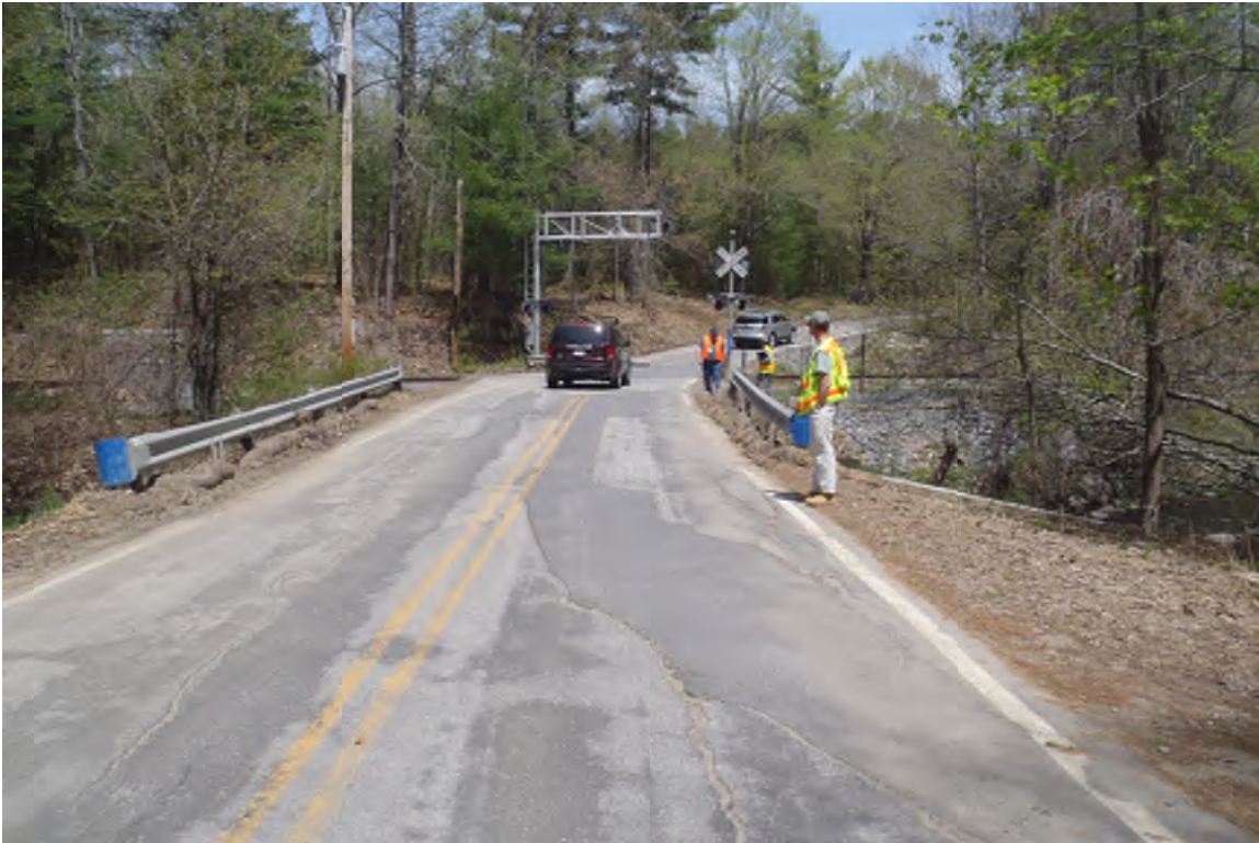
PRESCOTT STREET GRADE CROSSING- NORTHBOUND ROADWAY APPROACH
