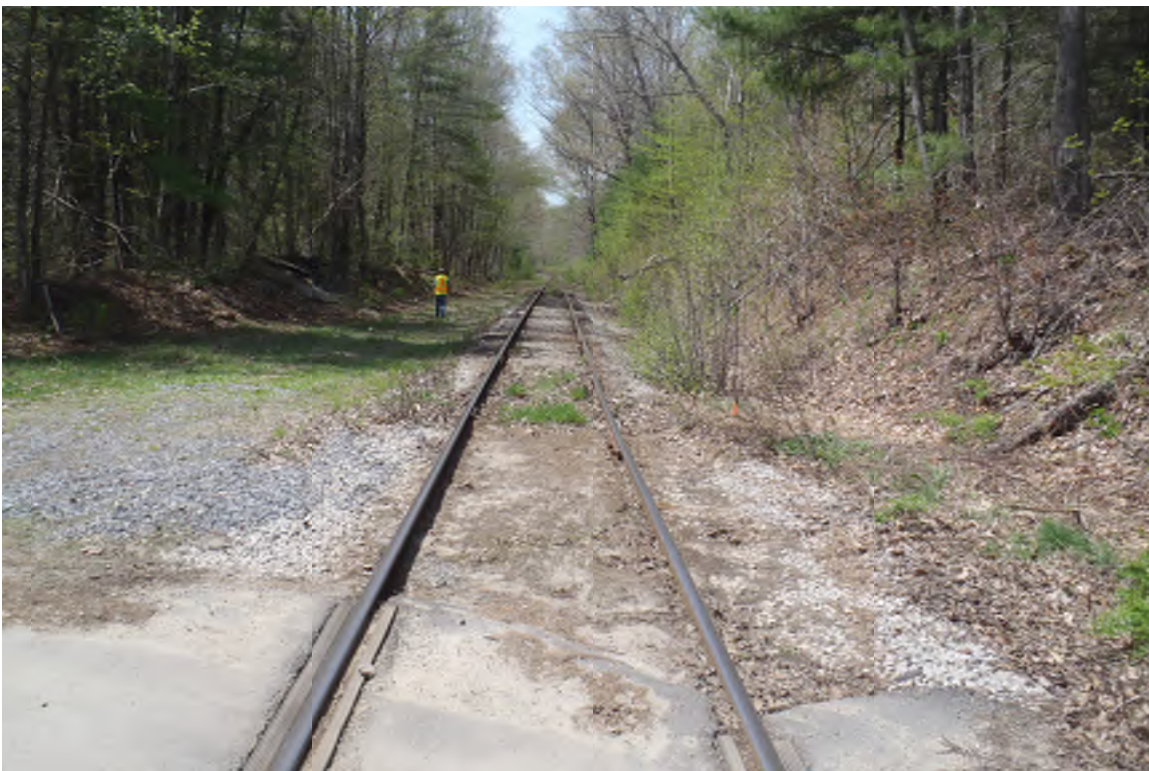
PRESCOTT STREET GRADE CROSSING- THE EASTBOUND APPROACH
