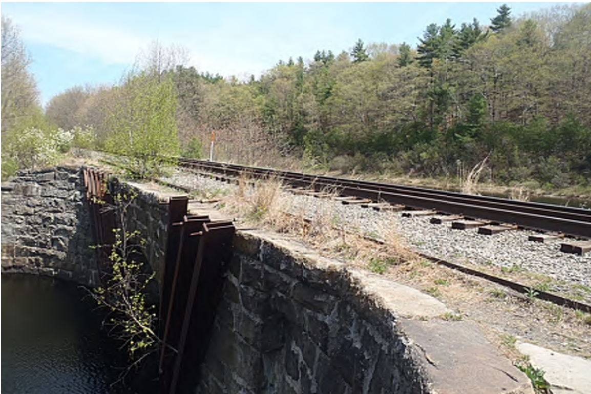
STONE ARCH BRIDGE OVER THE STILLWATER RIVER
