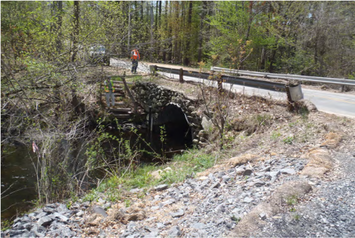
PRESCOTT STREET GRADE CROSSING- CMP ARCH OVER THE WAUSHACUM BROOK
