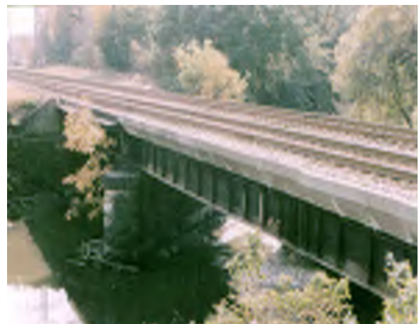
Figure 8-8 Ballast Decked Structure - Courtesy of Metra
