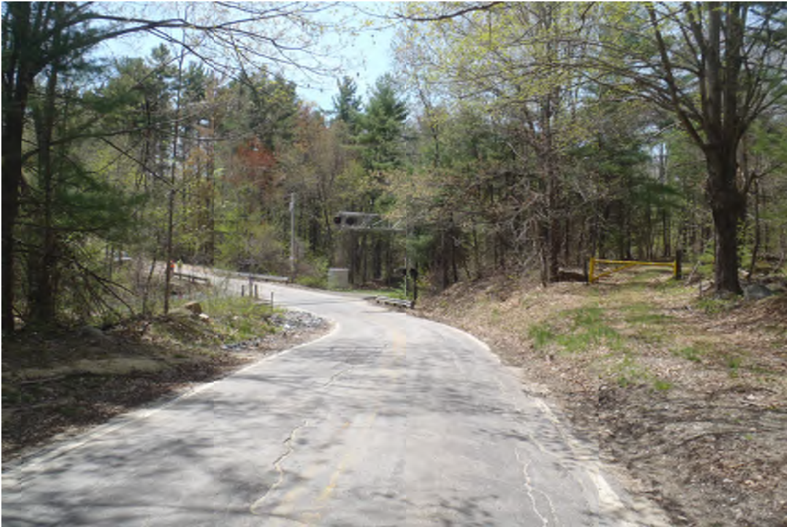
PRESCOTT STREET GRADE CROSSING-SOUTHBOUND ROADWAY APPROACH
