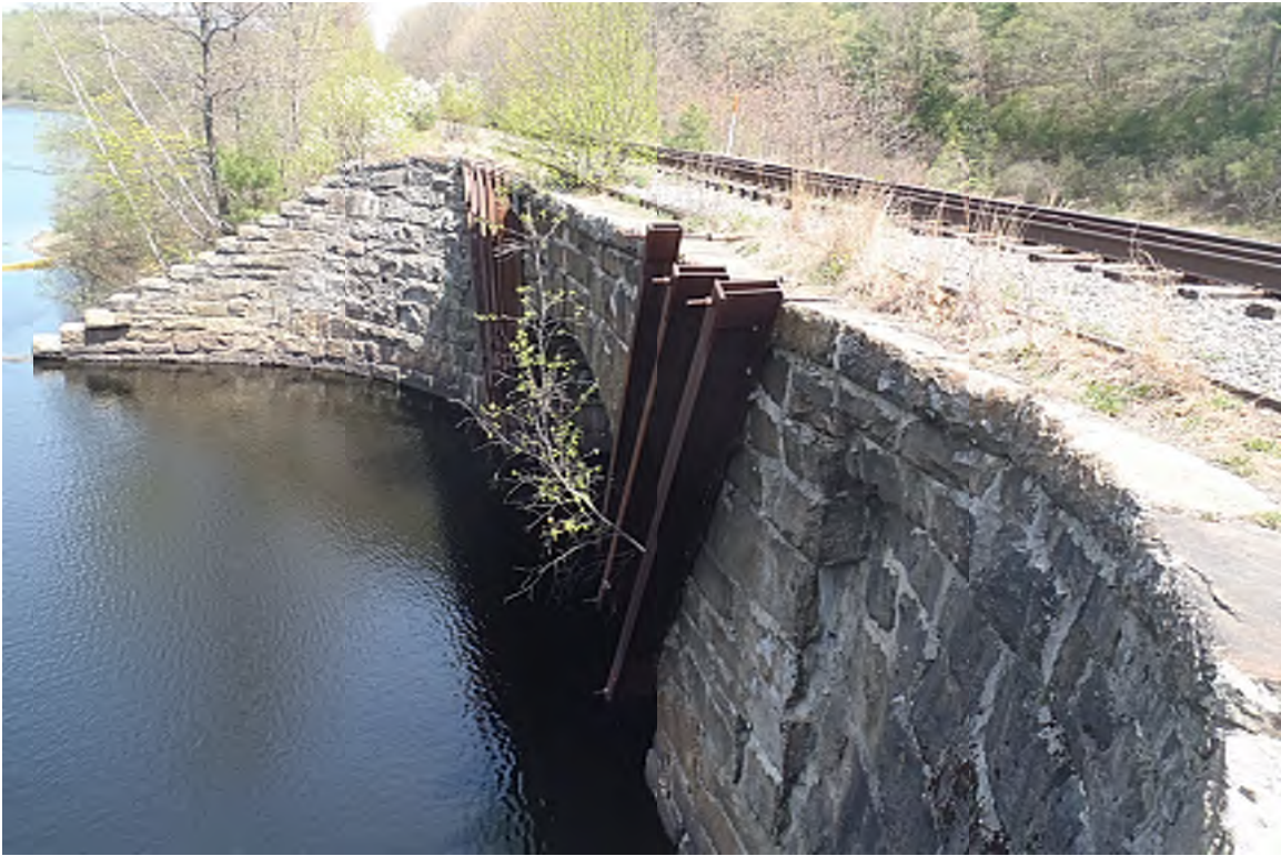
STONE ARCH BRIDGE OVER THE STILLWATER RIVER
