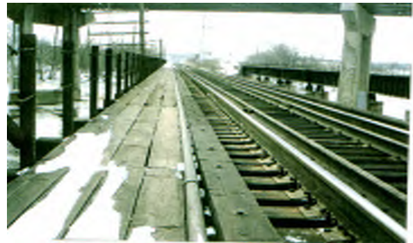
Figure 8-6 Open Deck Bridge - Courtesy of Metra
