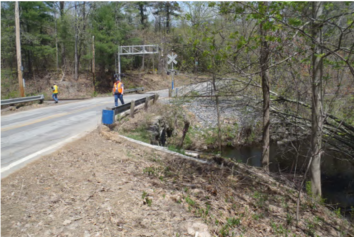
PRESCOTT STREET GRADE CROSSING- NORTHBOUND ROADWAY APPROACH
