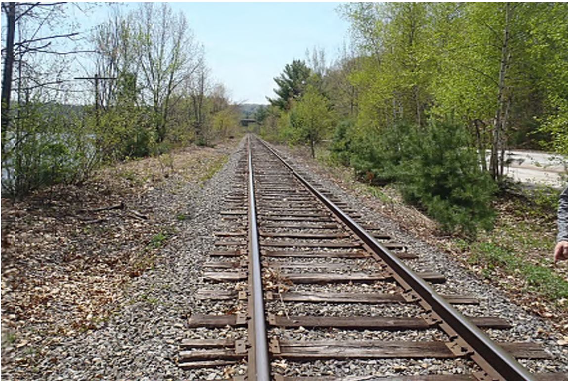
TRACK SECTION BY MP 10.25 +/-
