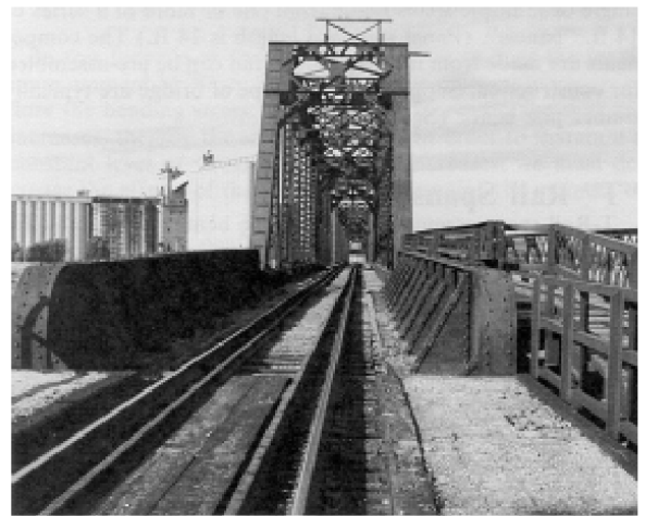
Figure 8-10 Inside Tee Guard Rails - Courtesy of BNSF
