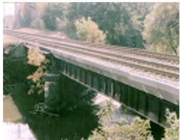
Figure 8-8 Ballast Decked Structure - Courtesy of Metra
