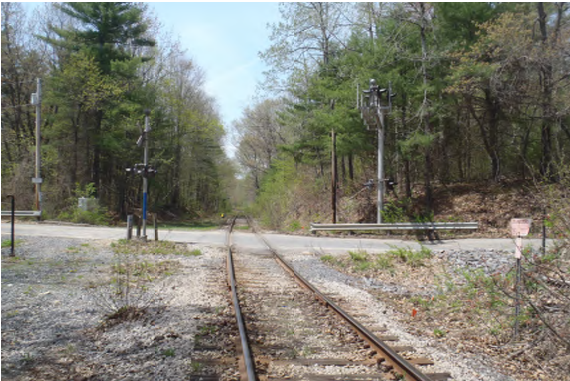
PRESCOTT STREET GRADE CROSSING- LOOKING WEST FROM EASTBOUNDBND APPROACH
