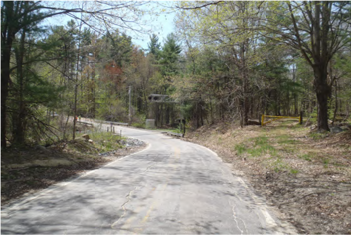
PRESCOTT STREET GRADE CROSSING-SOUTHBOUND ROADWAY APPROACH
