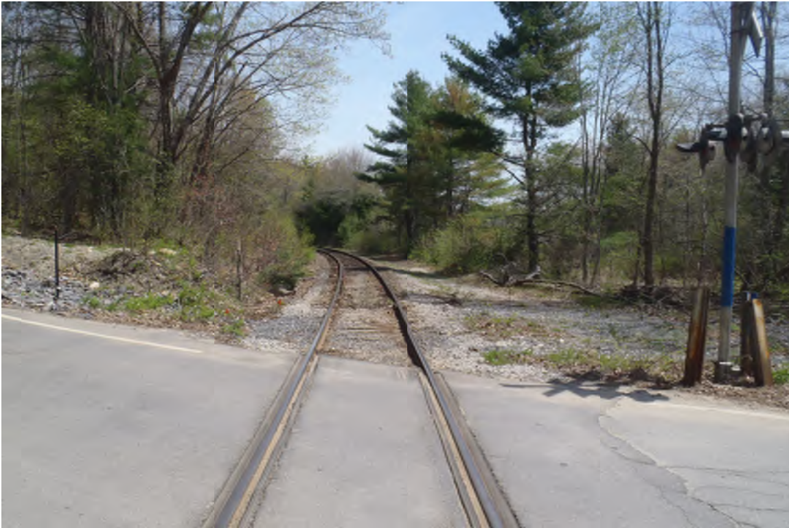
PRESCOTT STREET GRADE CROSSING- THE WESTBOUND APPROACH
