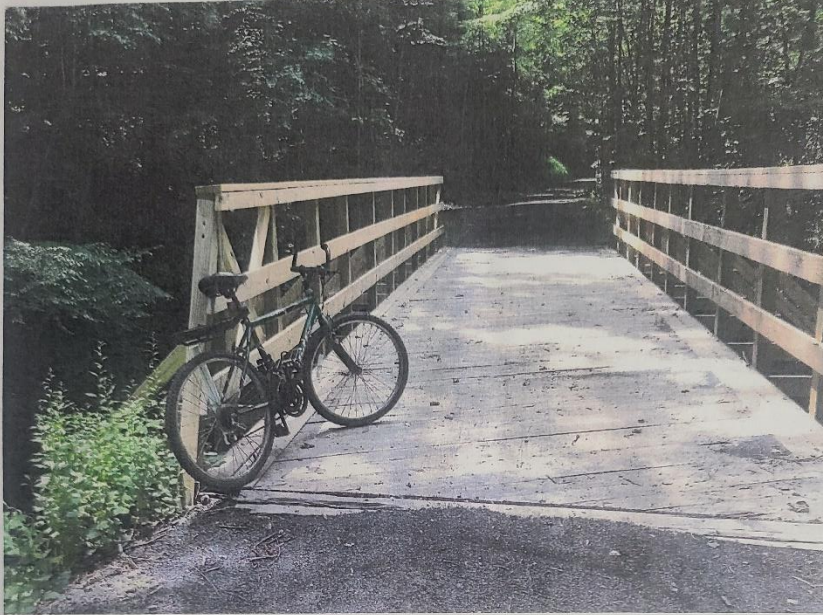
The first of four newly-constructed bridges on the section of the Elk River Trail from Duck to Ivydale.
