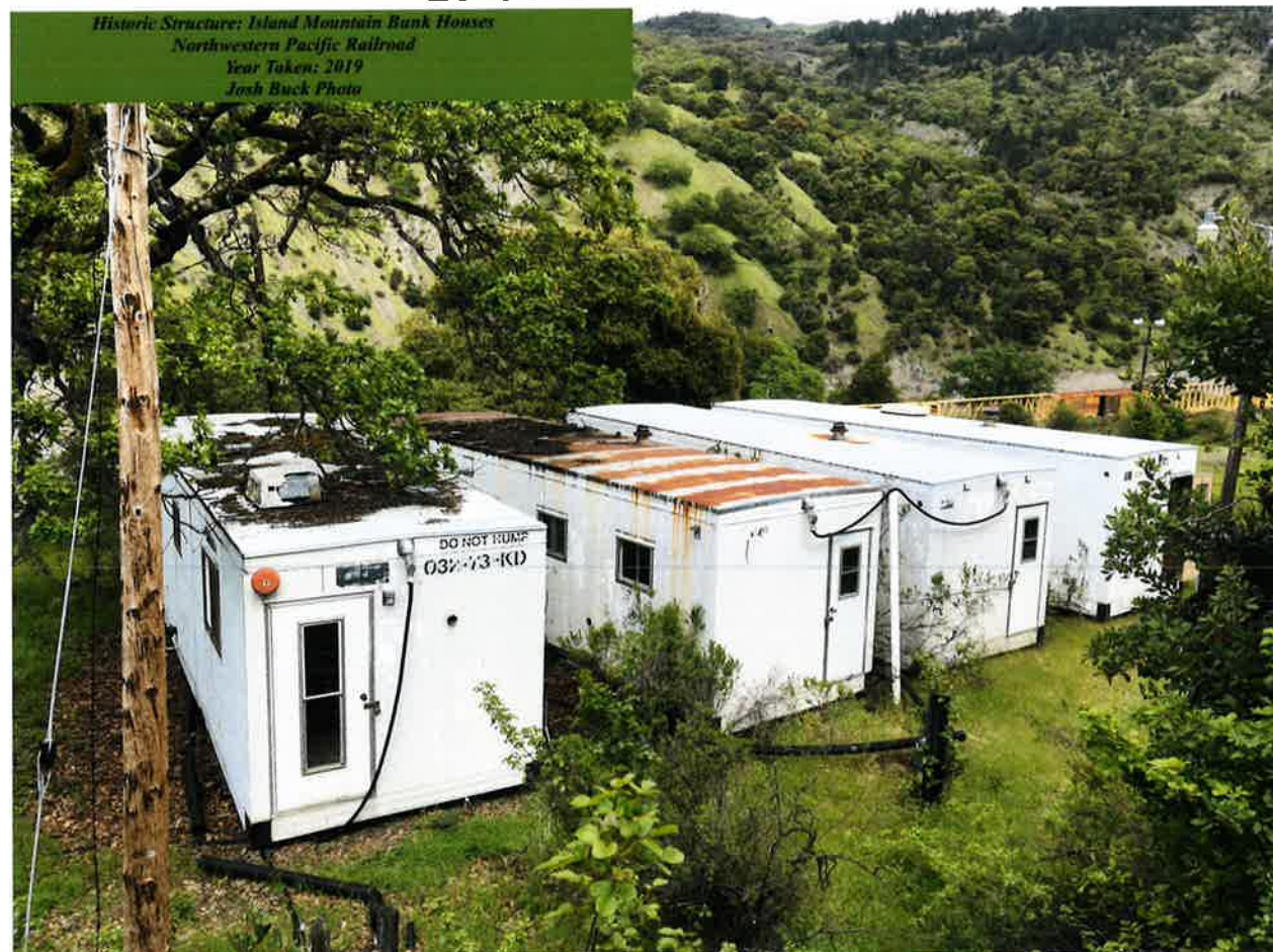
14 Island Mountain Metal Structures
