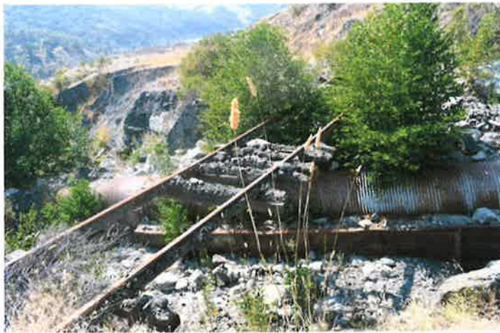
Fig. 16. Current (August 2020) condition of Abbott Creek crossing, at north edge of MP 201 mud glacier. Track is buried from the south end of the crossing over the entire slide zone. The track rests on a pipe installed in an unsuccessful effort to drain the glacier. The pipe rests on an old NWP gondola car. Photo by J. Buck, Aug. 2020
