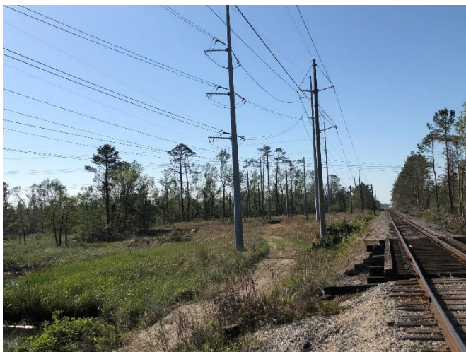
LOOKING SOUTHWEST ALONG LINE AT WATER CROSSING
