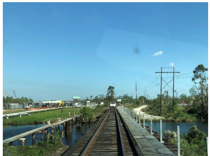
VIEW OF BRIDGE (LIMITED UTILITY AREA)
