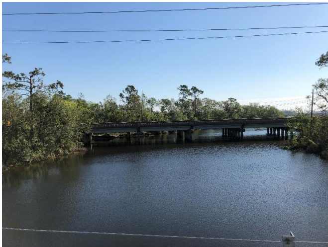
VIEW OF WATER CROSSING
