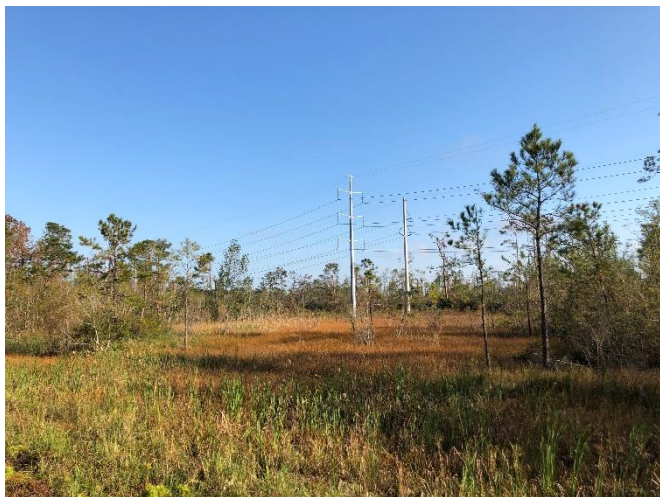
VIEW OF TYPICAL ADJACENT PROPERTY
