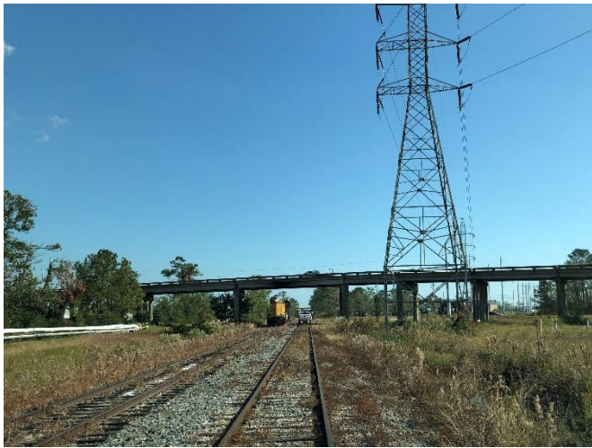
LOOKING NORTHEAST ALONG LINE TOWARD PRATER RD BRIDGE CROSSING
