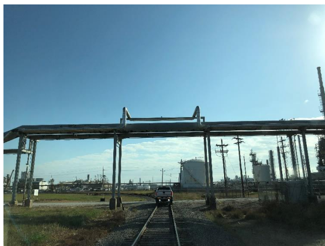
VIEW OF ABOVE GRADE PIPELINE CROSSING
