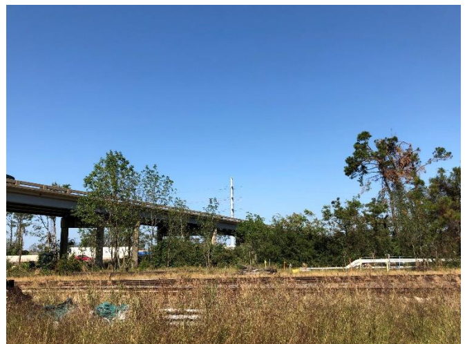
LOOKING NORTH TOWARD IH 210 BRIDGE CROSSING
