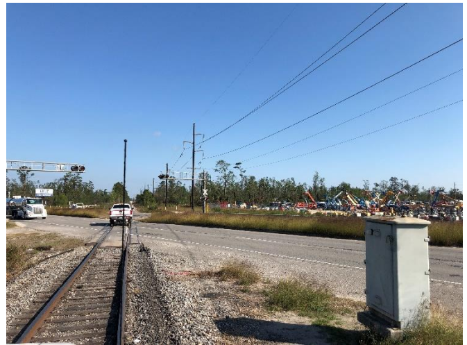
LOOKING NORTHEAST AT SH 108 CROSSING (100' WIDTH SEGMENT)
