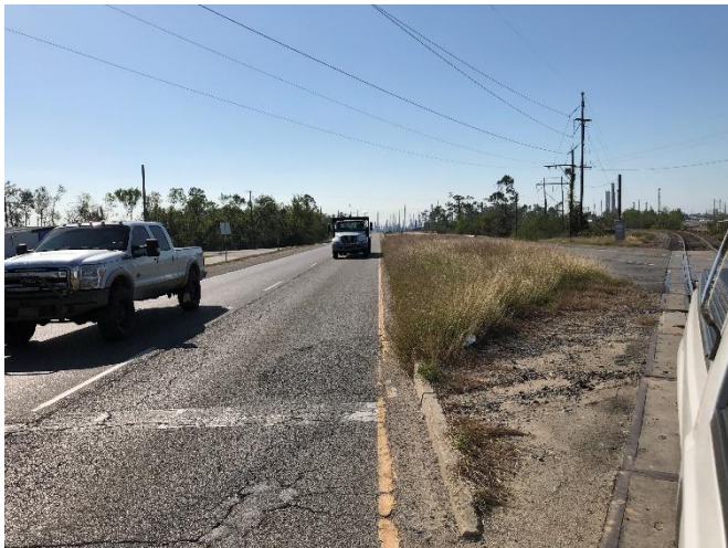
LOOKING SOUTH ALONG SH 108 FROM CROSSING
