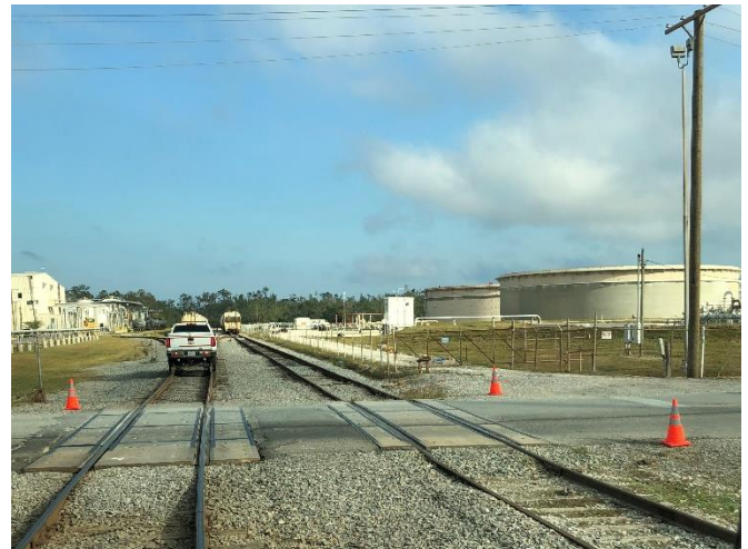
VIEW OF DAVISON ROAD CROSSING
