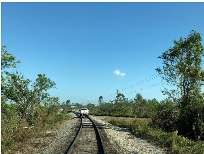
LOOKING NORTHEAST ALONG LINE (1960 SPUR ON RIGHT)
