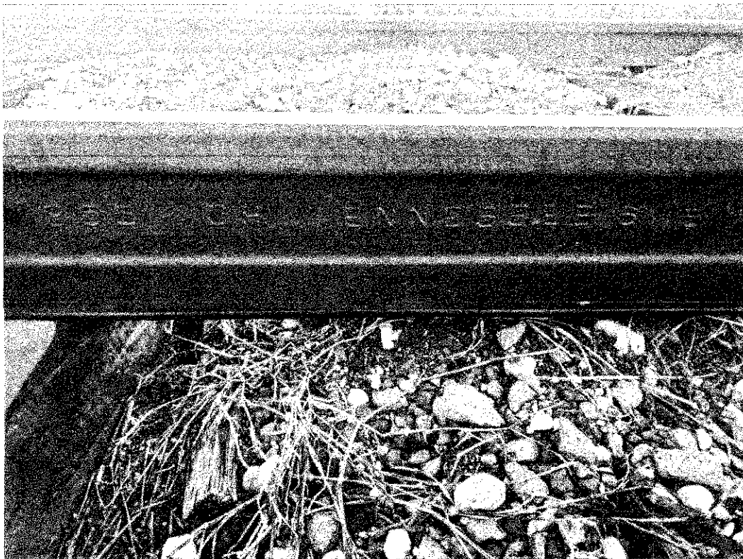
Figure 4, rail branding: 855 OH TENNESSEE.
