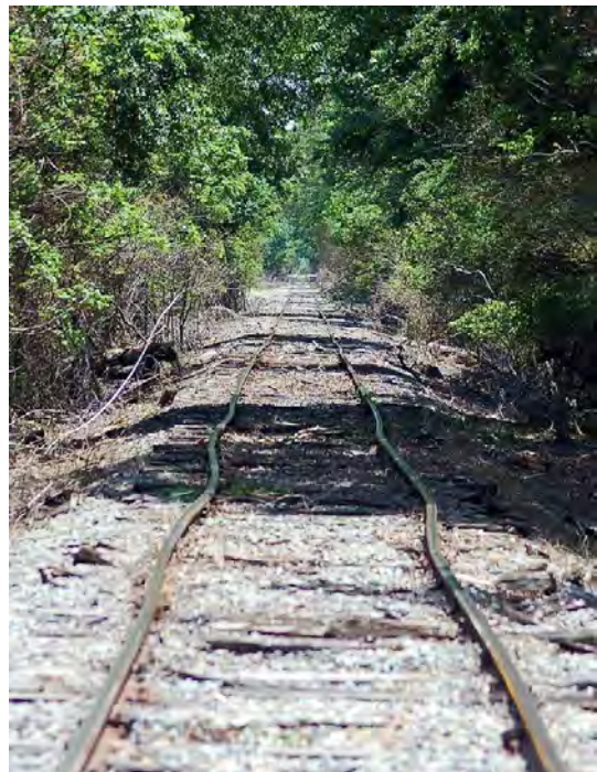
Figure 2: McGehee-Tallulah Railroad Corridor Existing Track Conditions
