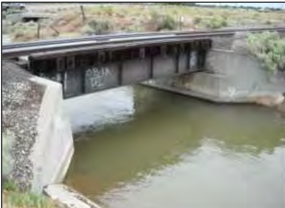
Irrigation Canal Bridge
