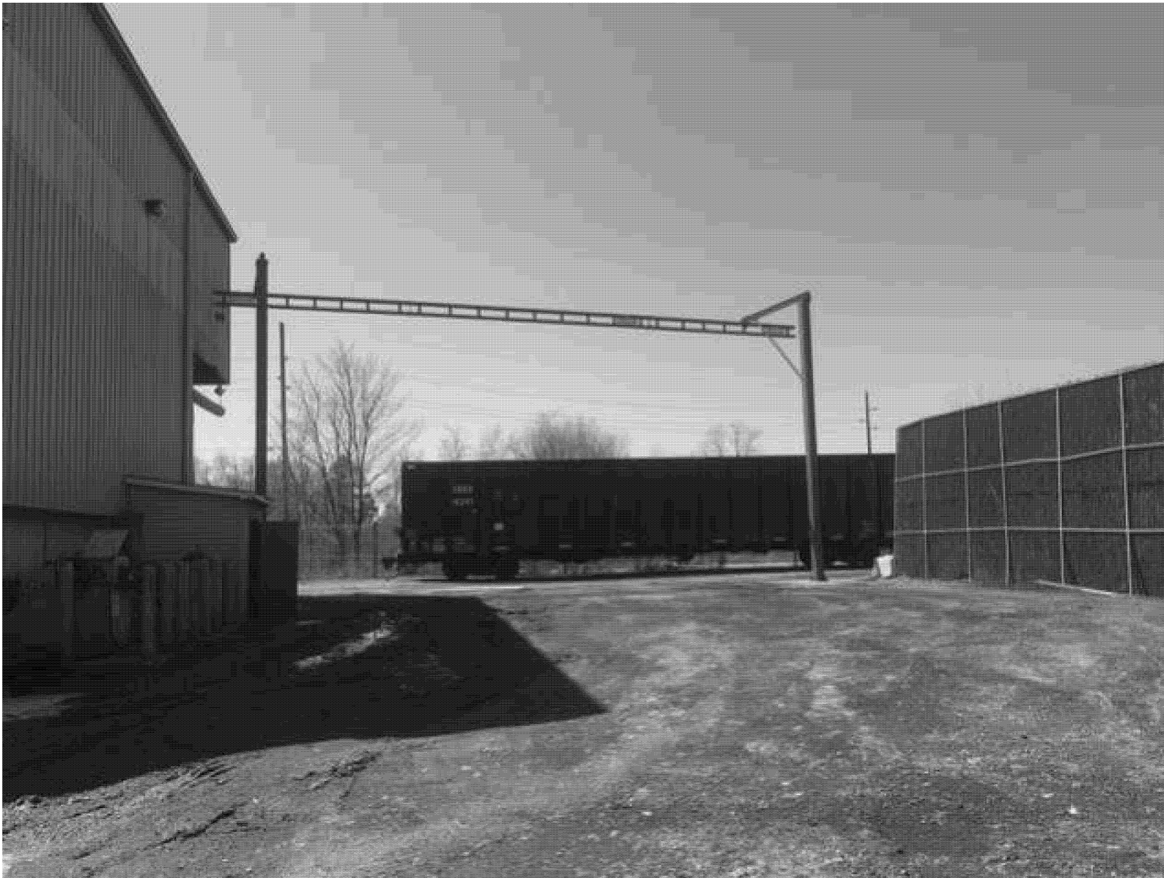
TYPICAL TARPING OPERTIONS
