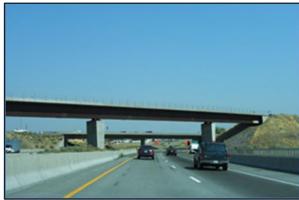
Berry's Overpass Bridge
