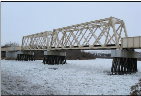
Yakima River Bridge
