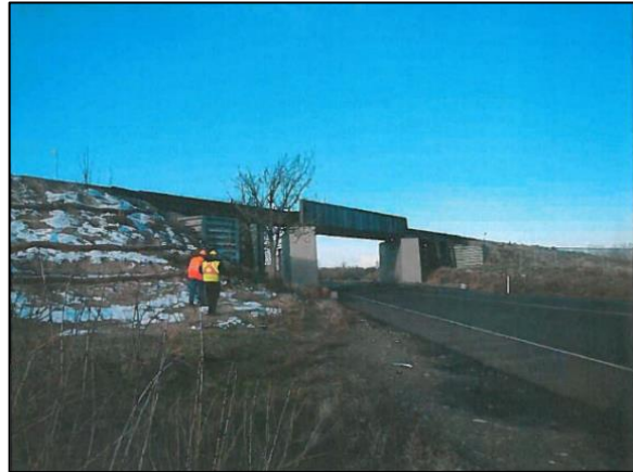
Columbia Park Trail Bridge
