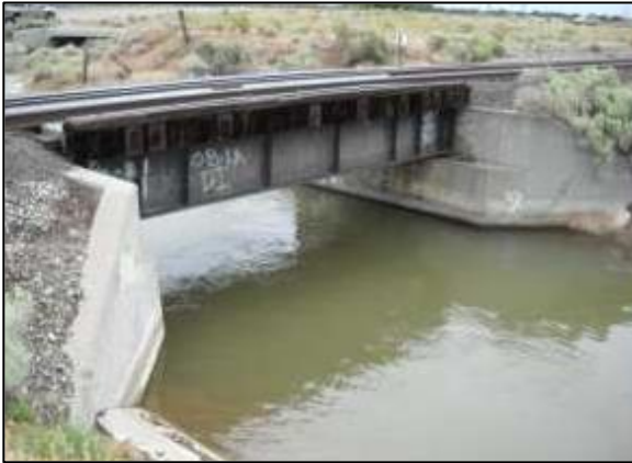
Irrigation Canal Bridge
