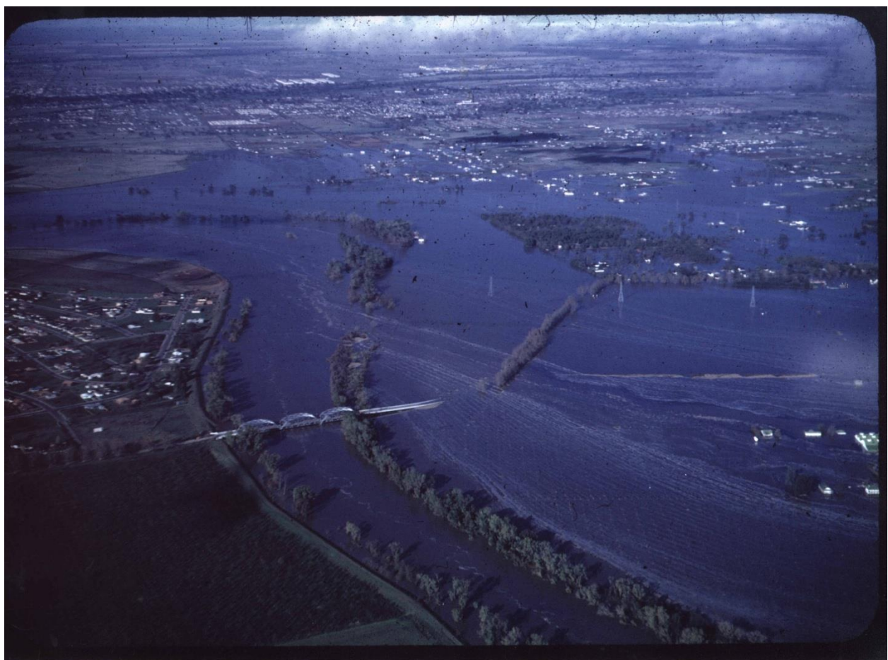
Figure 2.12. 1950 Flood – H Street Bridge
