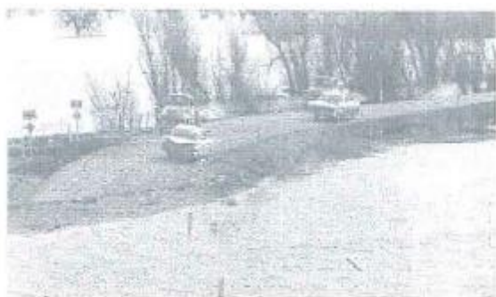
Figure 2.14. Flooding on Franklin Boulevard in 1964
