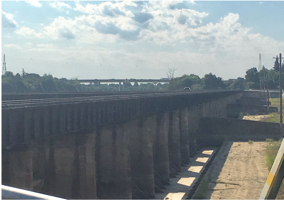
Photograph 3: Timber Rail Trestle adjacent to weir (camera facing south)
