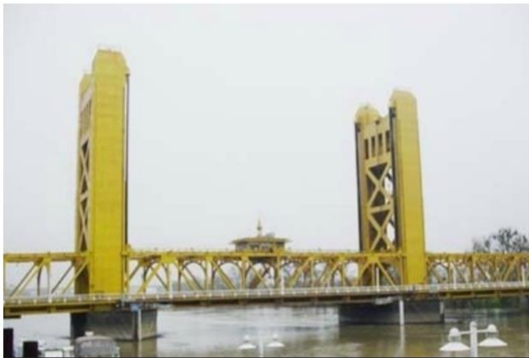
Figure 2.18. Tower Bridge – Jan 2003
