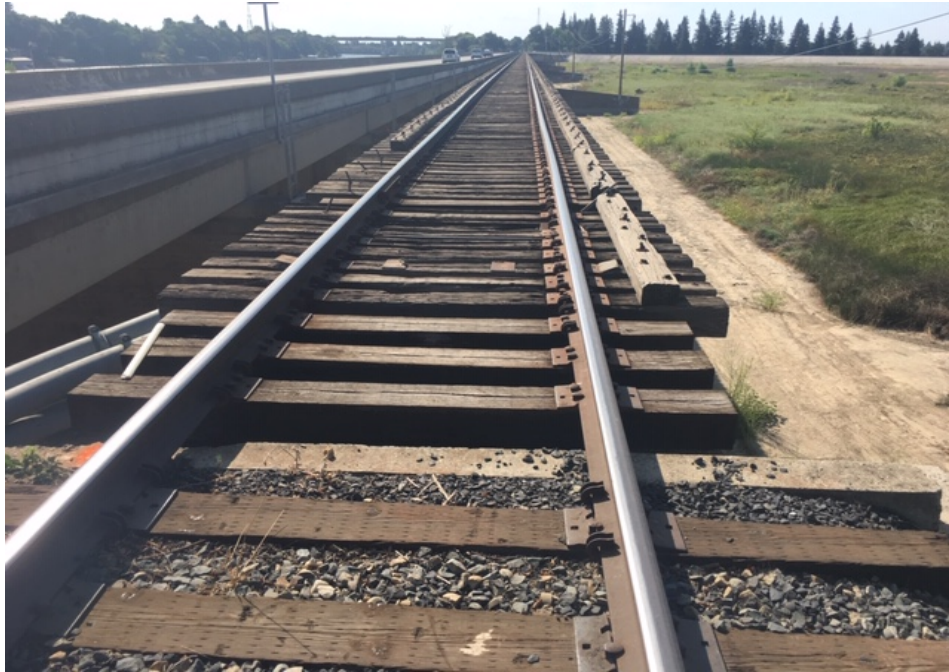
Photograph 2: Alignment Extending Across Sacramento Weir (camera facing south)
