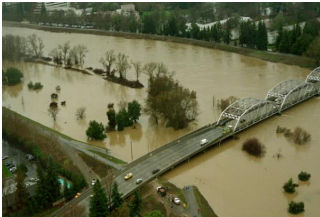
Figure 2.15. 1986 Flood – H Street Bridge
