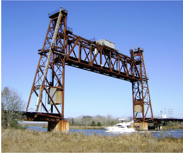
Figure 5. Cedar Bayou Bridge, Looking Southwest
