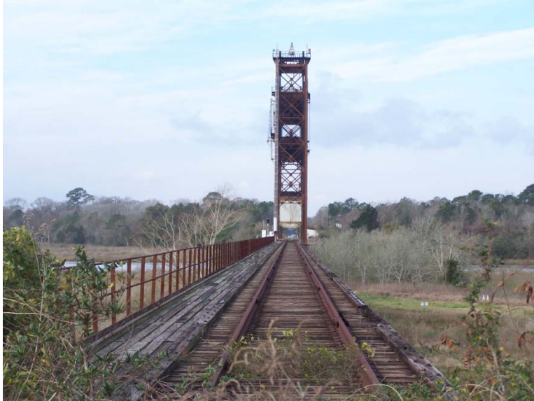
Figure 7. View of Girder Spans and Lift Tower, Looking West
