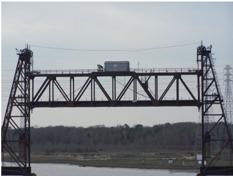
Figure 4. Cedar Bayou Bridge, Looking South
