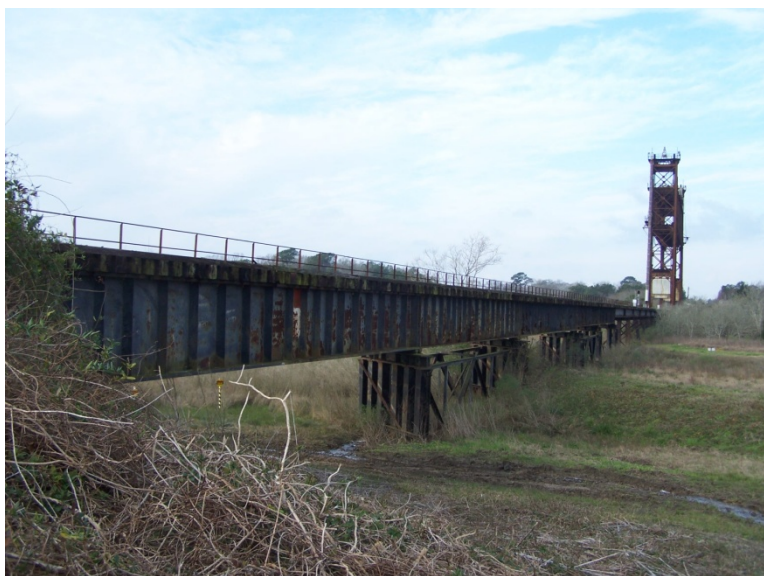
Figure 6. View of Girder Spans and Lift Tower, Looking Southwest
