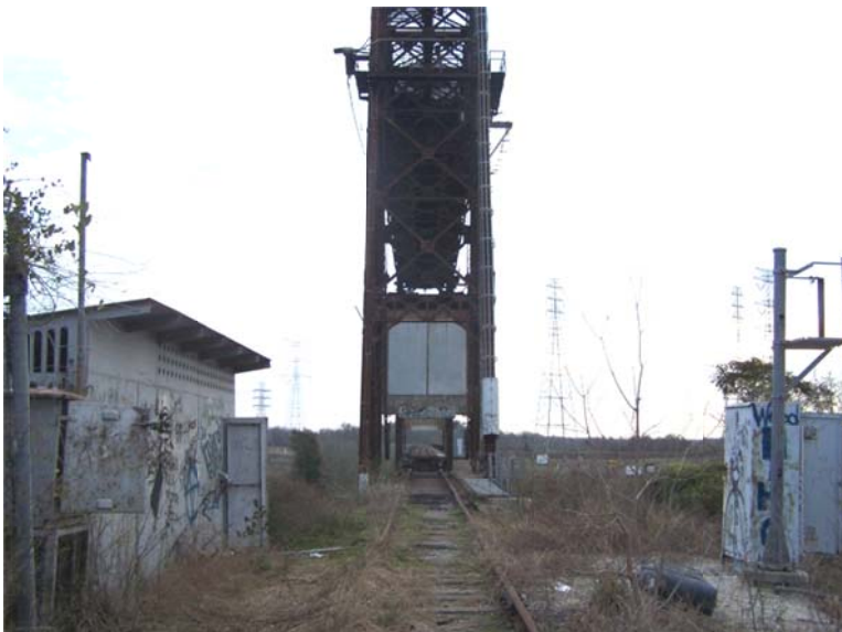
Figure 8. View of Deck and Lift Tower, Looking East
