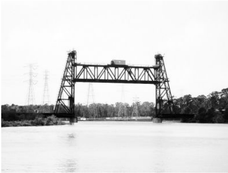
Figure 3. Cedar Bayou Bridge, Looking South
